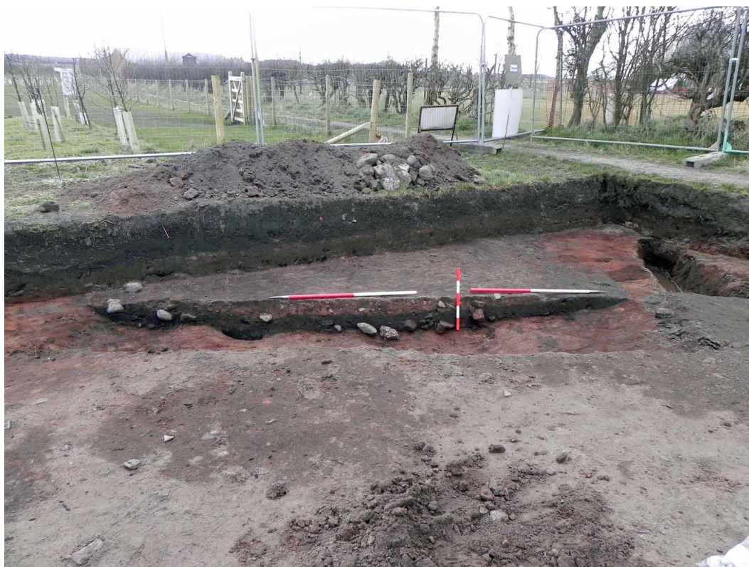
Plate 8. Section across the western end of the east-west aligned trackway. View looking north-west.
