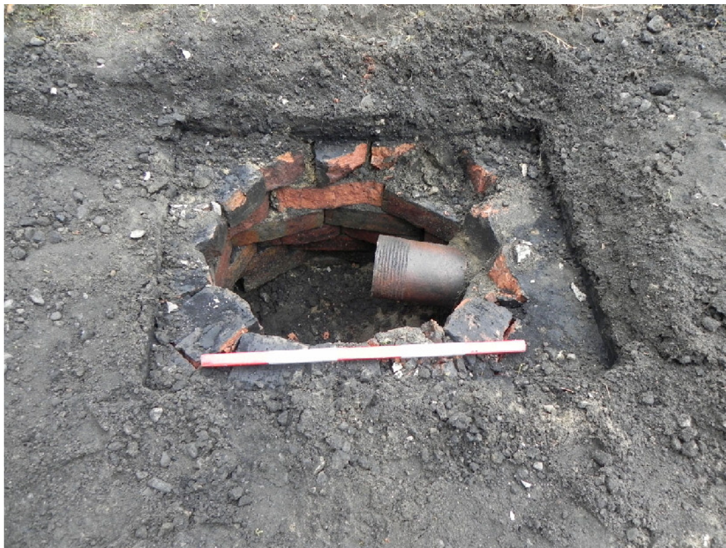
Plate 8. Brick lined soakaway in Trench VIII
