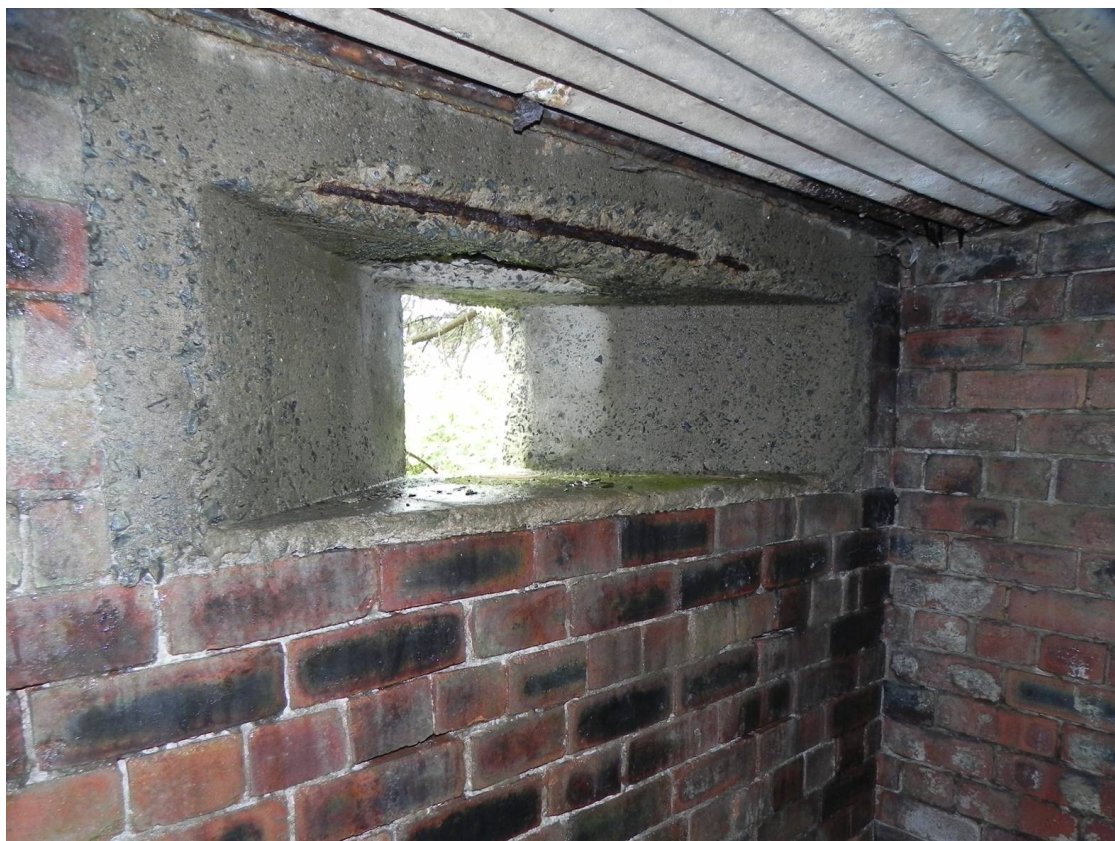
Plate 15. Structure 4, internal view of eastern gun slit.
