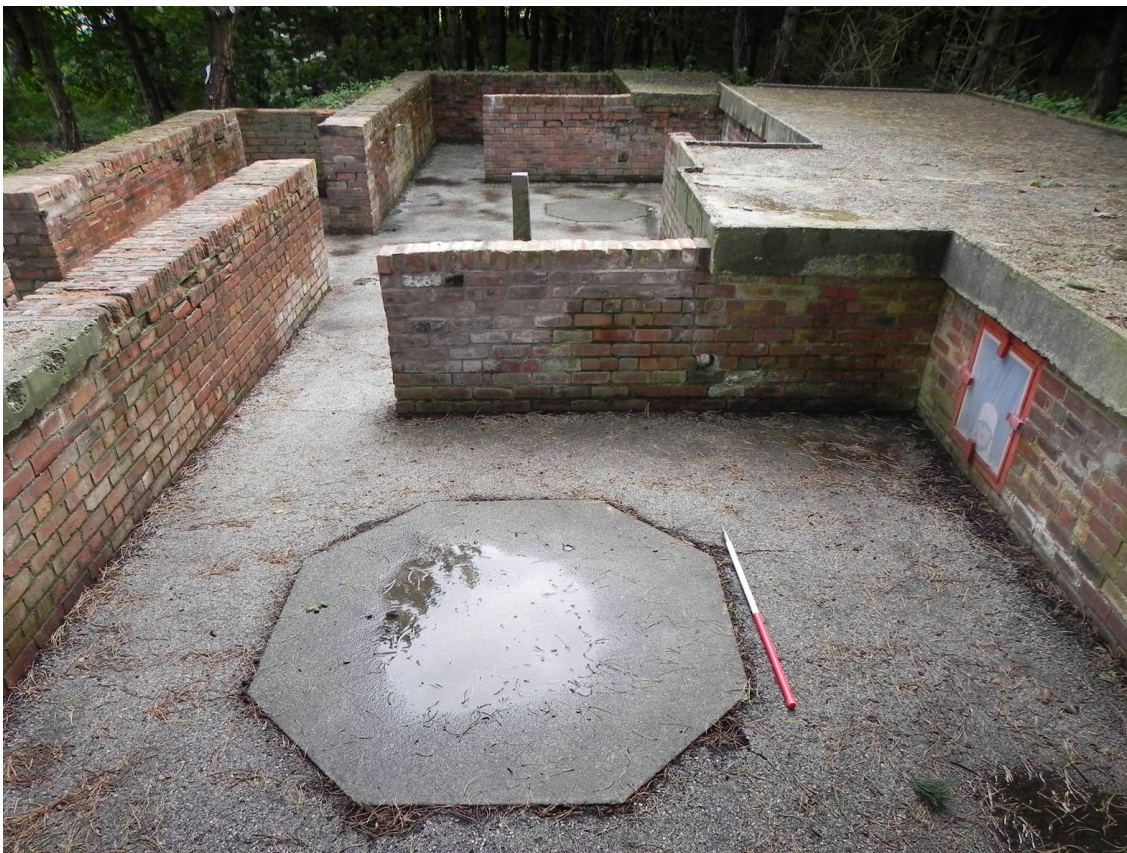
Plate 4. Structure 1, northern courtyard view from the north.
