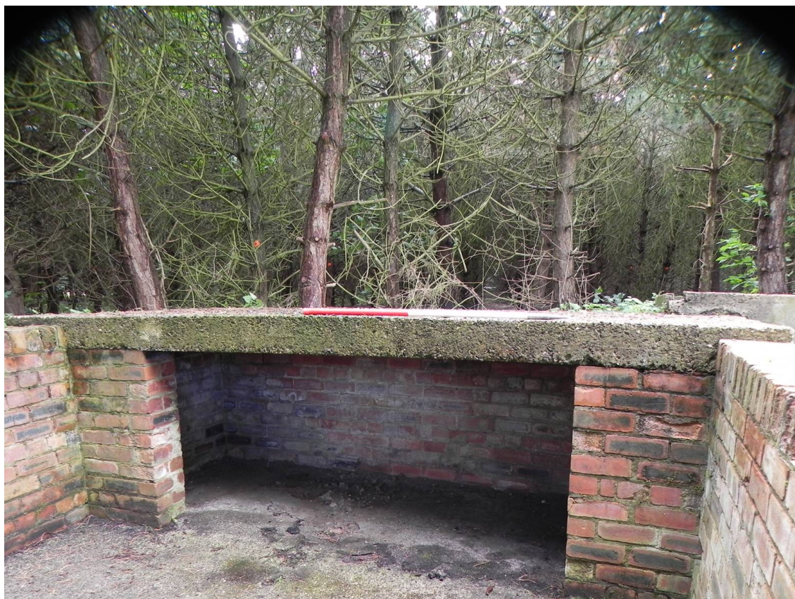
Plate 5. Structure 1, southern courtyard, storage bunker from the east.
