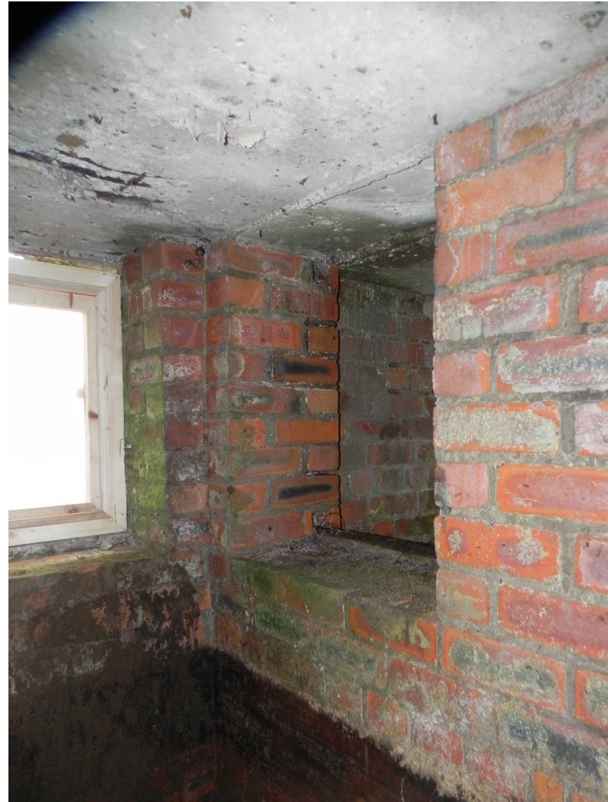
Plate 8. Structure 1, Room 2, window giving view of stairs (right).
