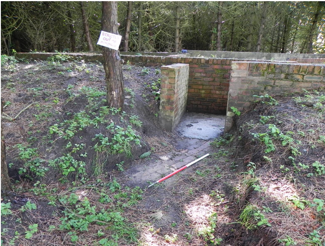
Plate 3. Structure 1, path leading from eastern entrance.
