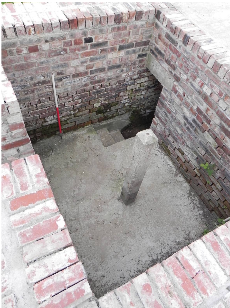
Plate 14. Structure 2. View looking north-west into the entrance.
