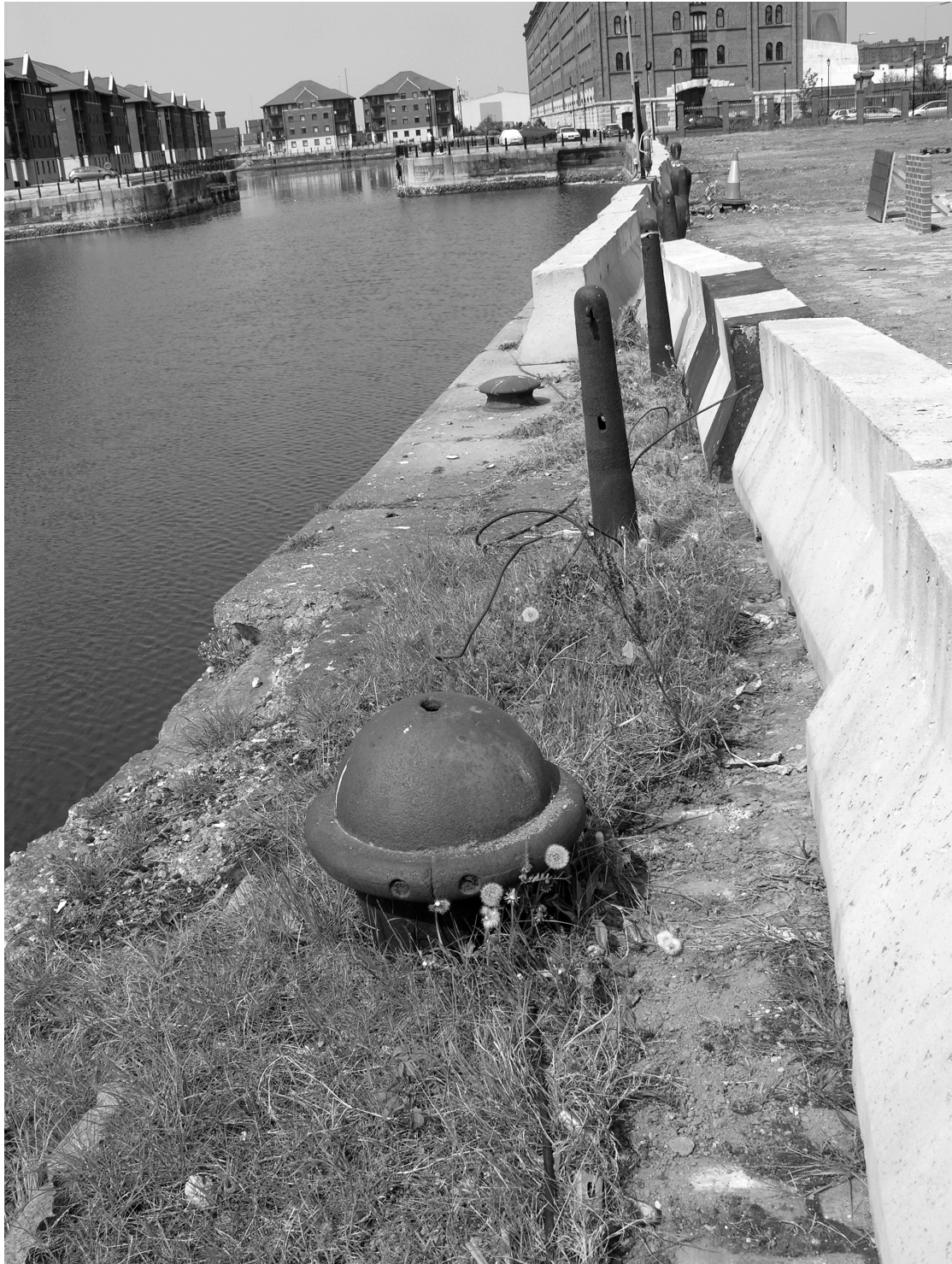
Plate 7. Bollard, NWSIAH (1981-2) modified Type B1 in cast iron with iron(?) 'collar fitted to the widest point.
