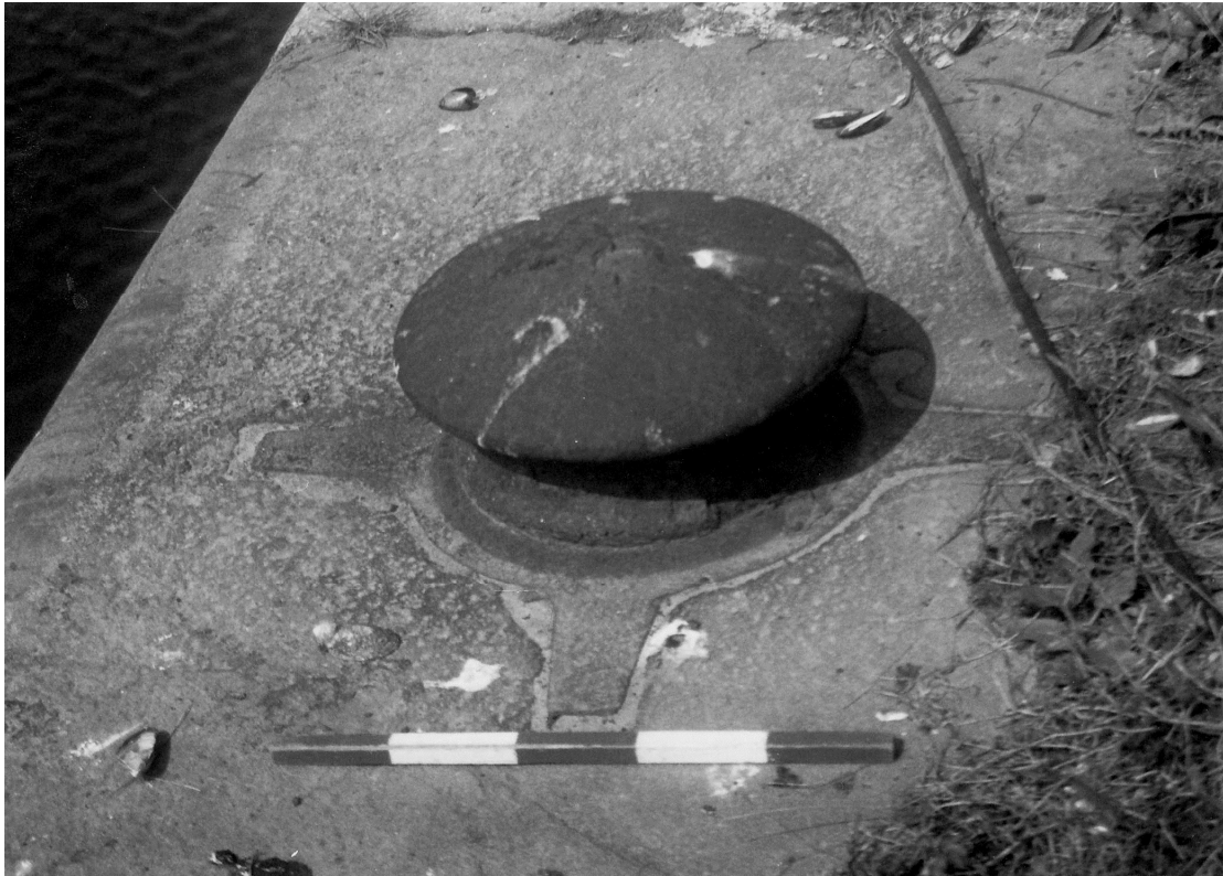
Plate 3. Idler Wheel: Cast iron on a cruciform cast iron base set into granite. NWSIAH (1981-2) Type T1
