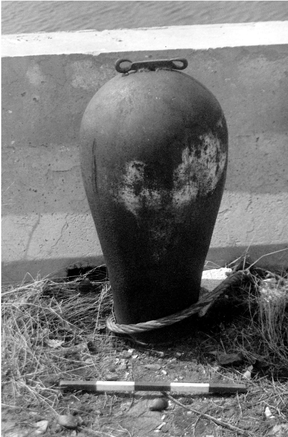
Plate 6. Bollard, NWSIAH (1981-2) modified Type B1 in cast iron with wrought iron bracket welded to the head.
