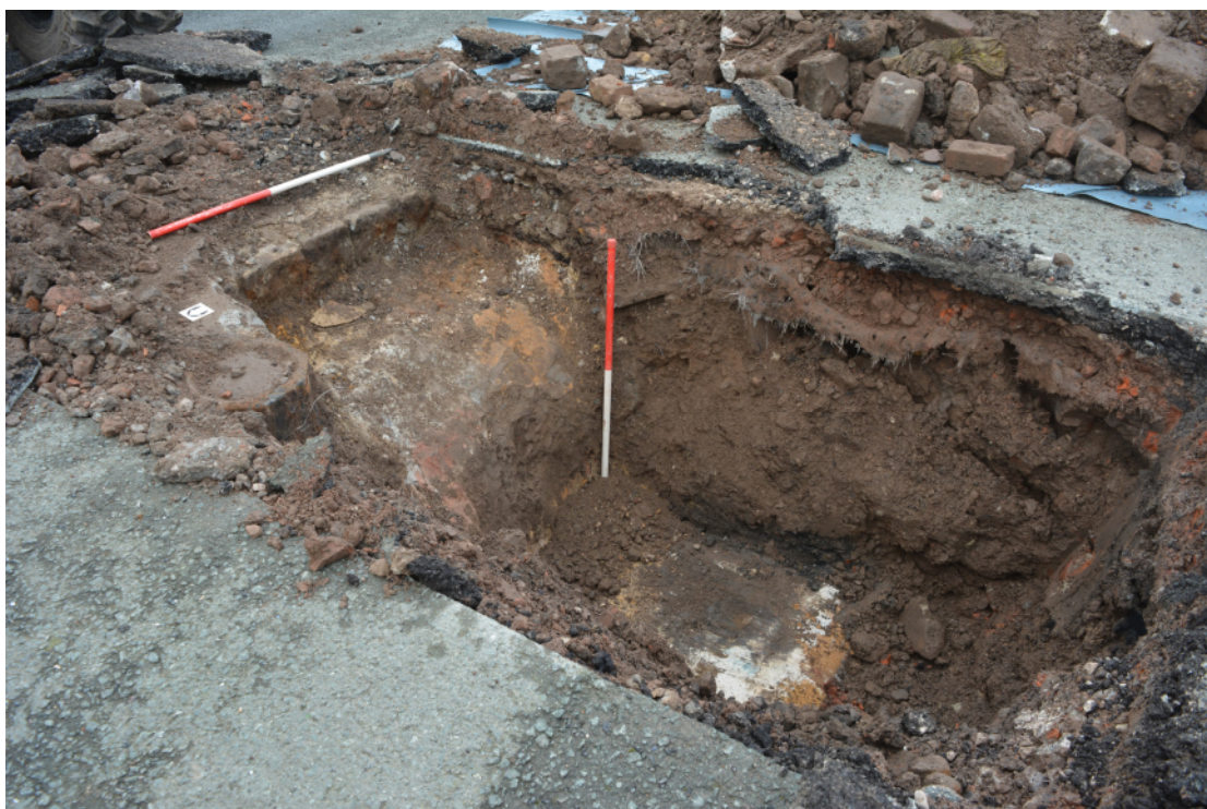
Plate 4. TT302/303. Step cut into upper surface of Princes Dock retaining wall. View looking south-east. Scales = 1m.
