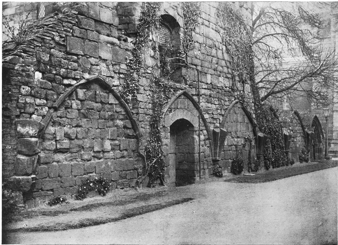
Fig. 4. Corbels and wall-ribs, W. side of Dorter sub-vault ; showing the whole six bays.
