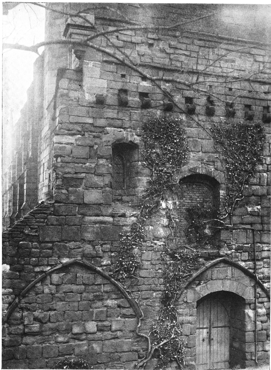
Fig. 9. East wall of Fraternity, showing door to Dorter sub-vault from Slype, and on the first floor the entrance to Dorter from day-stair (now blocked); also window and roof-corbels of Dorter.
