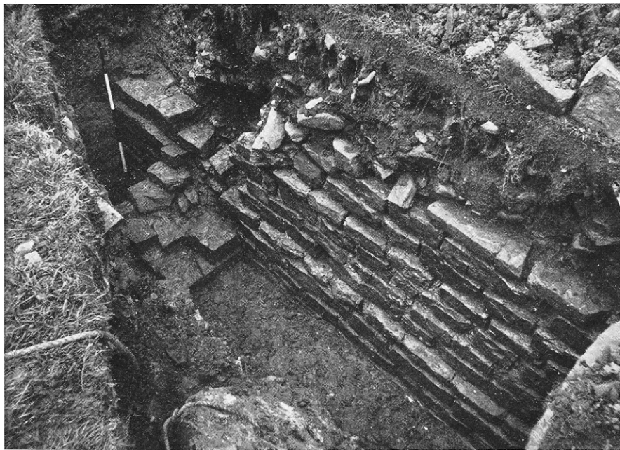
FIG. 5.—Foundation-work of third-century commandant's house, Bewcastle.
