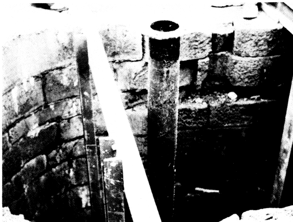
PLATE 1. Top of shaft showing 'waist' and methane pipe (Whitehaven Museum).
