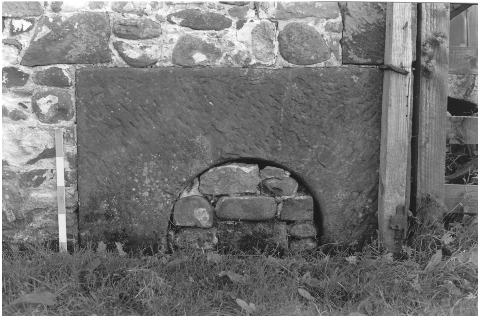
FIG. 1. Roman window head at 'The Drovers Rest', Monkhill, Cumbria. (the scale measures 500 mm). (Photograph: P. Cracknell)
