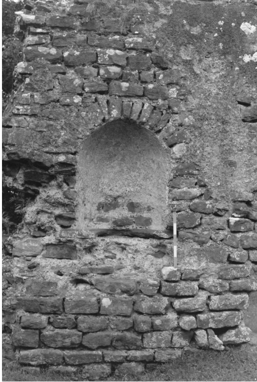
FIG. 3. Wall niche in the bath-house at Ravenglass (the scale measures 500 mm). (Photograph: P. Cracknell)
