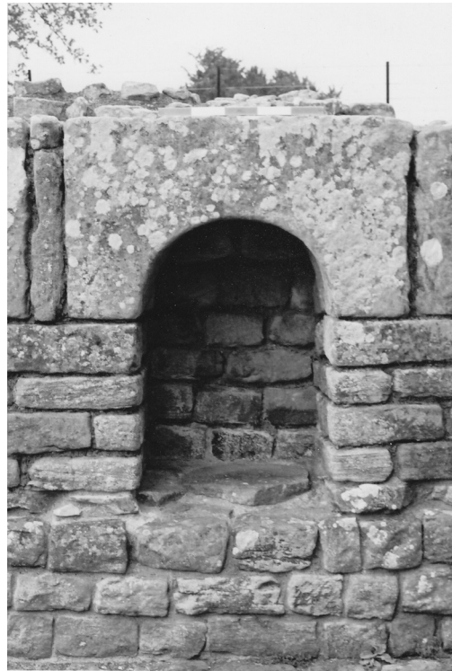
FIG. 2. Niche in the bath-house at Chesters fort (the scale measures 500mm). (Photograph: P. Cracknell)
