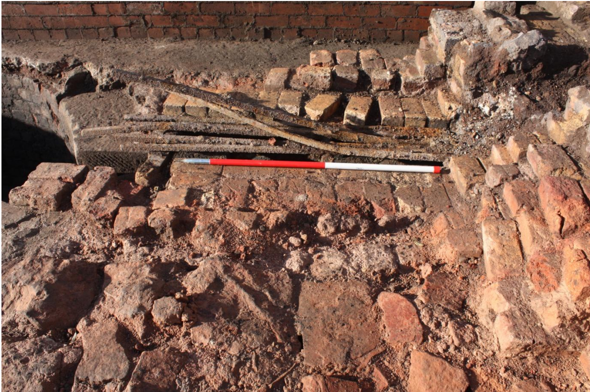
Plate 5: Fire rods in situ in fire trench of the western furnace. Facing west. Scale 1 x 1m.
