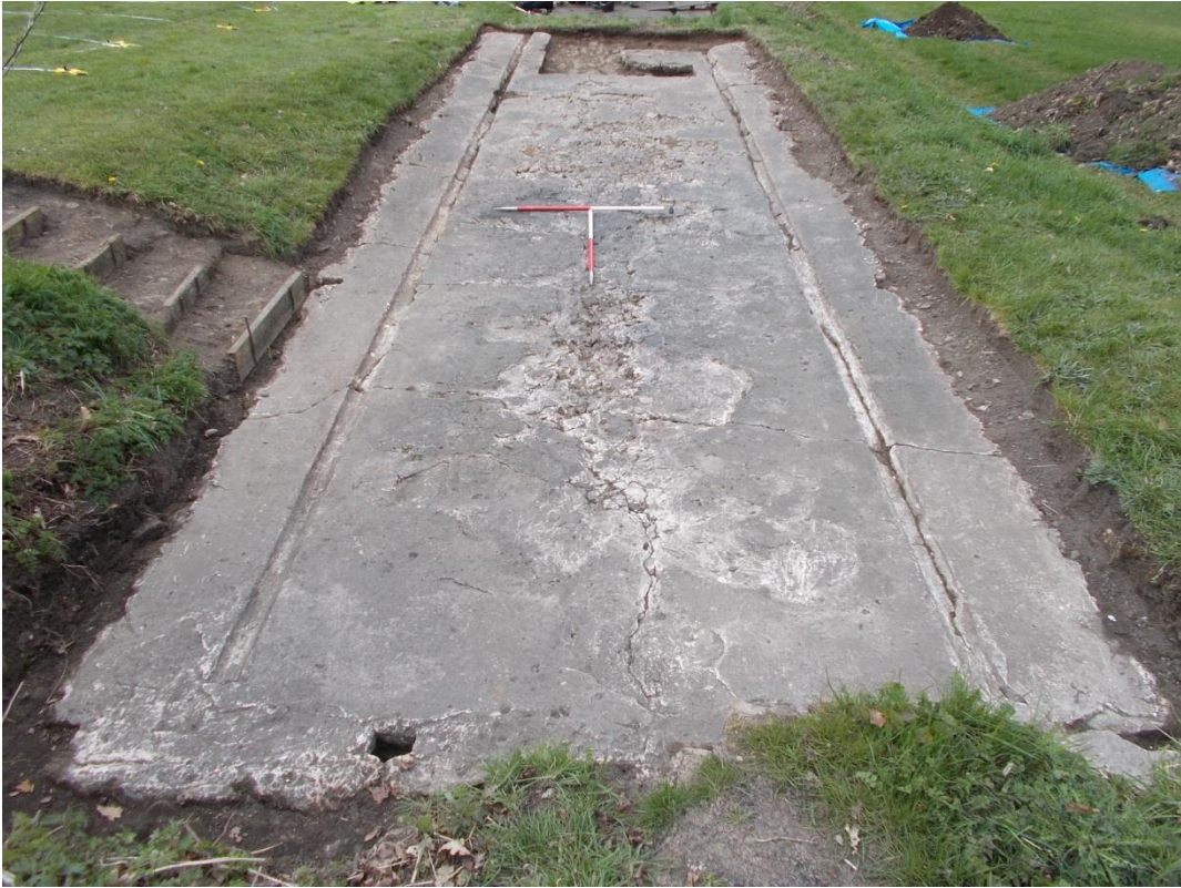
Plate 4: Base 2, detail of north-west end, showing void in concrete, facing north-east. Scales 2 x 1m.
