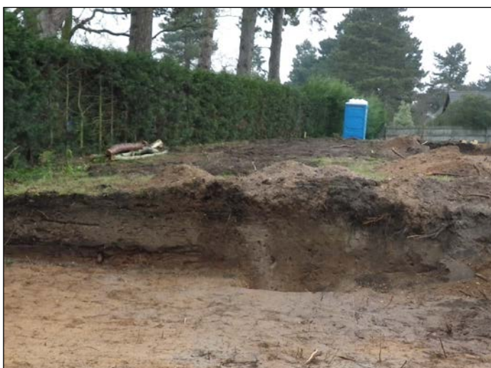
Plate 2. General view of ditch 0032 cutting through subsoil layers. Looking north
