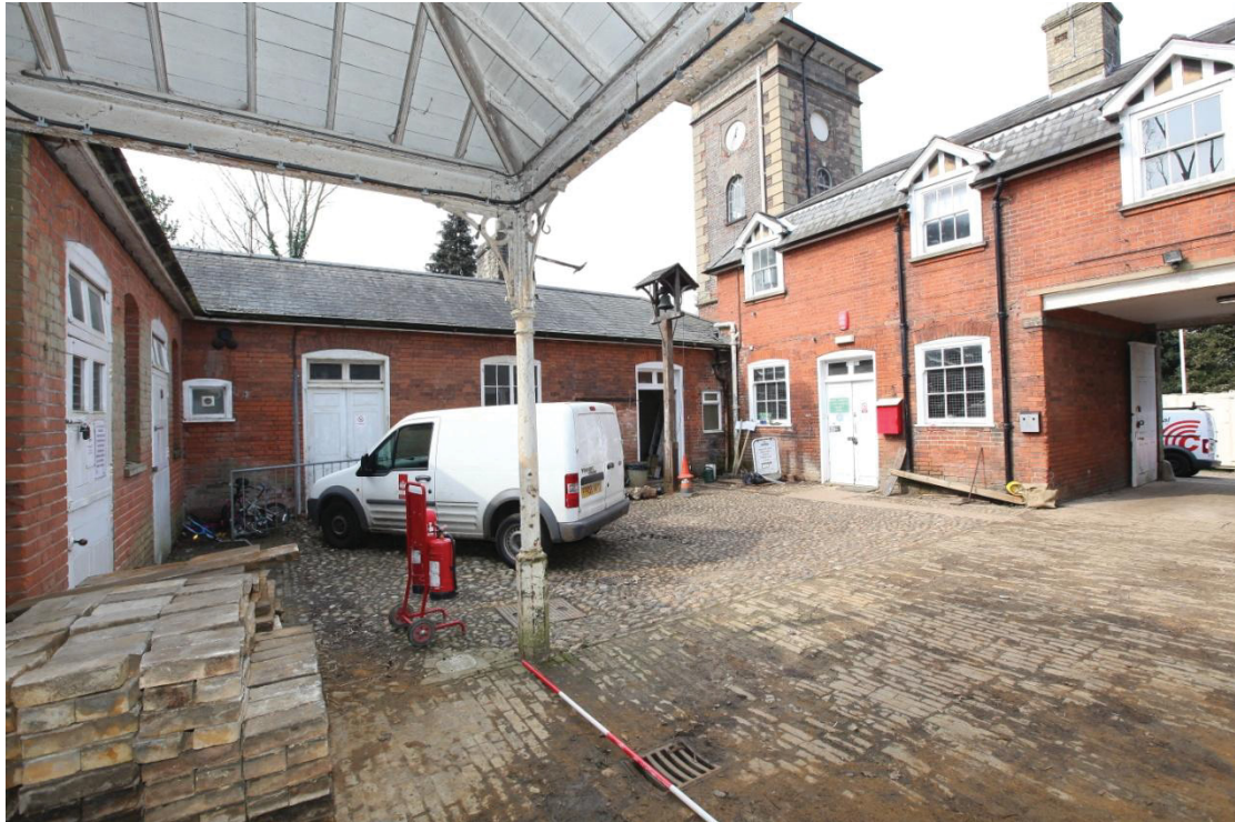
Illus. 3. The inner courtyard from the iron-framed open shelter (7) in its south-eastern corner showing the yard surface of cobbles and gault brick. The central door and windows of the double stable with two stalls (2) are visible to the left of the entrance on the right with the two doors of the southern stalls (8 & 9) on the extreme left. The doors of the much altered western range in the centre both open onto its eastern corridor (15).
