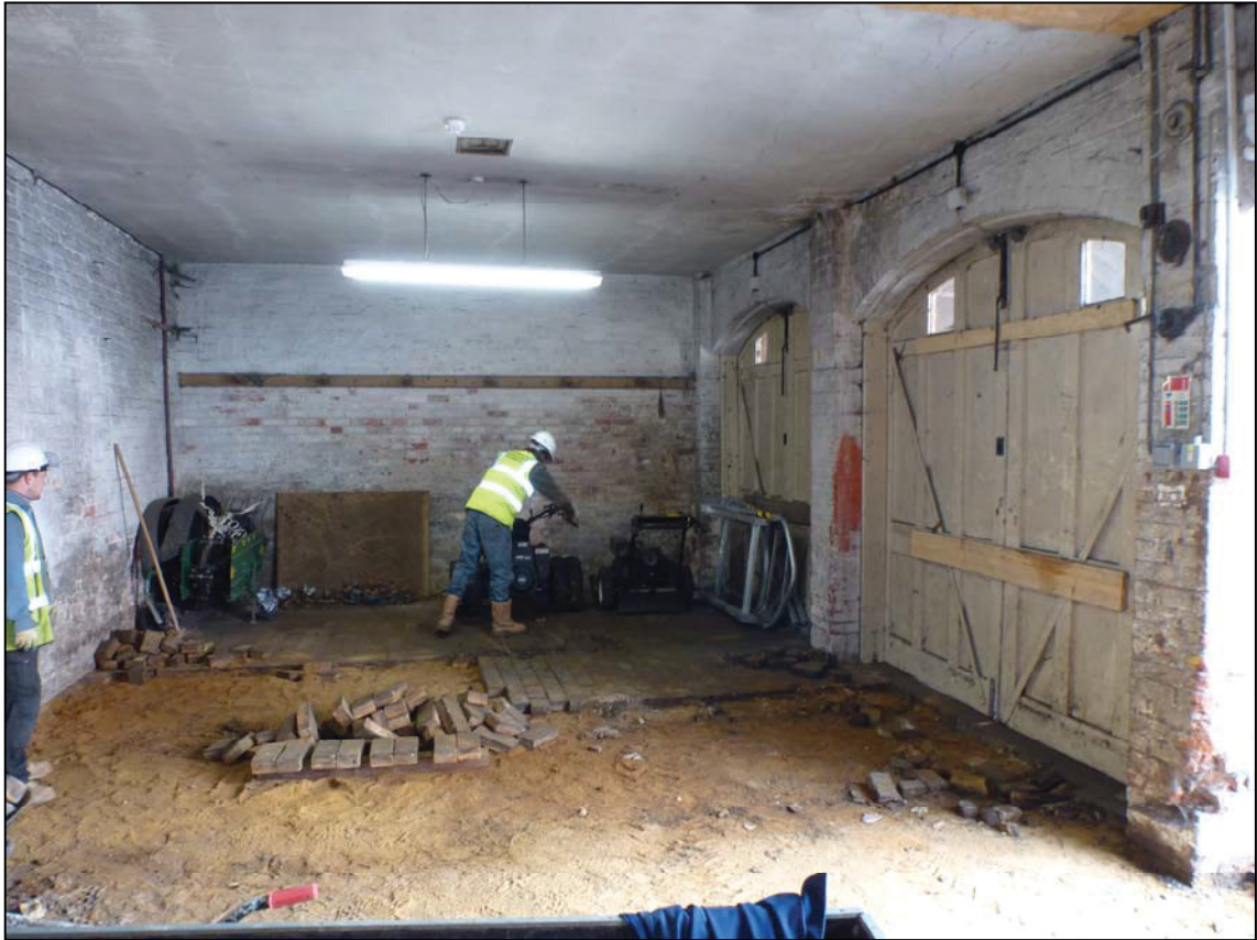
Plate 3. Stable block, coach house floor refurbishment, camera facing S
