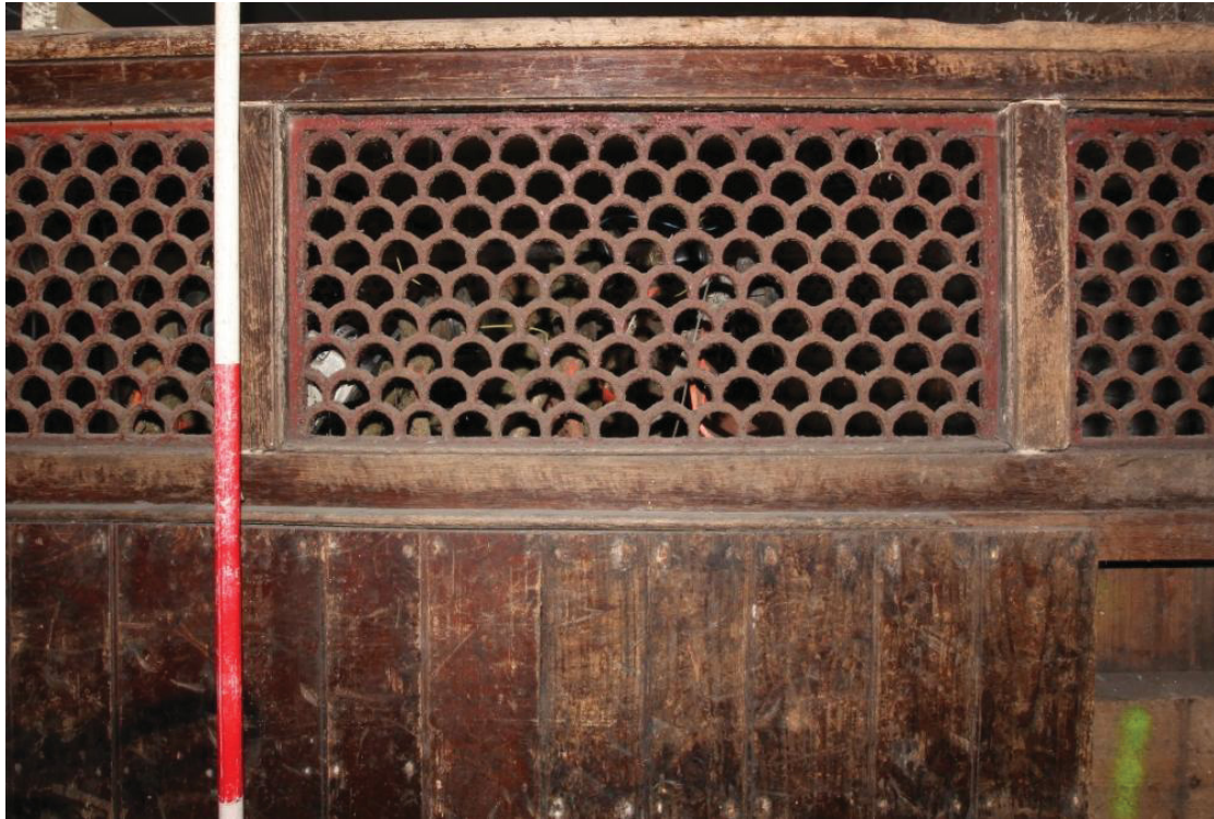
Illus. 13. A detail from the east of an original stall division in the triple stable (3) showing its red-painted decorative pierced iron grill.
