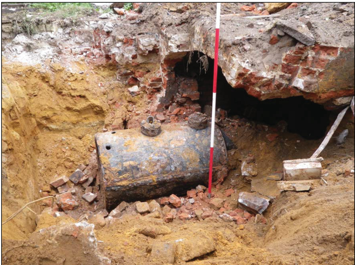
Plate 12. General view of boiler in boiler house 2, camera facing E
