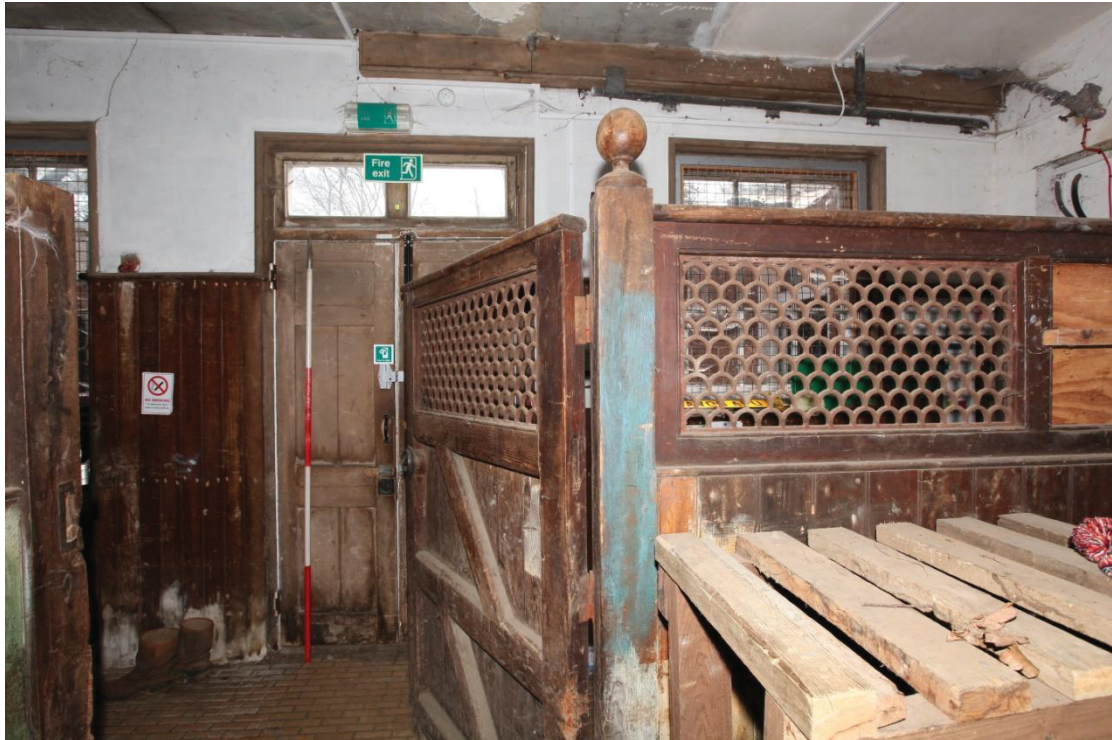
Illus. 9. The western stall of the double stable (2) viewed from the north and showing the turned wooden finial of the door post adjoining the southern corridor. The central entrance door and sash windows are visible in illus. A2.3 above.
