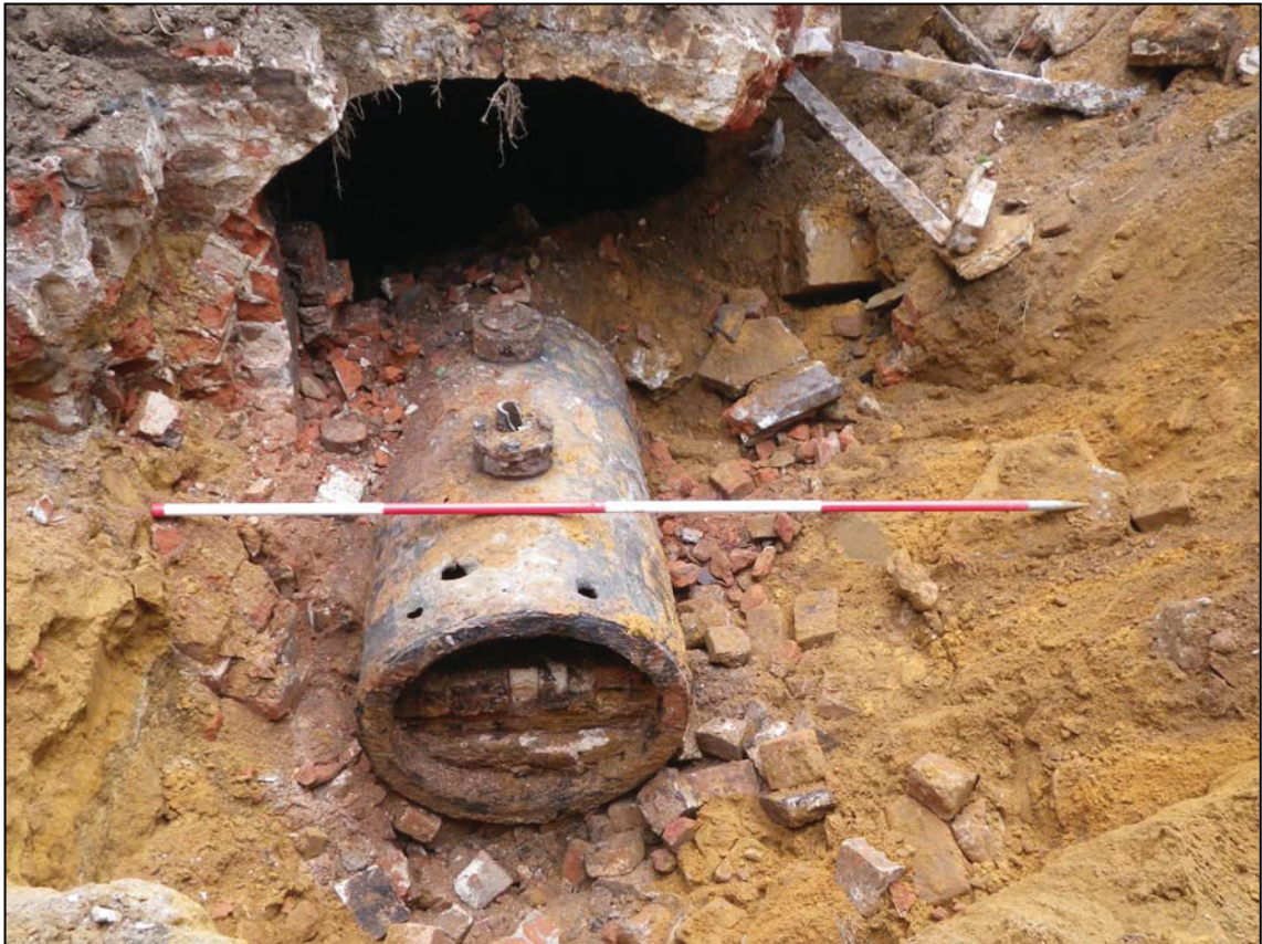
Plate 13. General view of boiler house 2, camera facing S
