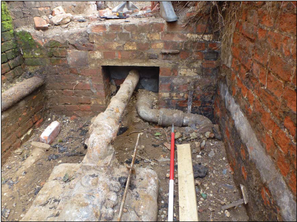
Plate 9. Southern wall of boiler house 1 showing repair/alteration, camera facing S
