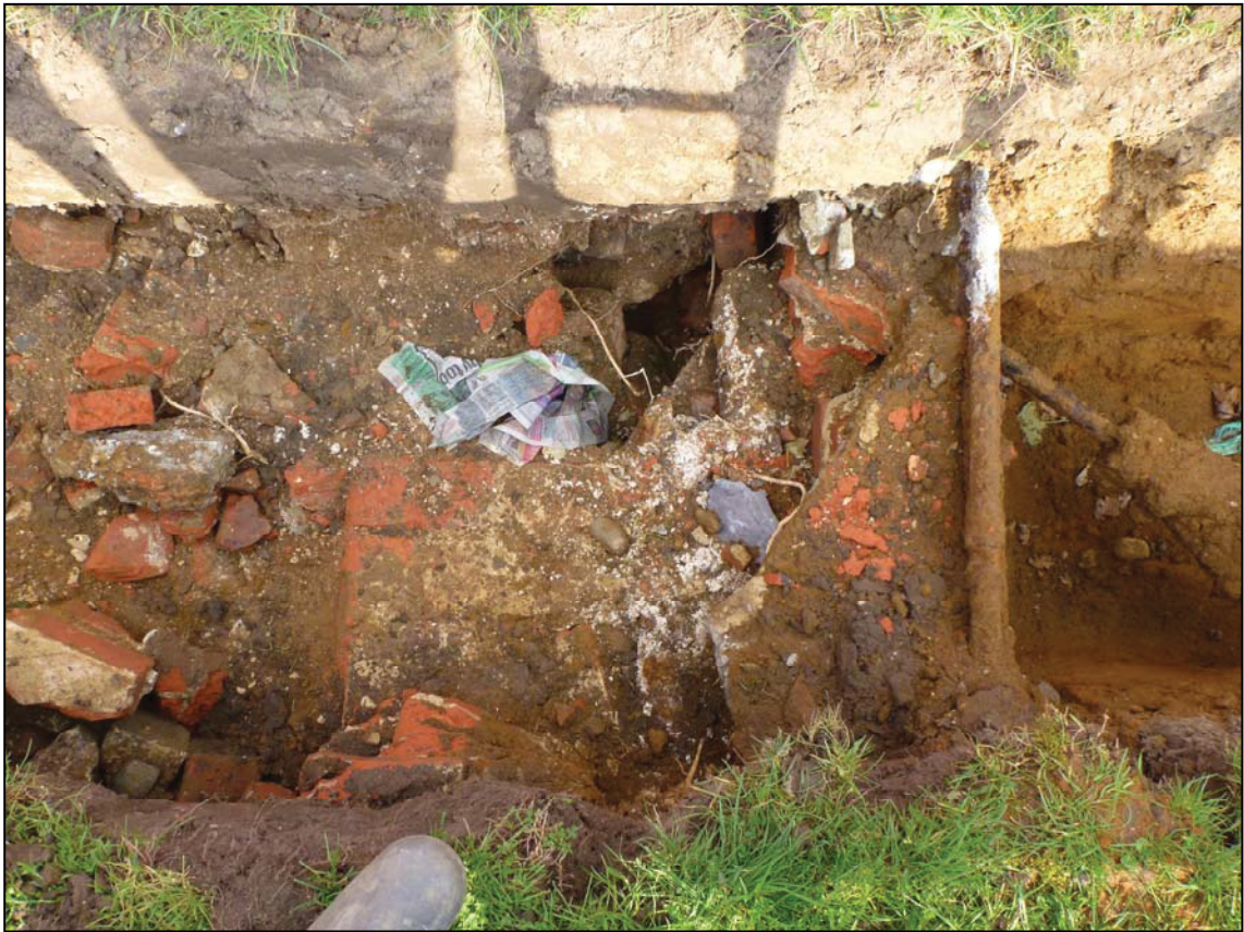
Plate 5. Brickwork, probable wall base, revealed in service trench, camera facing N
