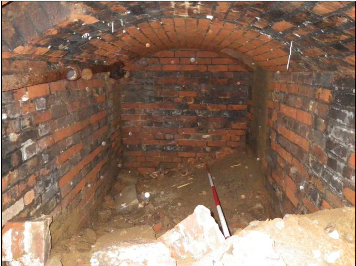
Plate 15. main chamber in boiler house 2, camera facing S
