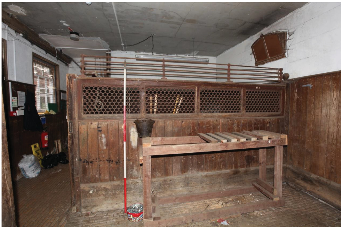
Illus. 8. The double stable (2) from the east showing its original boarded division against the western stall with its red-painted pierced iron grill and a turned wooden finial on the right. The horizontal bars appear to be an early addition.
