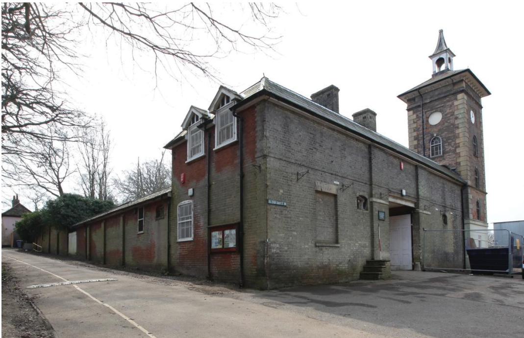
Illus. 2. The stable block from the north-east showing its gault-brick northern facade to the right and the red-brick eastern gable and single-storied eastern range (4-6) to the left. Note the original blind windows of the facade adjoining the two principal stables (2 & 3) and the mounting steps to the left of the entrance. The Queen Anne style of the clock tower is in stark contrast to the rest of the block and its red brick has been painted grey to match.
