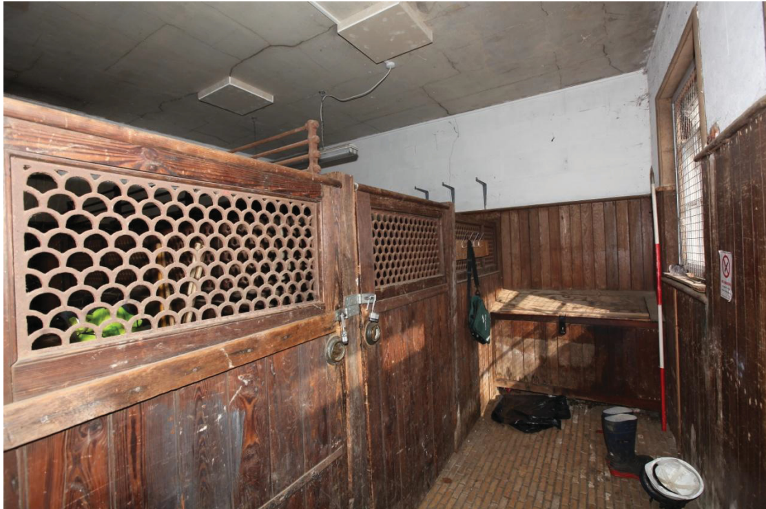
Illus. 7. The southern corridor of the double stable (2) seen from the west, with the courtyard window on the right. Note the ostensibly original grain bin at its eastern end and the gate to the eastern stall on the left.
