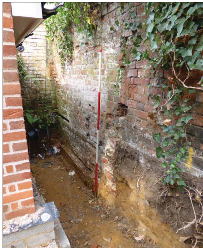
Plate 16. The north-south wall to the east of boiler house 2 (post construction) showing remnants of the retaining wall and other marks where a former glasshouse was attached, a clear vertical boundary to the whitewash is also visible
