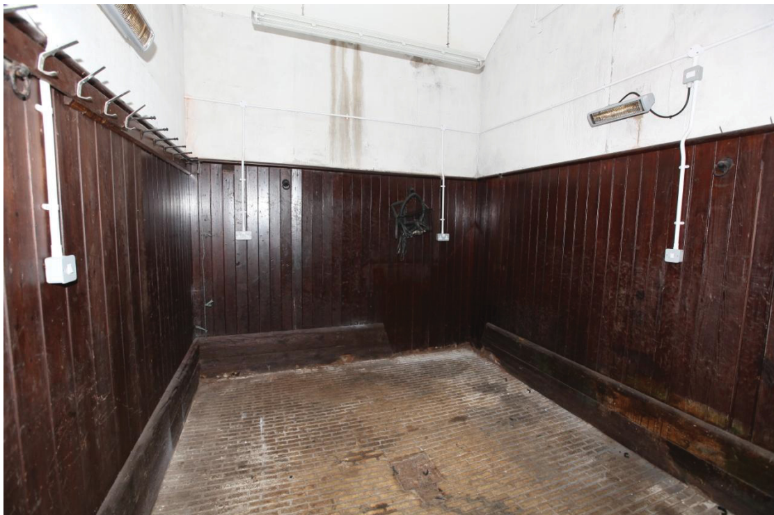
Illus. 12. The interior from the north of the later westernmost stall of the southern range (9) showing its ostensibly original wainscot and gault brick floor. The scar of a trough is visible above the interruption in the skirting board in the south-western corner.
