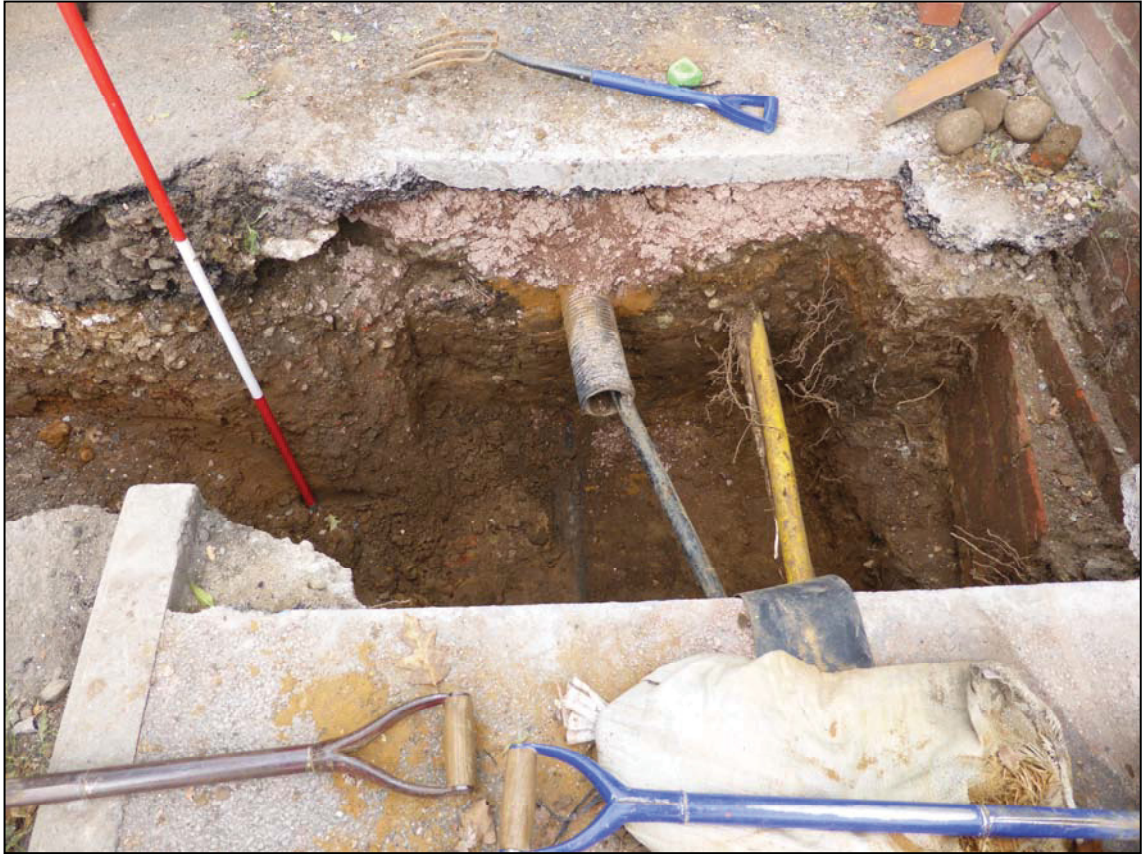
Plate 17. Cliff Lane entrance, foundation for eastern gate pier, camera facing N
