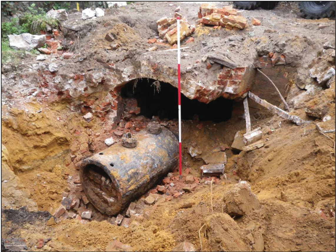
Plate 11. General view of boiler house 2, camera facing SE
