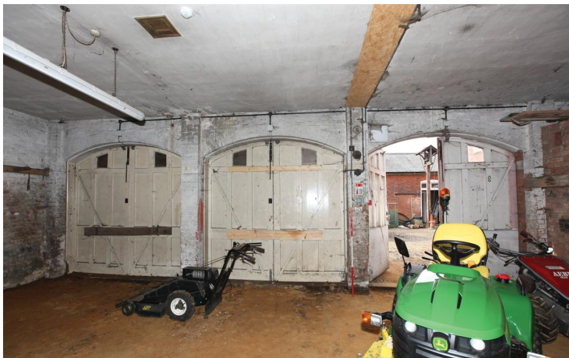
Illus. 6. The western internal elevation of the vehicle shed (6) in the eastern range showing its arched double doors with no evidence of internal partitions. A series of 20 th century wooden harness hooks is attached to the southern gable on the left and a 20 th century brick shed (5) blocks a fourth door on the right. The original gault floor bricks had been removed from the sand floor shortly before inspection.
