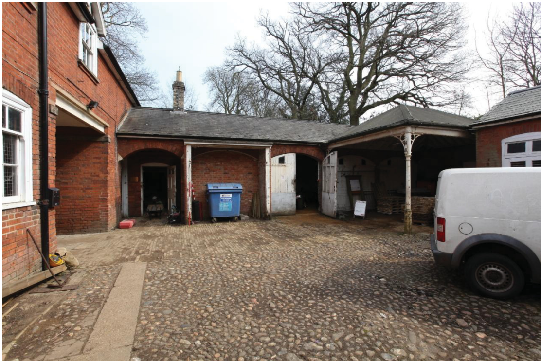
Illus. 4. The courtyard from the west showing the main entrance in the two-storied northern facade to the left and the arcade of the eastern range (4-6) in the centre. The left-hand arch opens onto both the triple stable (3) and single stall (4) with the blocked arch of the 20 th century shed (5) to its right.
