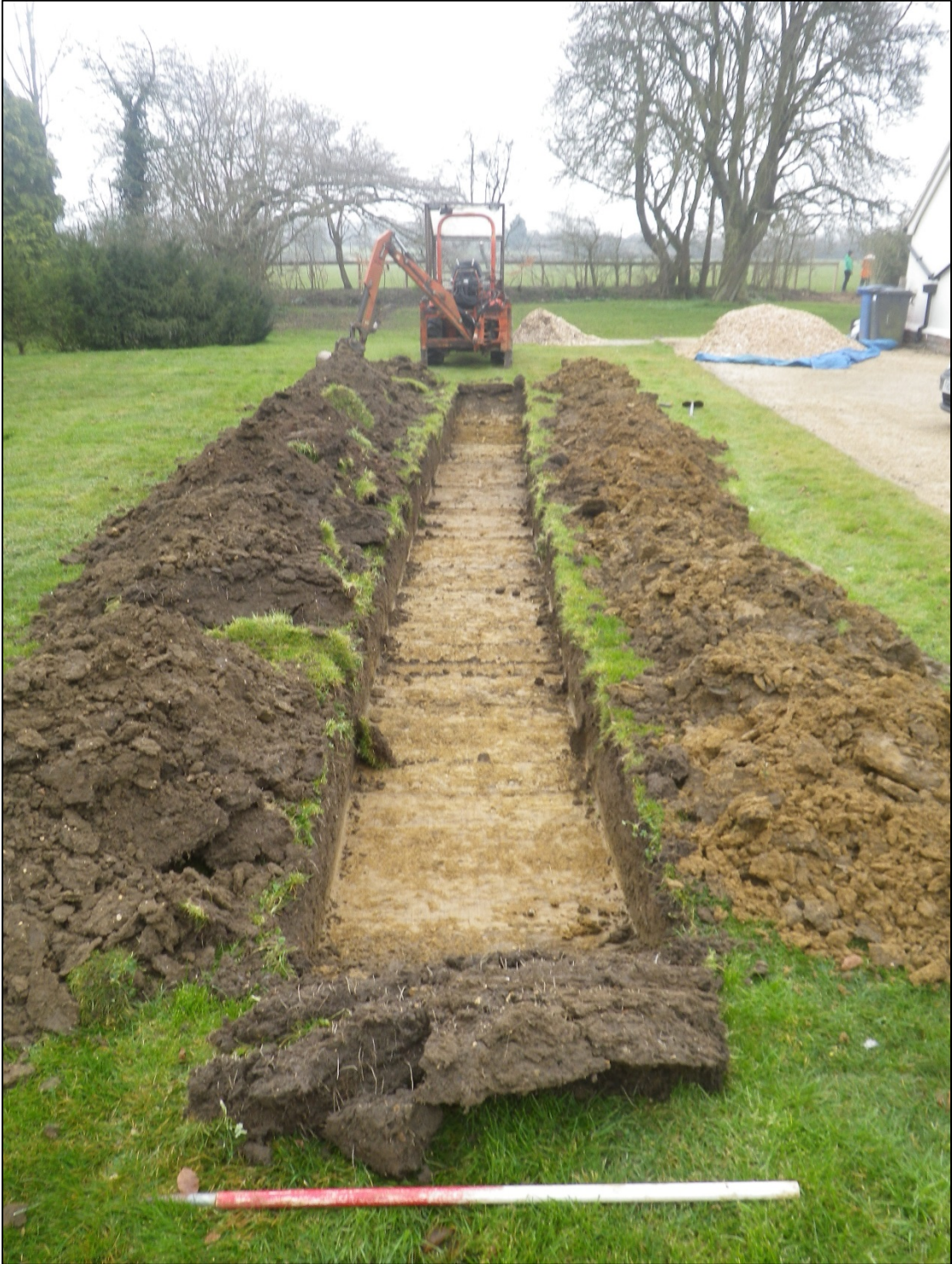
Plate 1. Excavated trench, 1m scale, looking south southeast.
