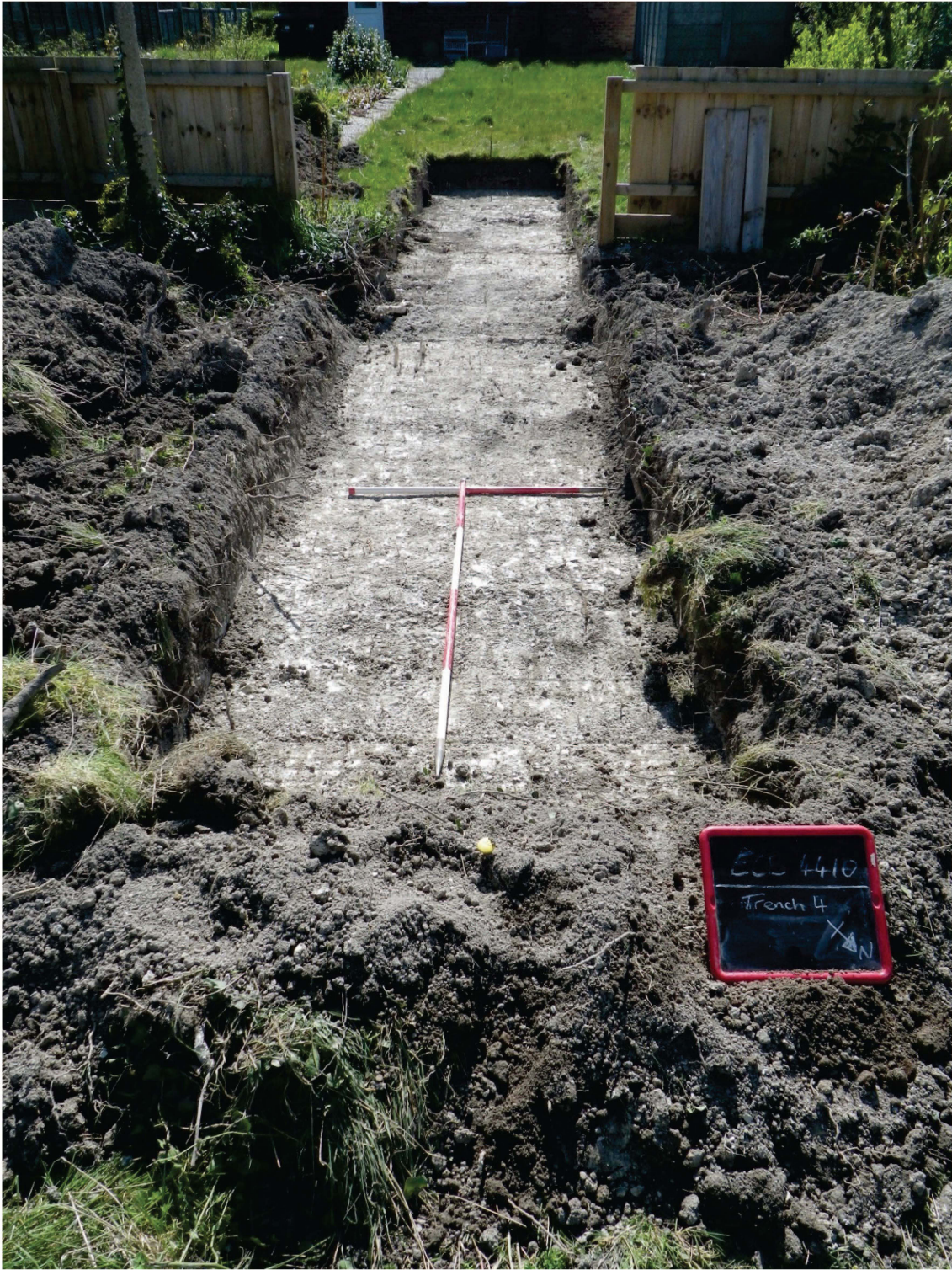
Plate 6. Trench 4, looking north-east (1m and 2m scale)
