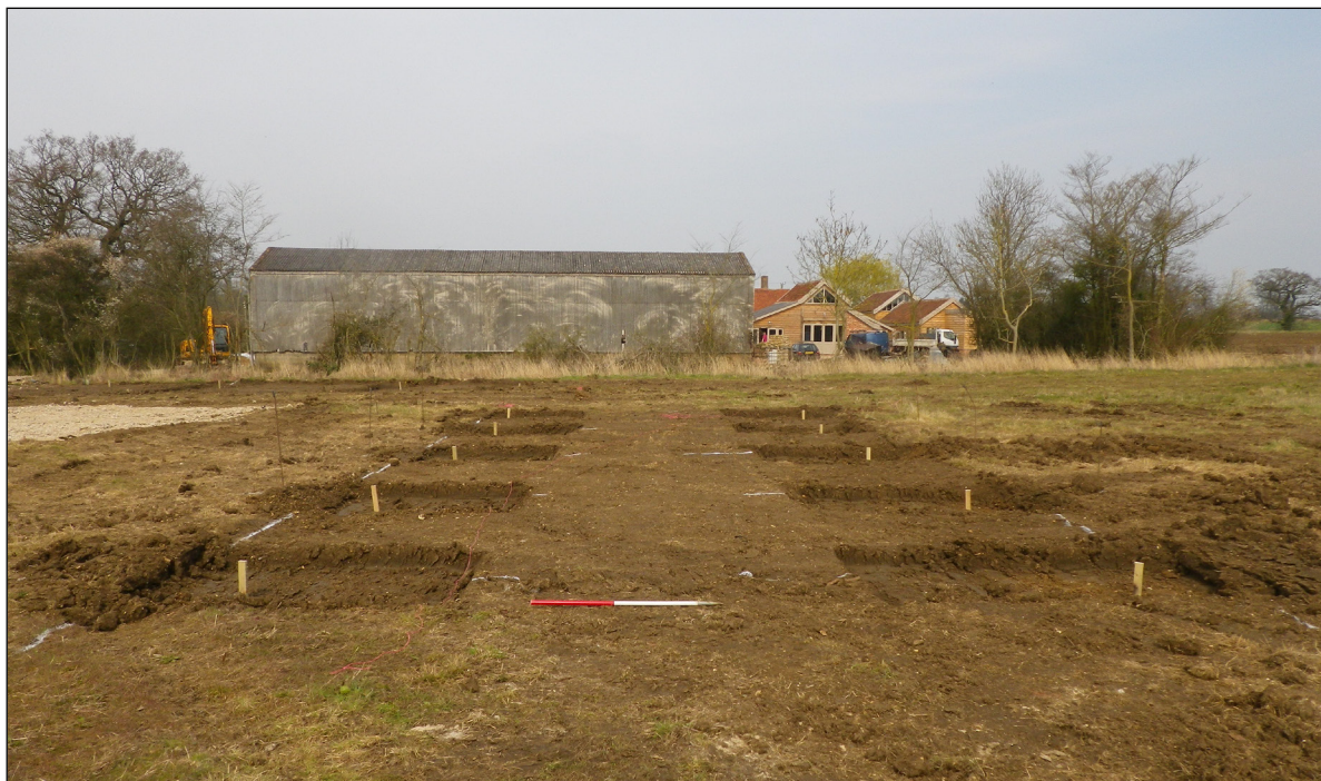
Plate 2. View of the excavated groundworks for chalet plot 4, looking north
