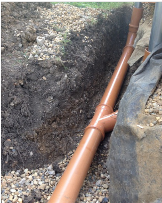
Plate 7. Excavated drain run
