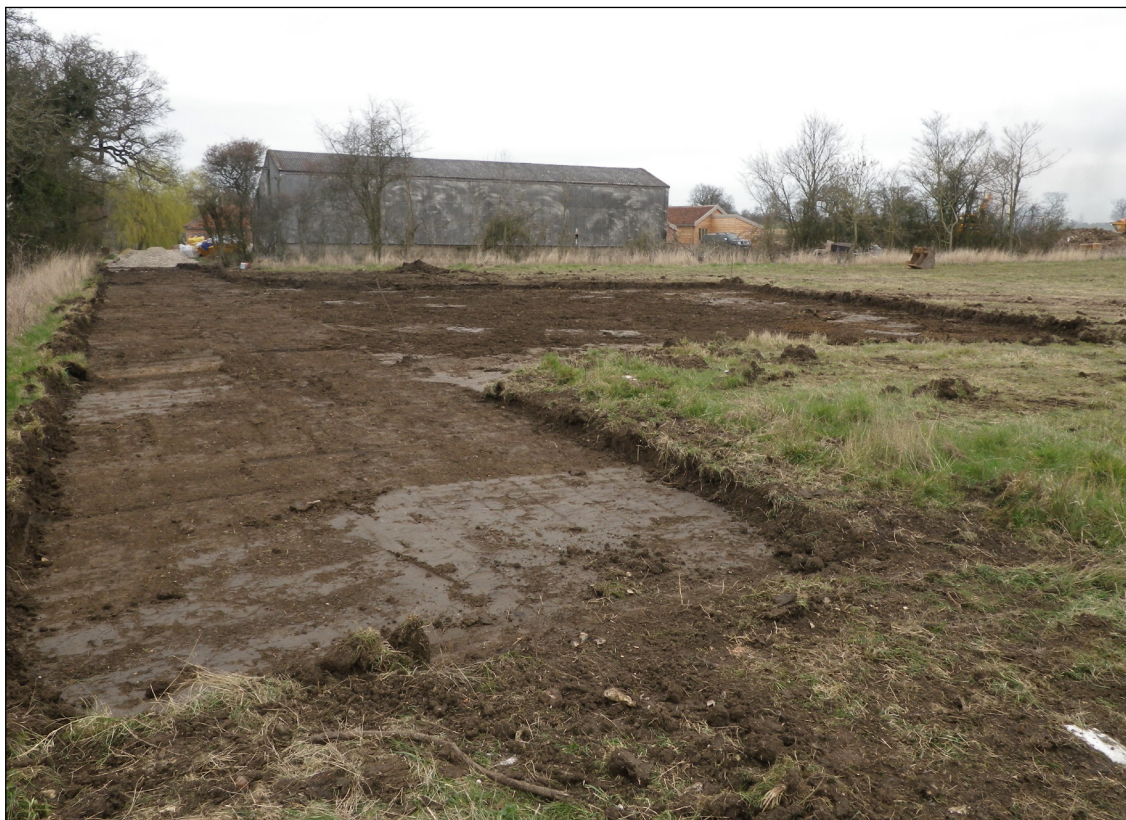
Plate 1. View of the stripped access road, looking north east
