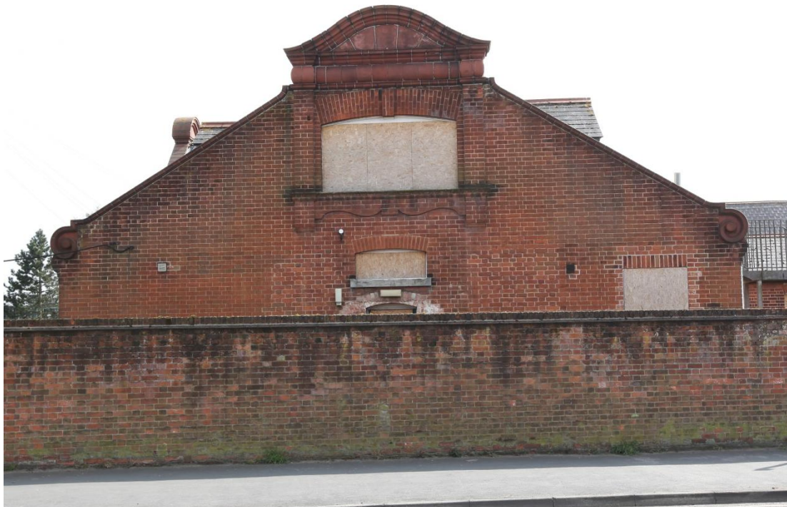
Illus. 4. The impressive Art Nouveau northern gable seen from Woodbridge Road. Note the terracotta volutes of the two corners to left and right, and the evidence of two blocked ground-floor windows flanking the later central door. The blocked first-floor windows are shown in illus. A2.12, but the high window beneath is hidden internally. The full photographic record includes several details of this gable.
