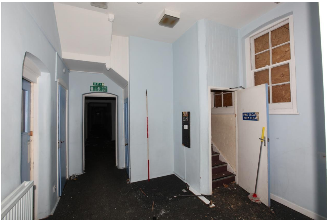
Illus. 14. The probably original staircase in the northern room of the early-20th century extension (B), viewed from the south and showing the door to the entrance lobby in the centre (see illus. A2.8). The stair has been enclosed and its treads renewed but the turned finials of its posts project from the ceiling. The curved jambs of the left-hand doorway are an original feature found elsewhere in structure B.
