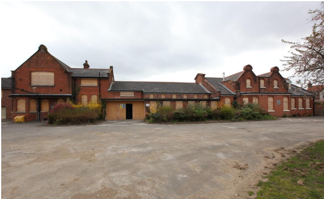
Illus. 1. The eastern facade of the former workhouse showing the original structure of the 1890s as illustrated in figure 2 on the right (A) and the early-20 th century extension (B) to the left. The original three-tiered central range has lost its upper tier of windows and the roof of the southernmost block has been remodelled and now lies behind the boarded modern entrance. The extension consists of the left-hand gable and the adjoining tall section containing the staircase shown in illus. A2.14 below.
