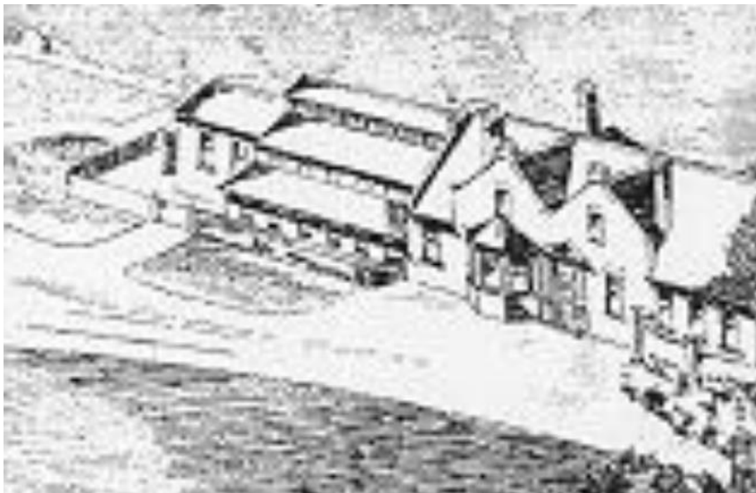
Figure 2a. A detail of figure 2 showing the detached northern block of the workhouse which forms the subject of this report. The shape of this original structure is still recognisable although the narrow upper tier of windows has been lost, and the position of its principal entrance to the south (left) as indicated by a gate remains unaltered.
