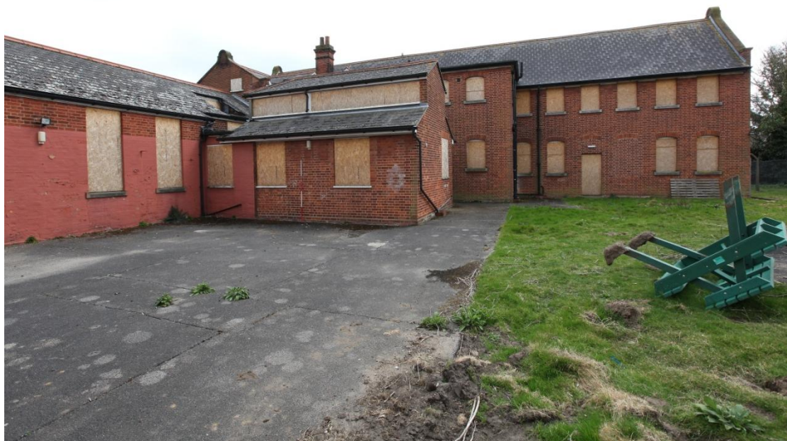
Illus. 6. The mid-20th century central extension (C2) from the north showing its roof profile with an upper tier of blocked windows reflecting the identical tier which has since been removed from the single-storied southern range of the original structure to the left (A). The large southern extension of the mid-20 th century (C1) is shown to the rear.
