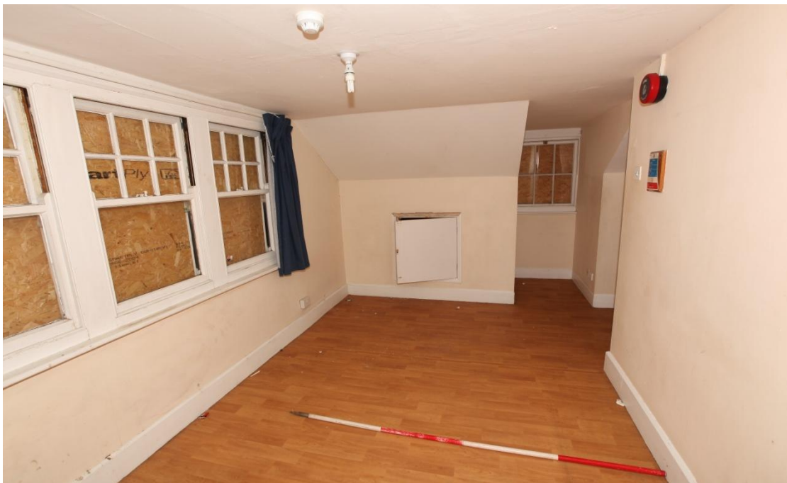
Illus. 12. The northernmost first-floor chamber of the original structure (A), seen from the west and showing the blocked windows in the Art Nouveau gable on the left with the secondary dormer window (not depicted in figure 2) on the right. All the partitions on the upper storey appear to represent 20 th century insertions.
