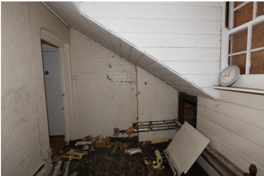
Illus. 18. The first-floor north-western chamber of the early-20th century extension (B) viewed from the north and showing the door to the staircase shown in A2.14 on the left. The painted brickwork and horizontal boarding of this space appears to be largely original as it served as a storage cupboard and escaped modernisation in 1995.
