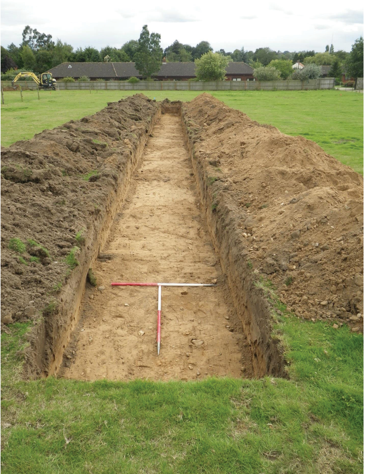
Plate 4. Trench 3. Looking south (1x2m and 1x1m scale)
