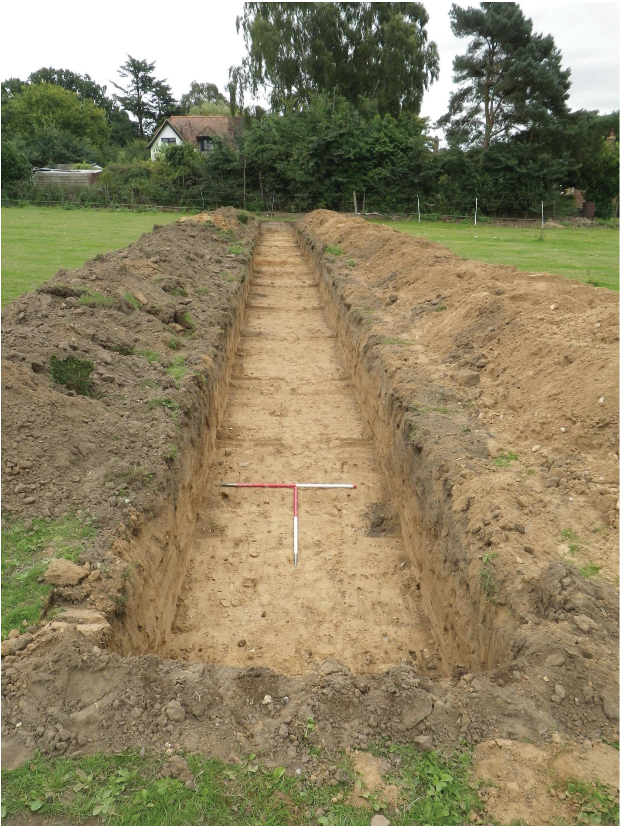
Plate 3. Trench 2, showing layer 0014. Looking east (1x2m and 1x1m scale)
