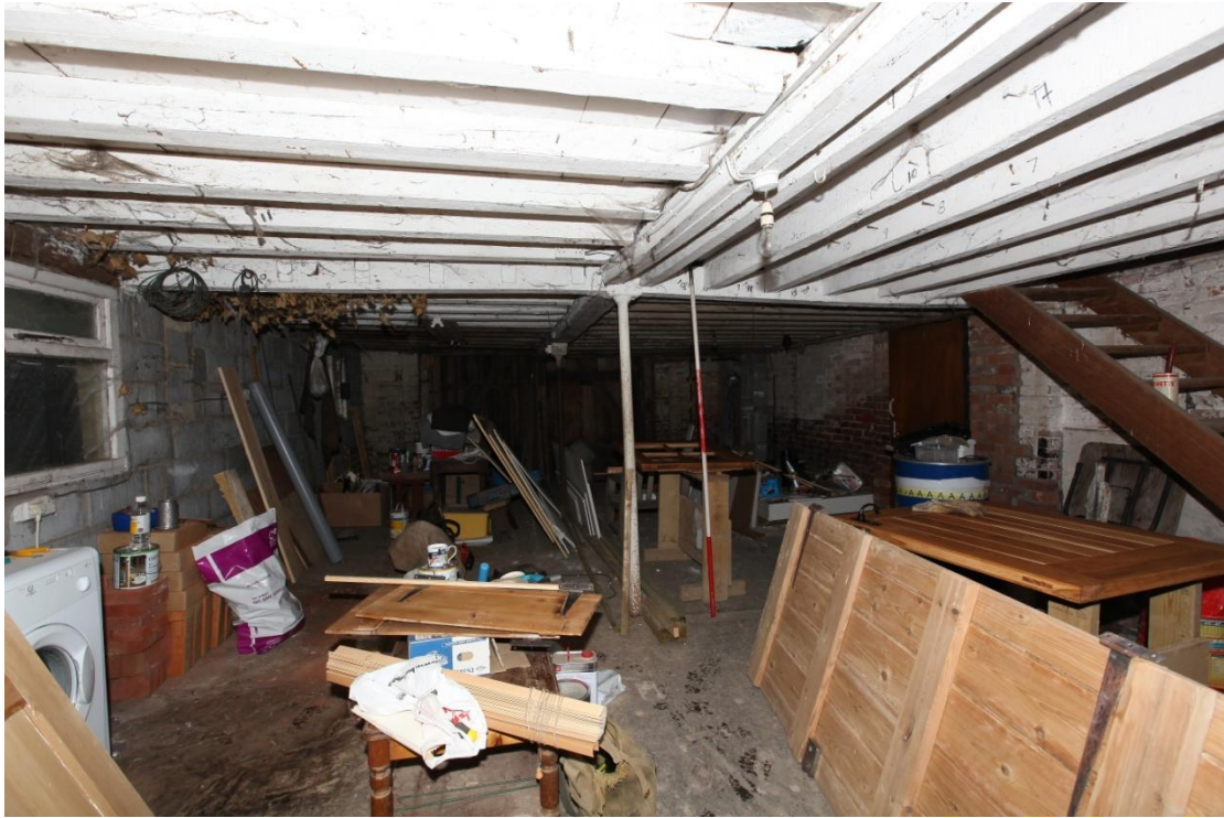
Illus. 7. The interior of the vehicle shed (1) from the north showing its early-20 th century secondary ceiling of painted deal joists supported by two axial iron posts. The lateral joists to the left have been altered as the principal joist is rebated for earlier axial joists. The stair to the right is a late-20 th century insertion.
