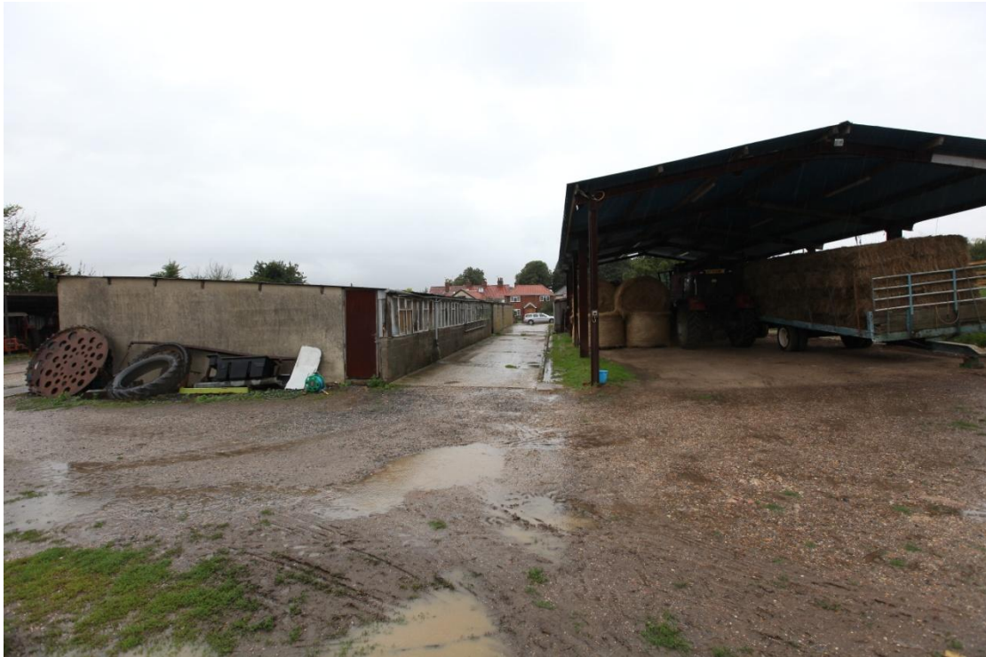
Illus. 13. The mid-20 th century farm buildings to the south of the site entrance, viewed from the south. An open-sided steel-framed Dutch Barn (Barn 4) is shown to the right of the much altered single-storied range of cement-block pig sheds (Barn 5). Included for site context.
