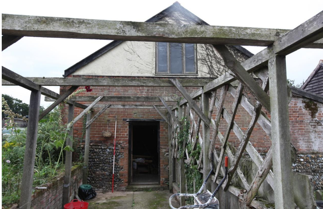
Illus. 5. The northern external gable of the vehicle shed (1), showing its 20th century window and an ostensibly secondary door with cement-mortared brick jambs interrupting the flint-rubble plinth.
