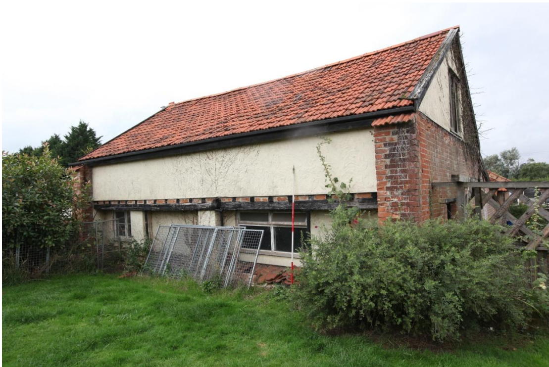
Illus. 4. The cement-rendered eastern wall of the vehicle shed (1) rebuilt in circa 1980 and recessed behind its original brick corners to left and right. The original wall is understood to have consisted of flint-rubble, and the pantiles at ground level protect the remains of its foundation. The treble-tiled roof also dates only from circa 1980.
