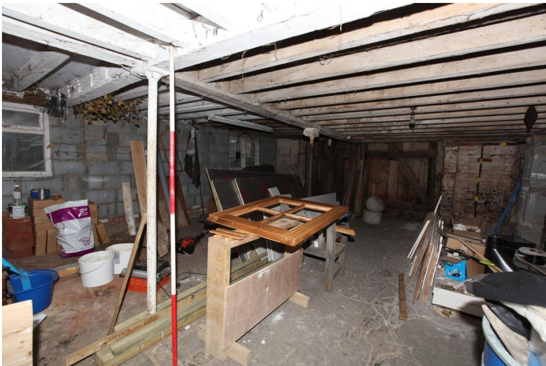
Illus. 8. The interior of the vehicle shed (1) from the north-west showing its two axial iron posts with the southern gable doors in the rear and the cement-block fabric of the eastern wall on the left. The floor consists entirely of 20 th century concrete.
