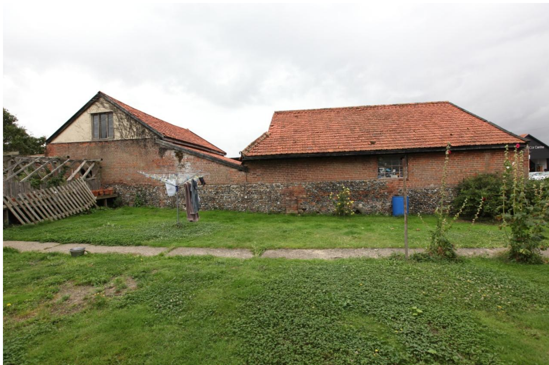
Illus. 6. The northern exterior of Barn 1 showing the vehicle shed (1) to the left and the surviving red-brick and flint-rubble wall of the contemporary buildings on the site of the lean-shed (1a) and storage shed (1b). The rest of these two structures dates only from the second half of the 20 th century. The flint-rubble plinth may have been retained from an earlier yard wall, although there is no obvious sign of this on the tithe map.
