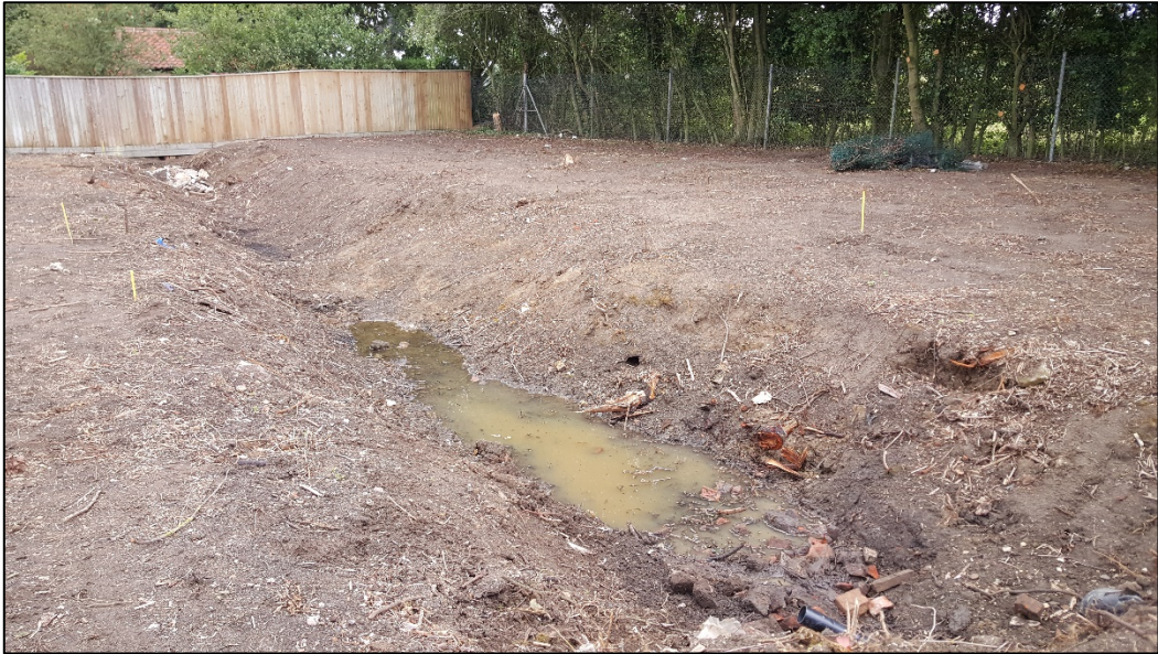
Plate 3. 0002 boundary ditch, prior to hardcore infilling, facing north
