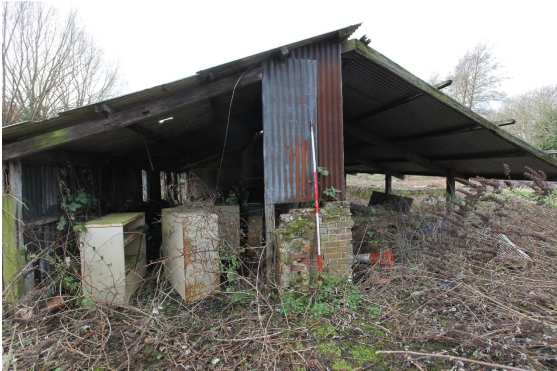
Illus. 11. The eastern gable of the linear sheds showing the 20 th century brick extension to the original flint-rubble wall which divides the contemporary extension to the mid-19 th century eastern shed (1b) on the left from the mid-20 th century open-sided shed (1c) on the right.
