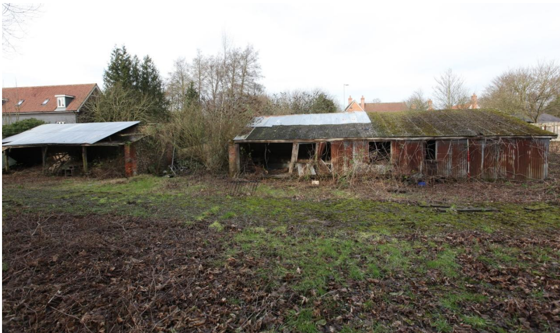
Illus. 8. The linear open-sided sheds from the south, showing the original gap between the western shed (1a) on the left and the eastern shed (1b) on the right. The latter was extended to the right in the mid-20 th century, as indicated by the change in roof covering from corrugated iron to corrugated asbestos.
