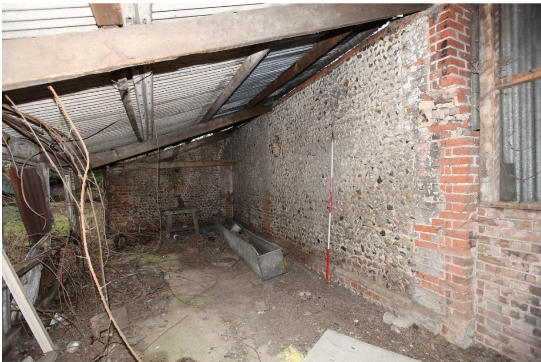
Illus. 10. The interior of the mid-19 th century eastern shed (1b), seen from the east. The flint-rubble northern wall terminated at the red-brick dressing on the right, which abutted a timber-framed shed shown in figure 3, but was extended in brick in the mid-20 th century. The softwood rafters are 20 th century replacements.
