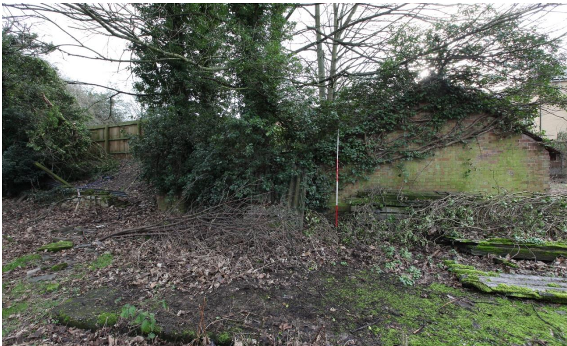
Illus. 6. The Fletton-brick northern gable of the circa 1900 pantiled shed (3a, right) with the low stub wall (4) adjoining its north-eastern corner on the left. This stub wall or plinth consists of two sections on slightly different alignments: a predominantly brick section abutting the shed, largely hidden by vegetation, and a section of re-used dressed stone to the left of a narrow gap that presumably served as a doorway. The right-hand pier of this doorway consists of early- to mid-19 th century brickwork incorporating further re-used stone. These walls ostensibly survive from the ‘eastern barn’ depicted in 1845 (figure 2) and its mid-19 th century eastern extension (figures 3 and 4).
