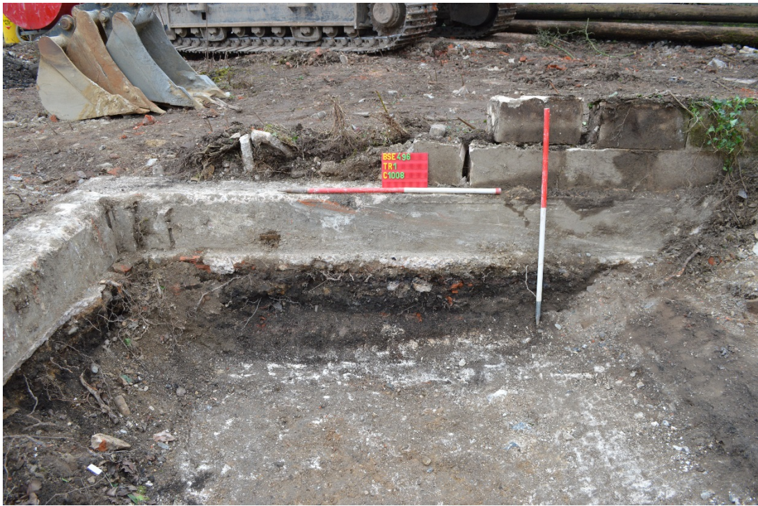
Plate 3. Trench 1, wall 0008, facing north
