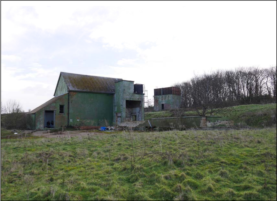
Plate 3. General view of the Generator House, fuel store and water tower from the southwest
