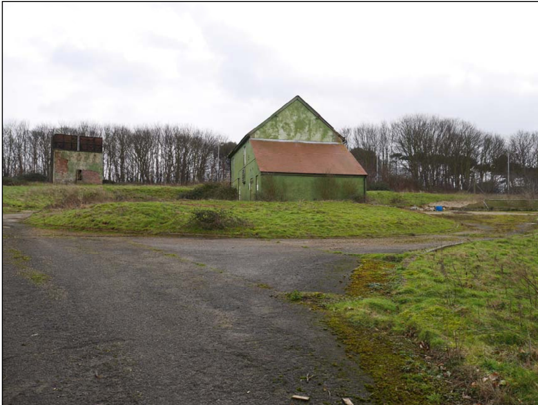
Plate 5. Generator House and water tower from the northwest
