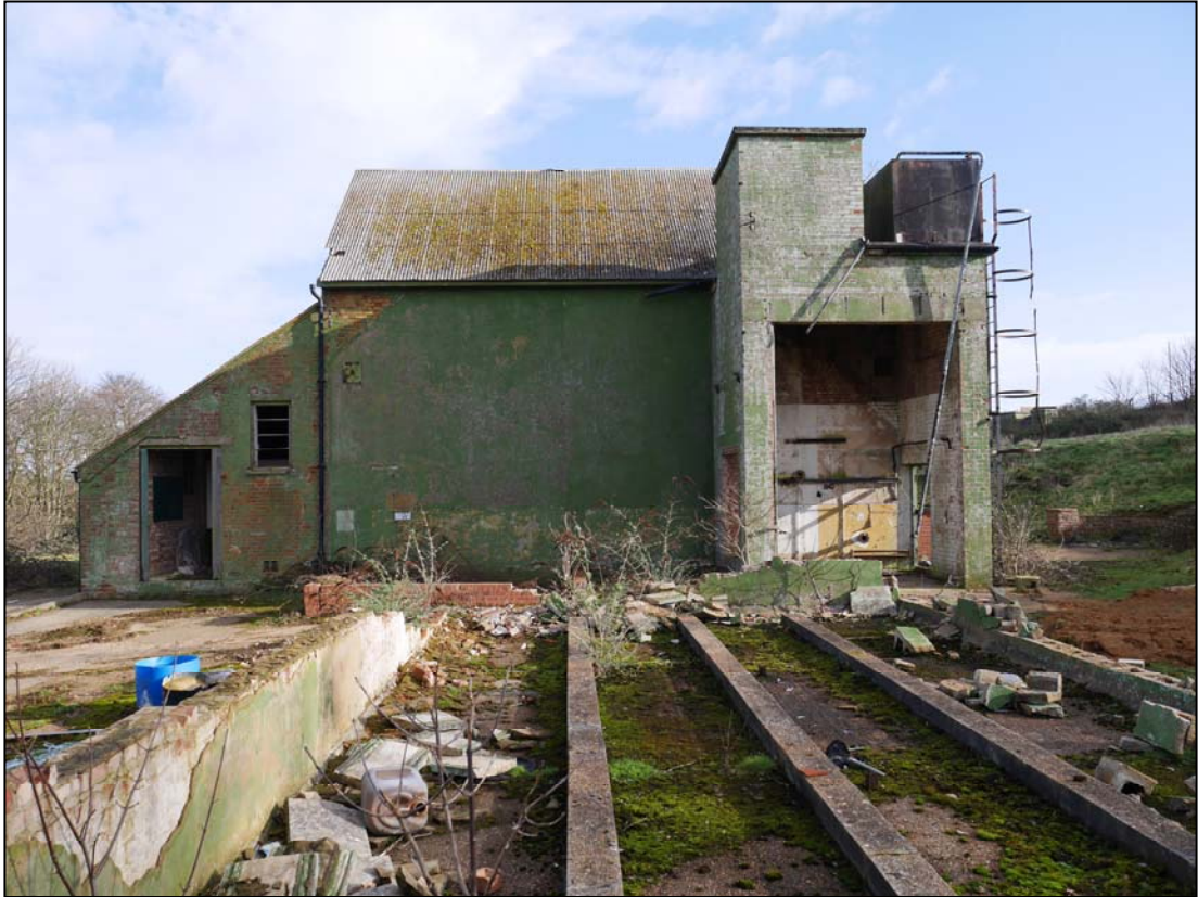
Plate 7. Generator House, camera facing northeast
