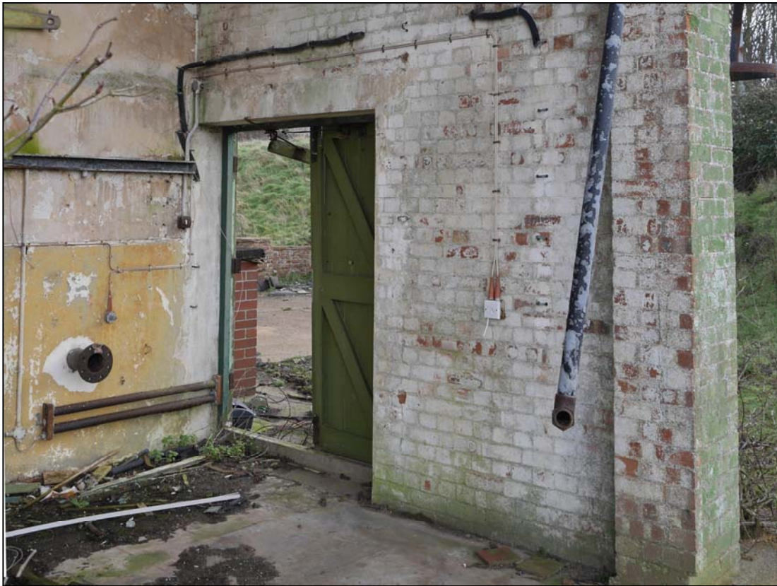
Plate 33. Double doors in southeast wall of cooling tower
