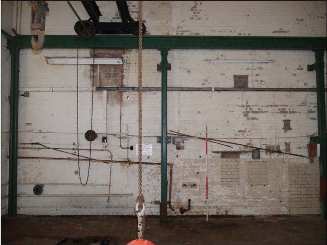
Plate 67. Southwest wall (southeast section)
