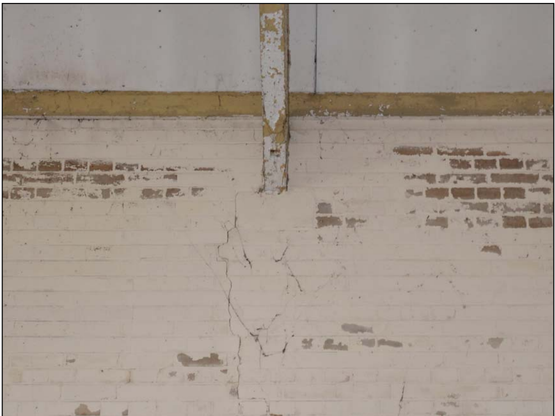
Plate 48. End of roof truss resting on ?concrete block built into brickwork
