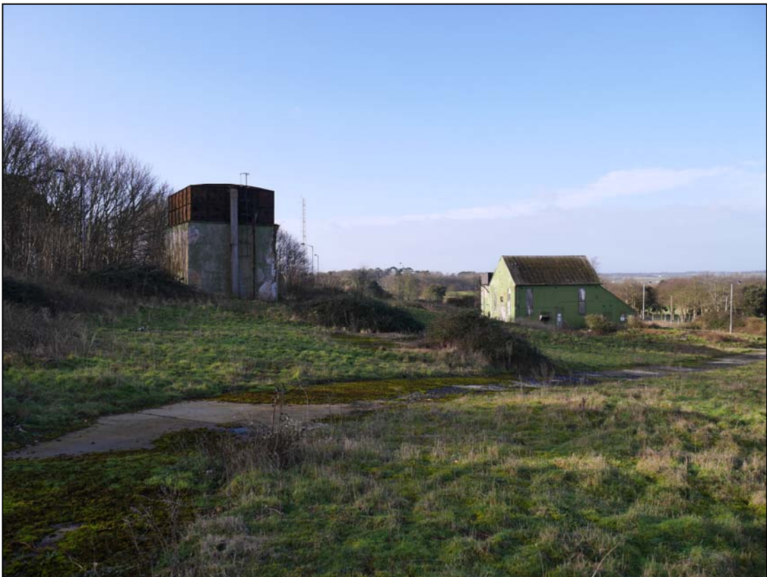
Plate 4. Generator House and water tower from the east
