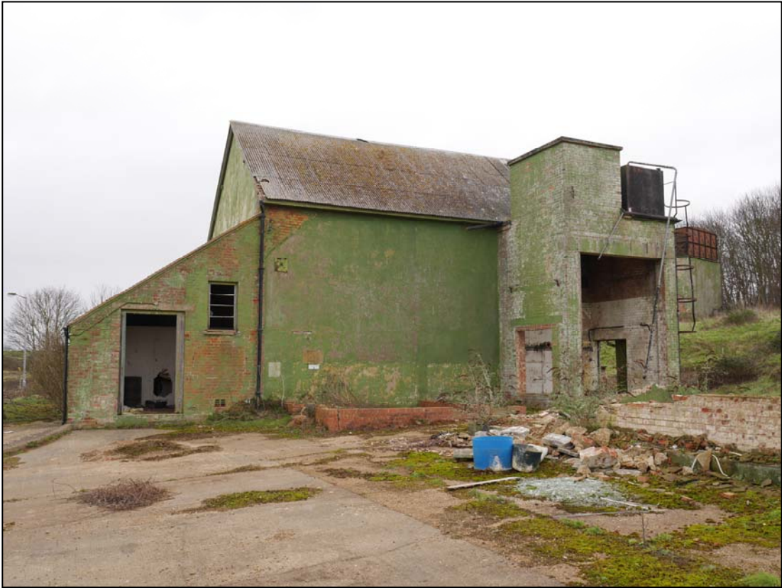
Plate 13. Generator House, camera facing east
