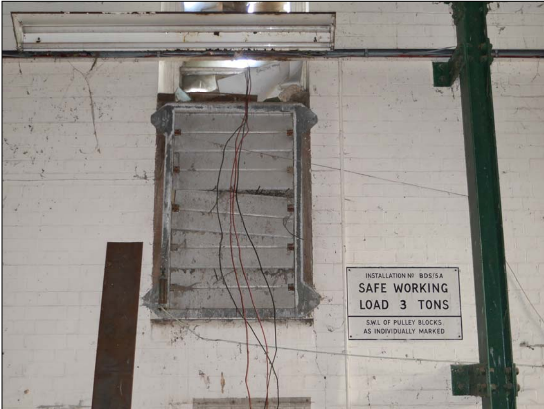
Plate 17. Mechanically operated louvered vent on main room window, internal view
