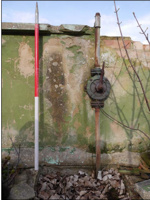
Plate 77. Sump and hand pump within fuel storage area, camera facing northwest
