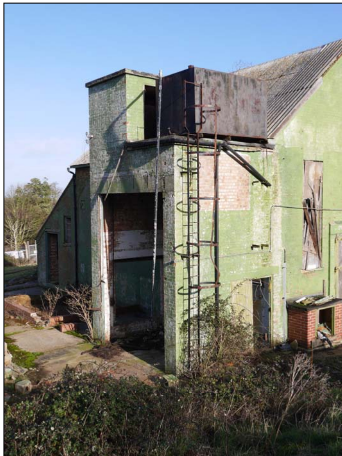
Plate 28. View of the cooling tower, camera facing north
