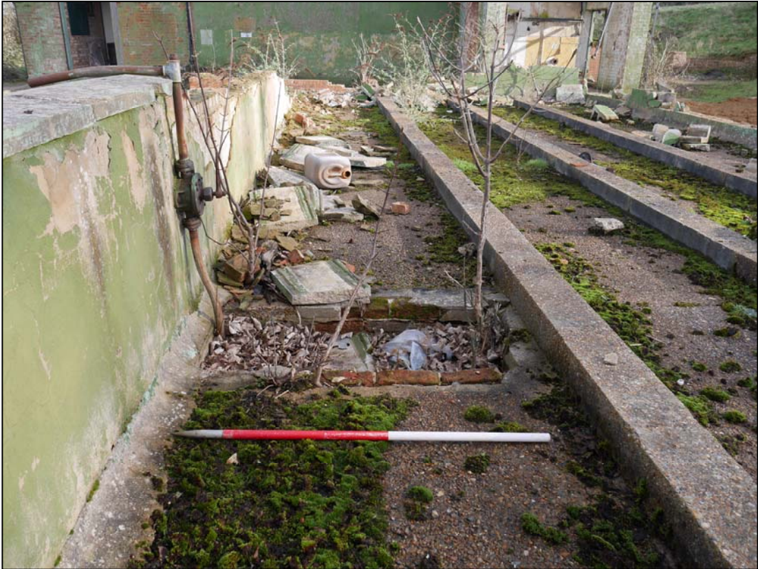
Plate 75. Sump and hand pump within fuel storage area, camera facing northeast
