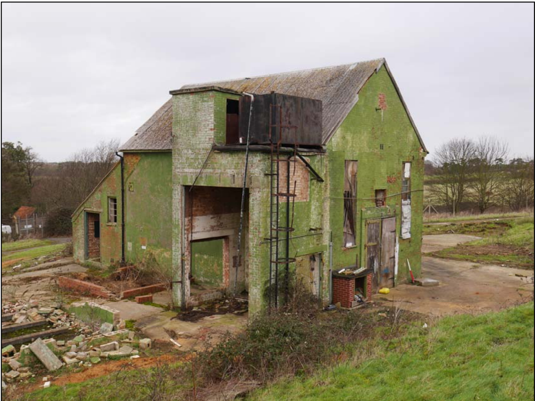
Plate 12. Generator House, camera facing north
