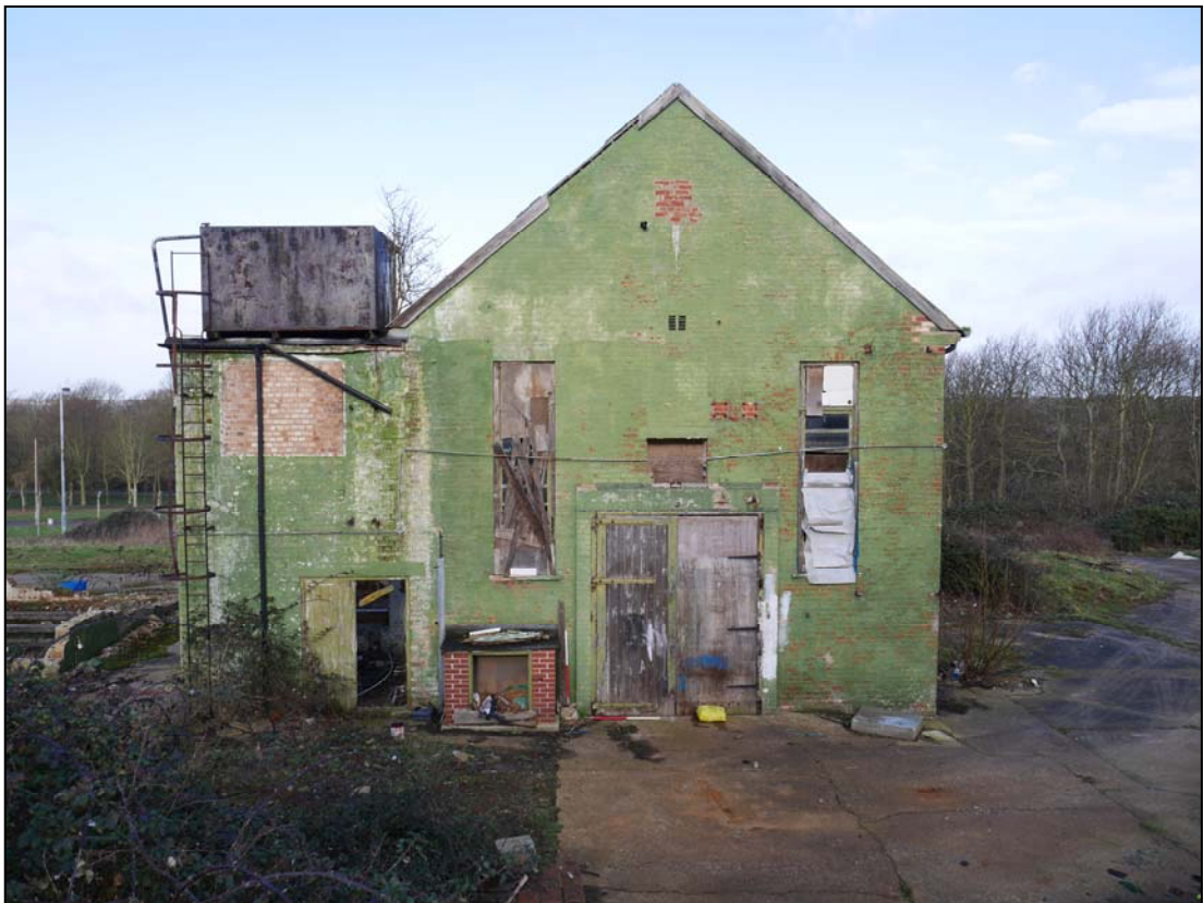
Plate 8. Generator House, camera facing northwest
