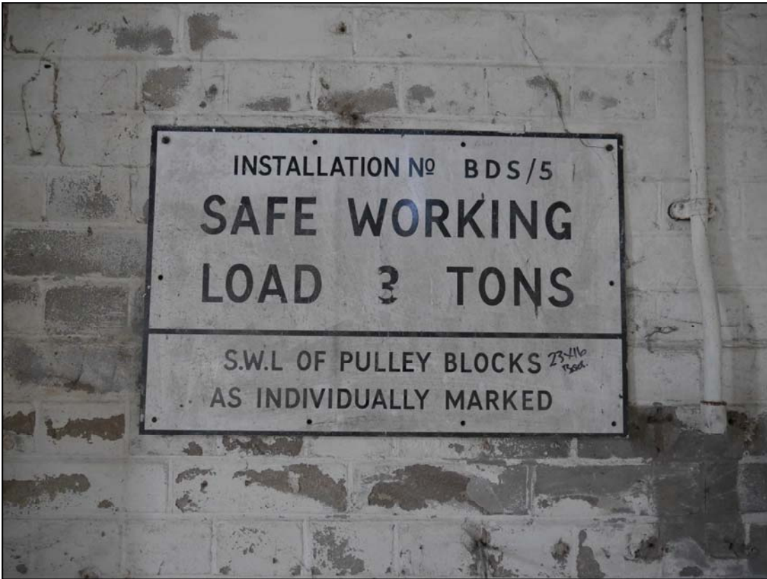
Plate 59. Weight limit sign relating to the overhead gantry crane
