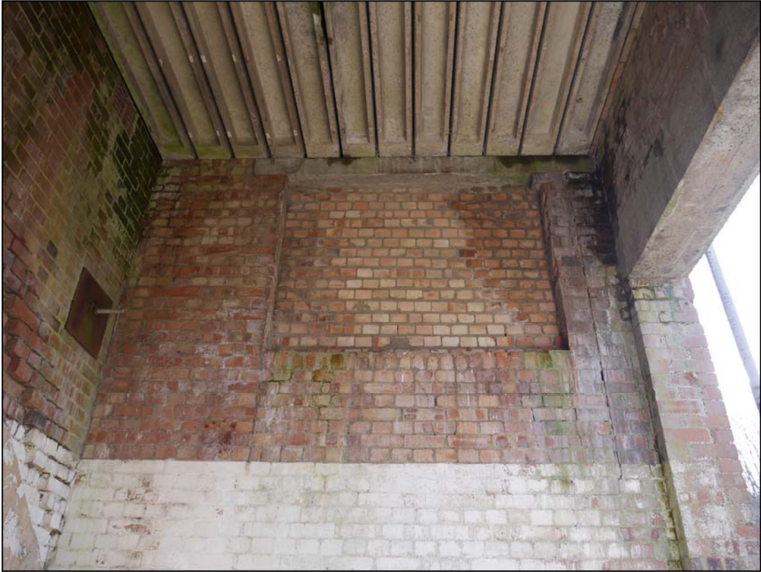
Plate 35. Bricked up opening high in southeast wall of cooling tower
