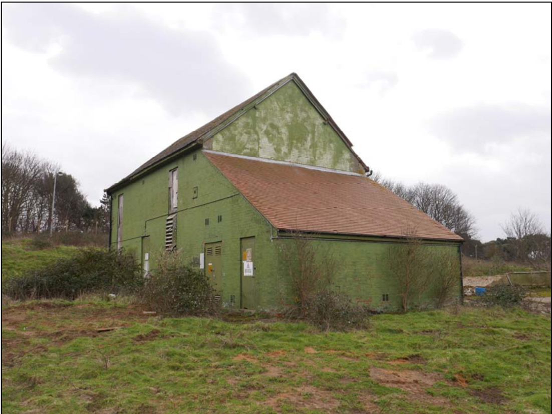
Plate 14. Generator House, camera facing south
