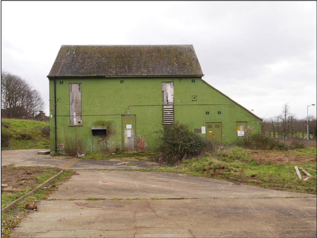
Plate 9. Generator House, camera facing southwest
