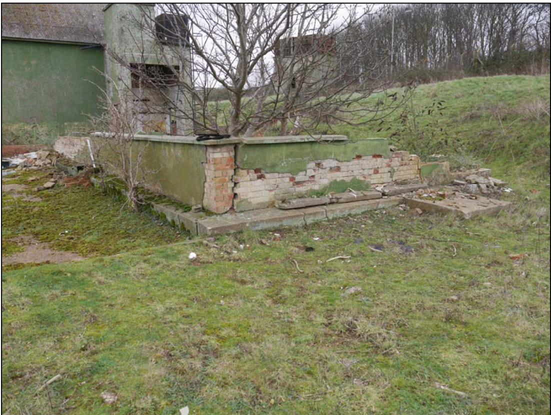
Plate 72. The fuel storage area, camera facing east
