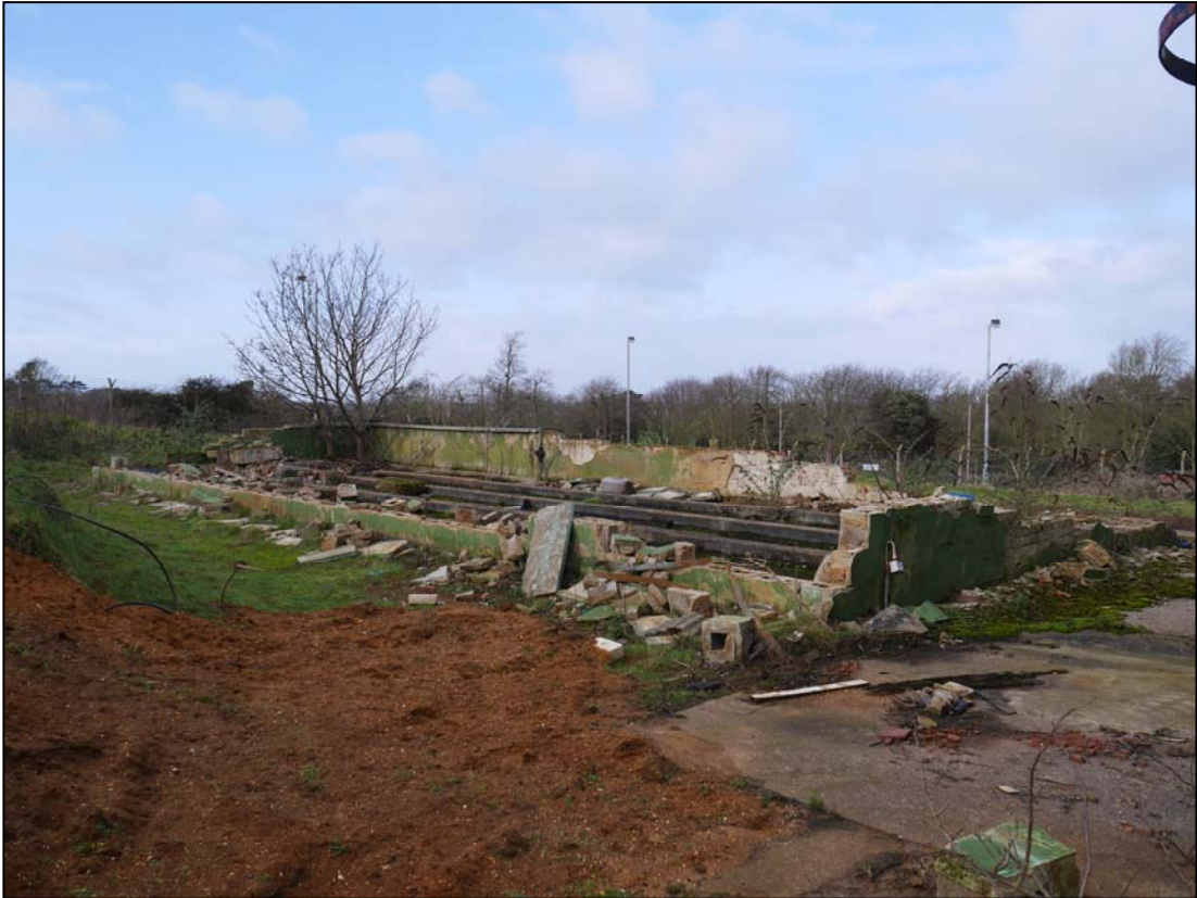
Plate 71. The fuel storage area, camera facing west
