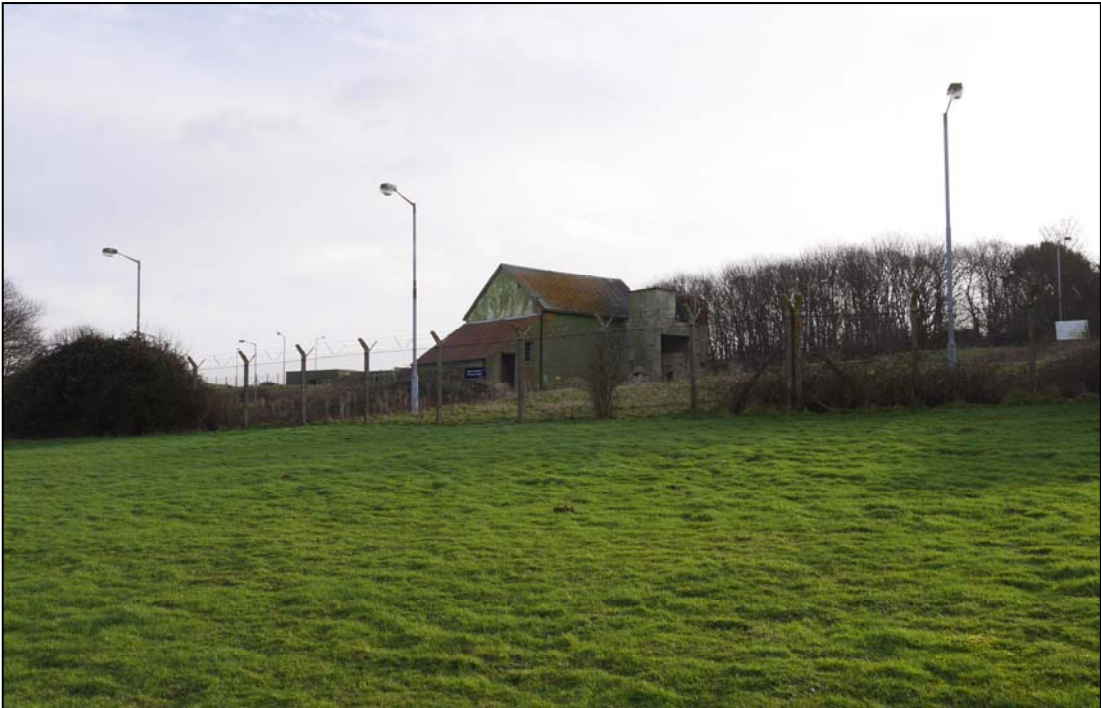
Plate 1. General view of the Generator House from the northwest showing the security fence and lighting
