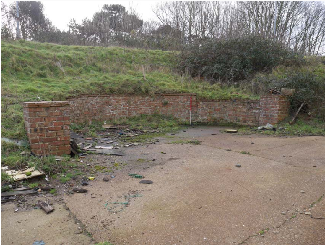
Plate 39. Curving revetment wall to the southeast of the Generator House
