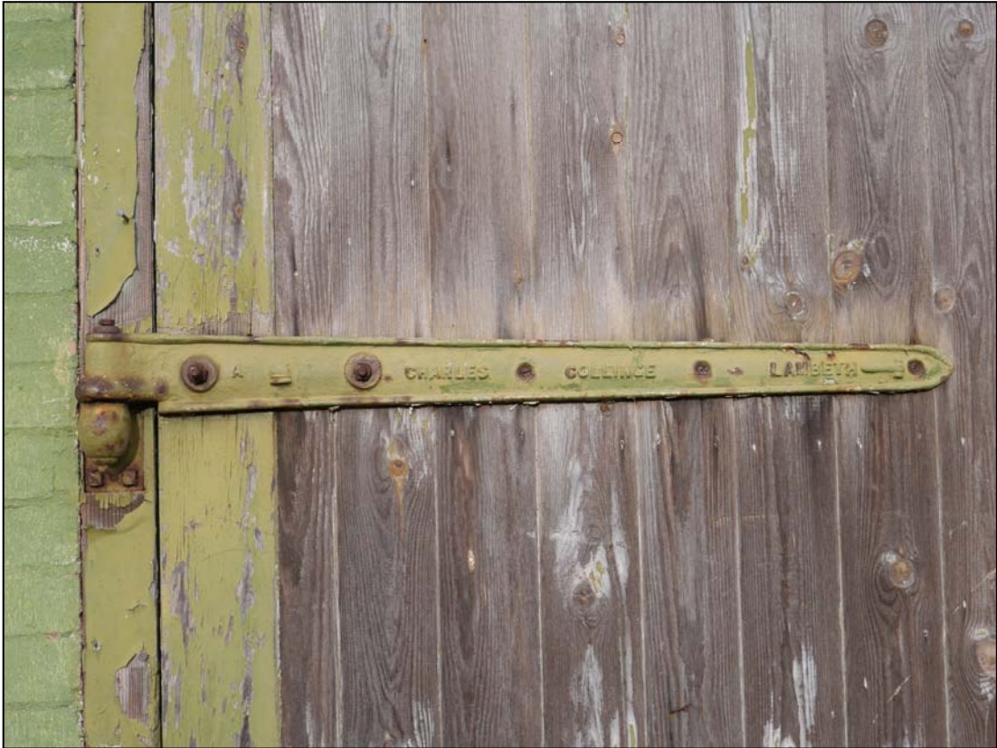
Plate 21. Hinge on main entrance door
