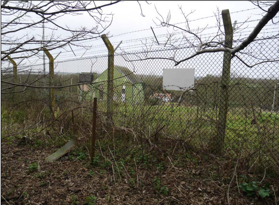
Plate 2. Generator House viewed through the security fence on the southeast side of the enclosed area, camera facing north
