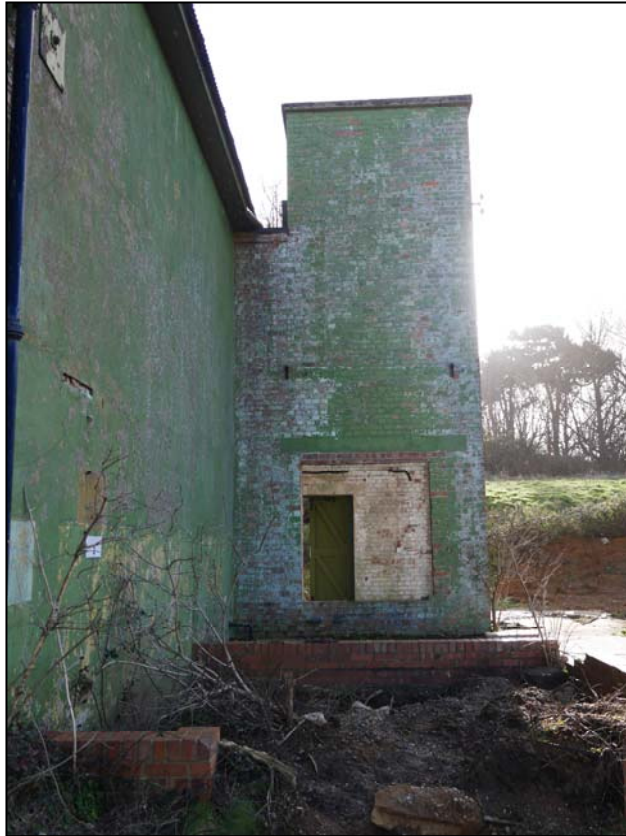
Plate 31. View of the cooling tower, camera facing southeast
