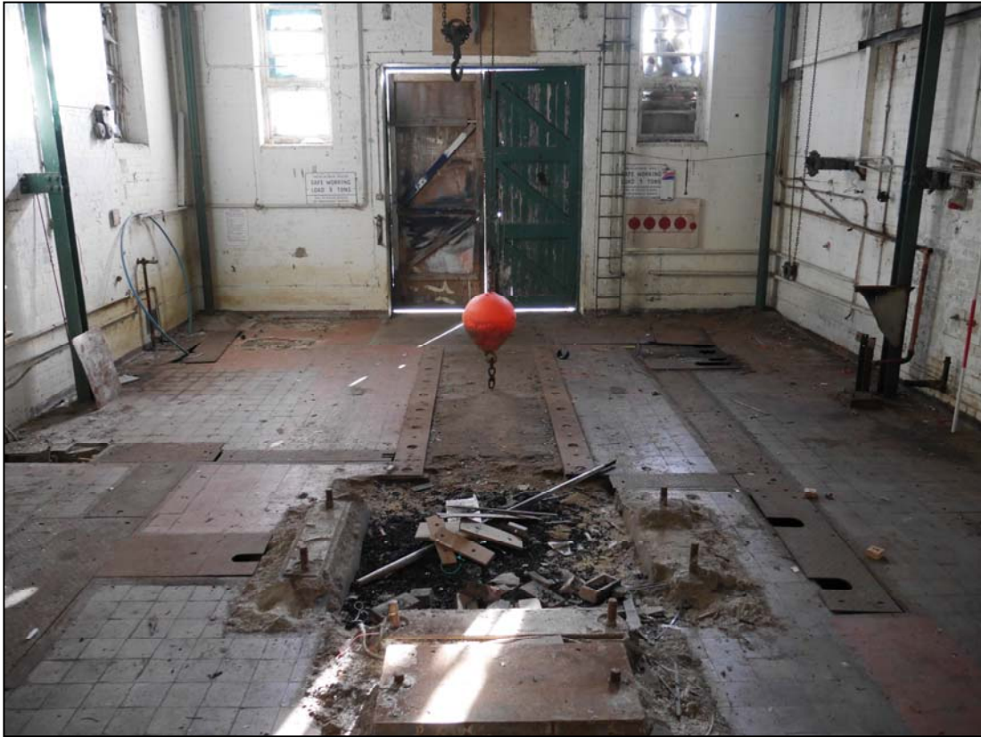
Plate 51. Engine bed (distant) and generator mount (foreground), camera facing southwest
