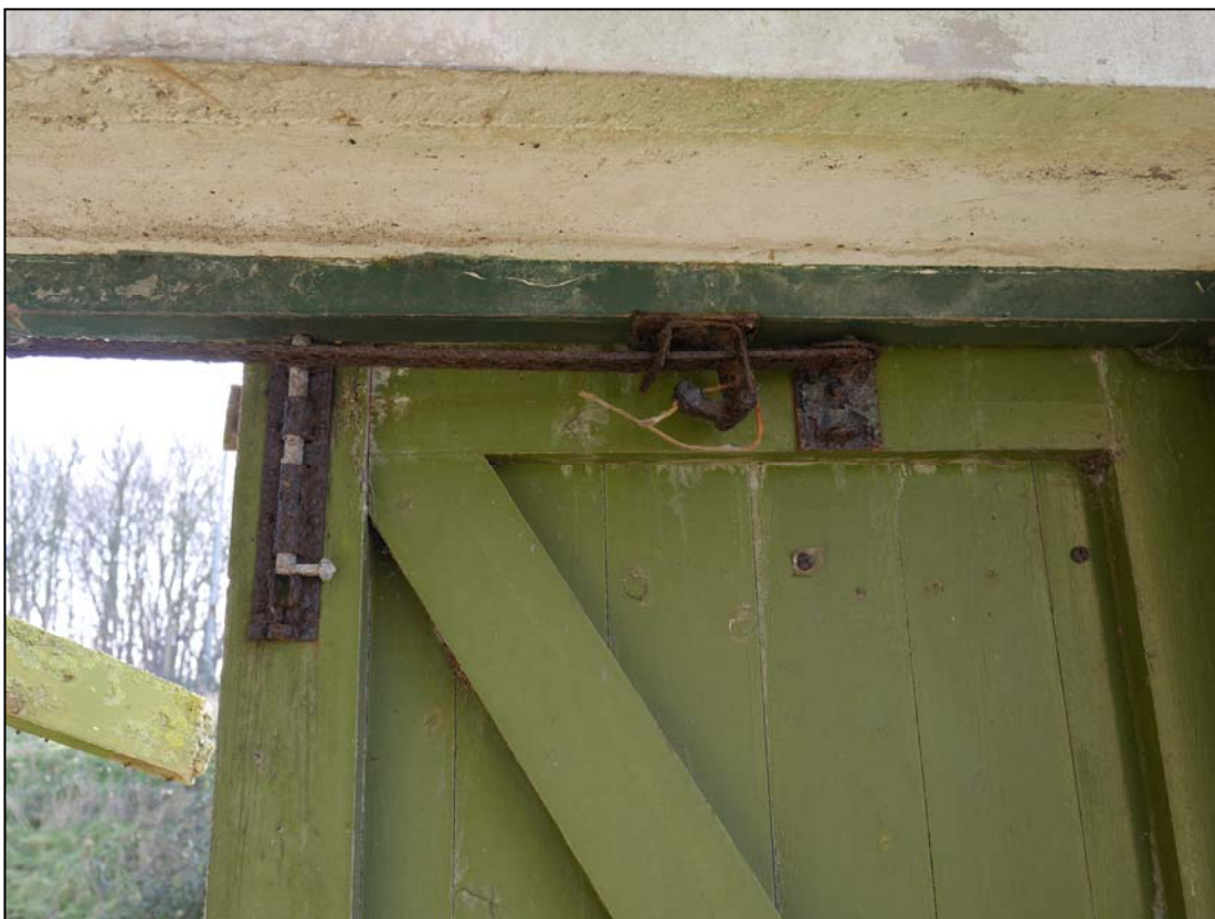
Plate 34. Doors into cooling tower showing detail of closing mechanisms
