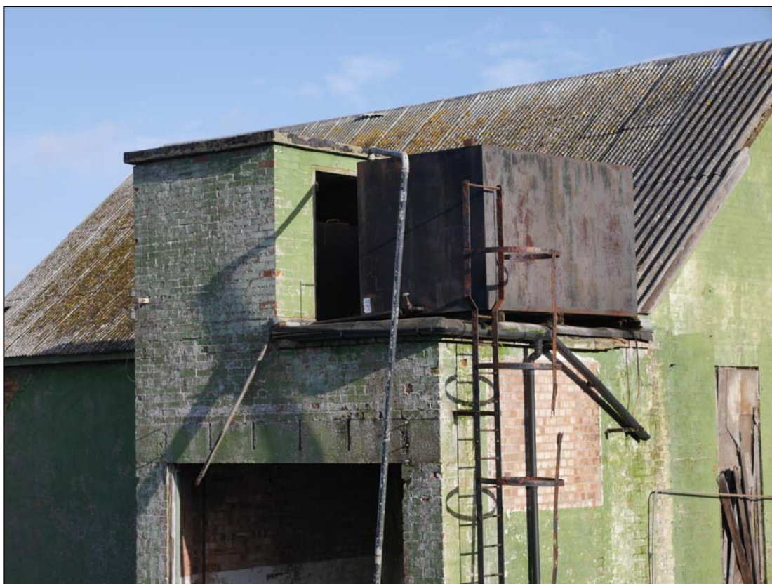
Plate 32. Cooling tower tanks, camera facing north
