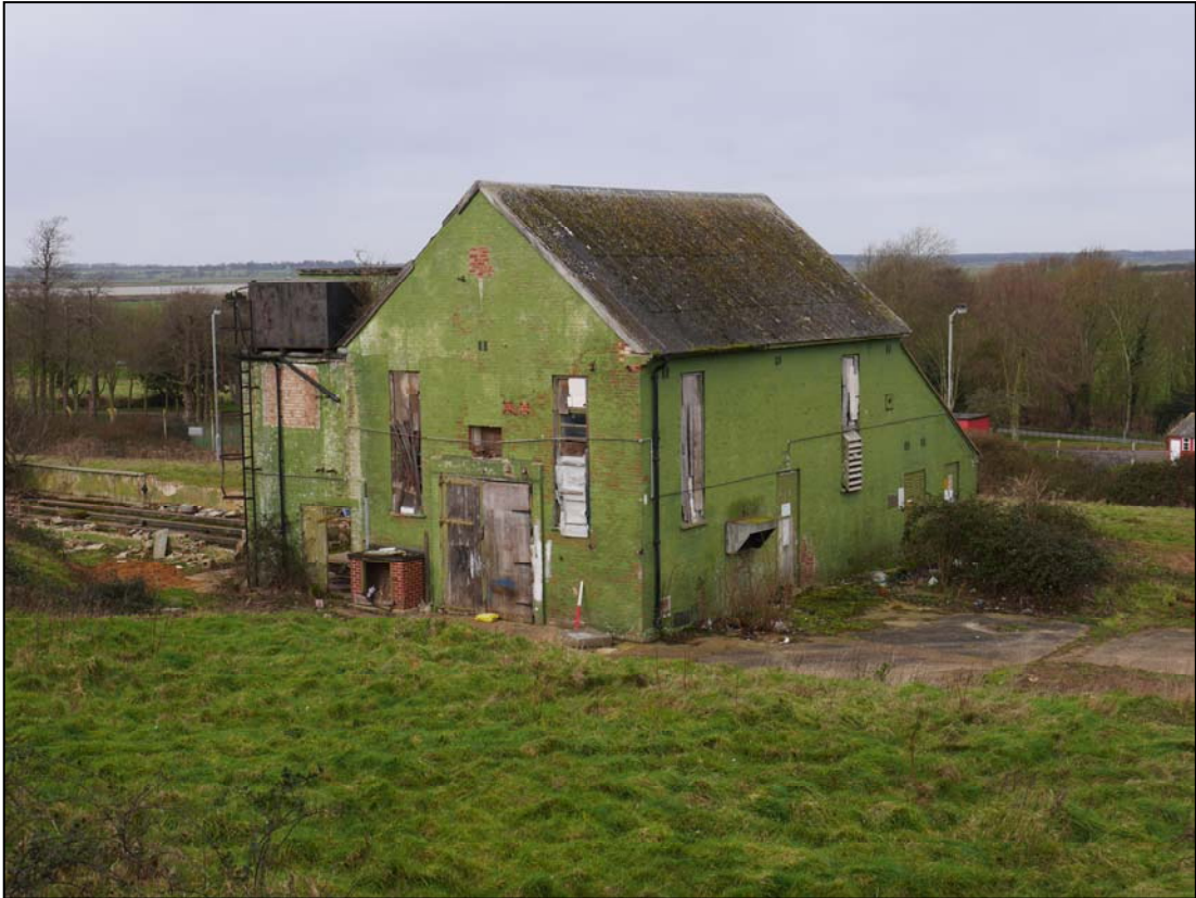
Plate 11. Generator House, camera facing west
