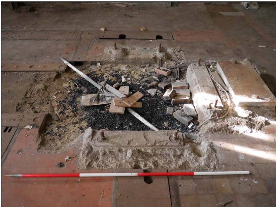
Plate 52. Generator mount with an additional mount for the external exciter to the right, camera facing southwest
