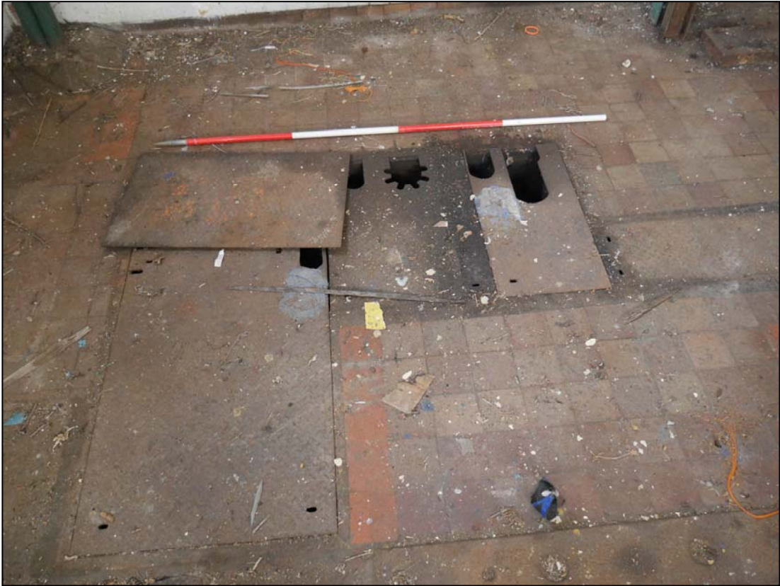
Plate 53. Covered service ducts in southern corner of main room
