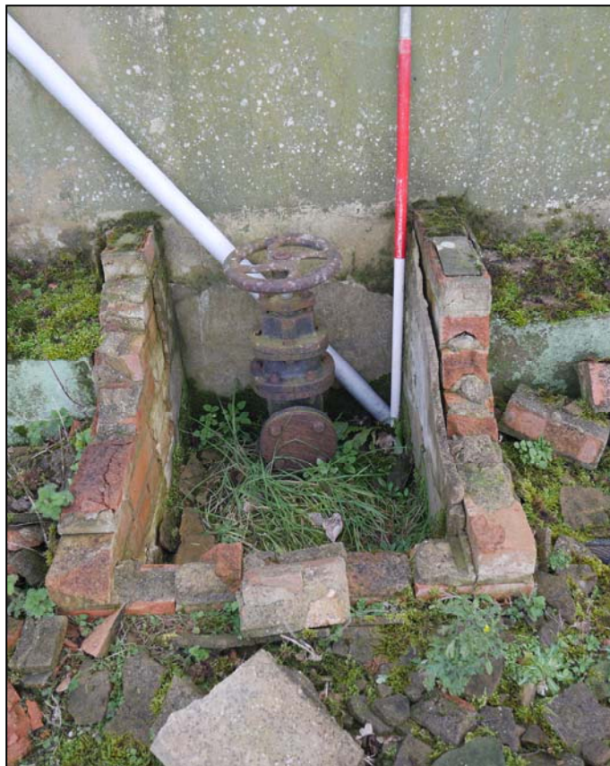
Plate 76. Fuel storage area, external pipe and valve, camera facing southeast
