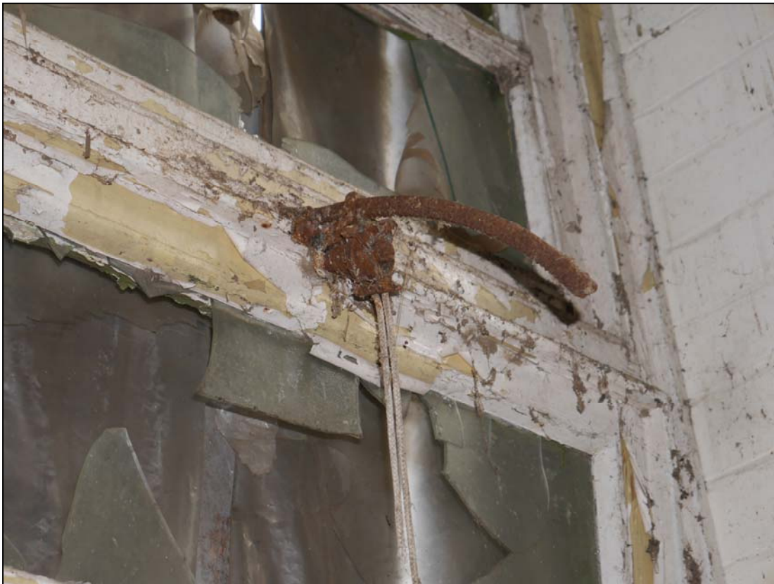
Plate 16. Main room window operating mechanism
