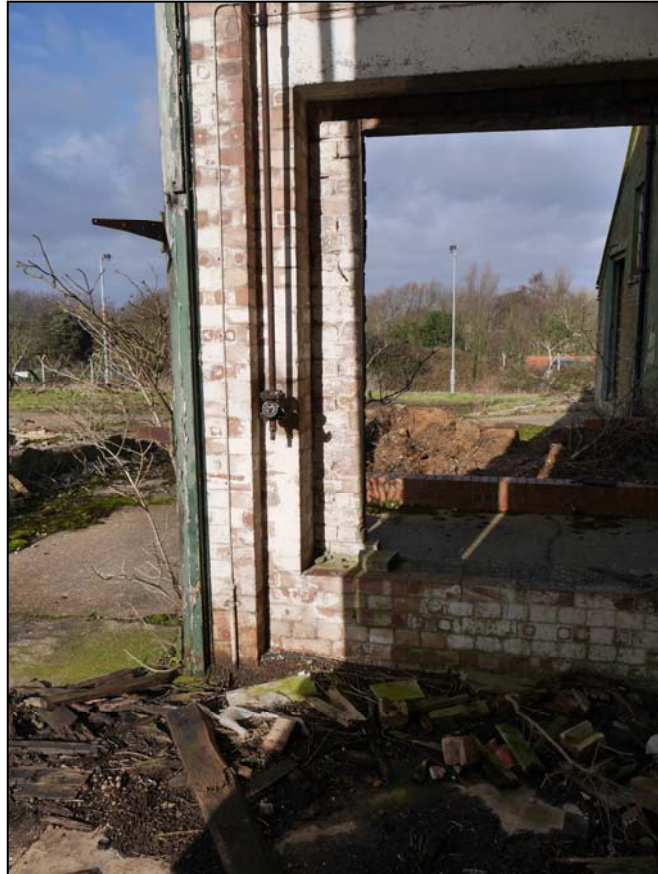
Plate 38. Water pipe with valve in western corner of the cooling tower
