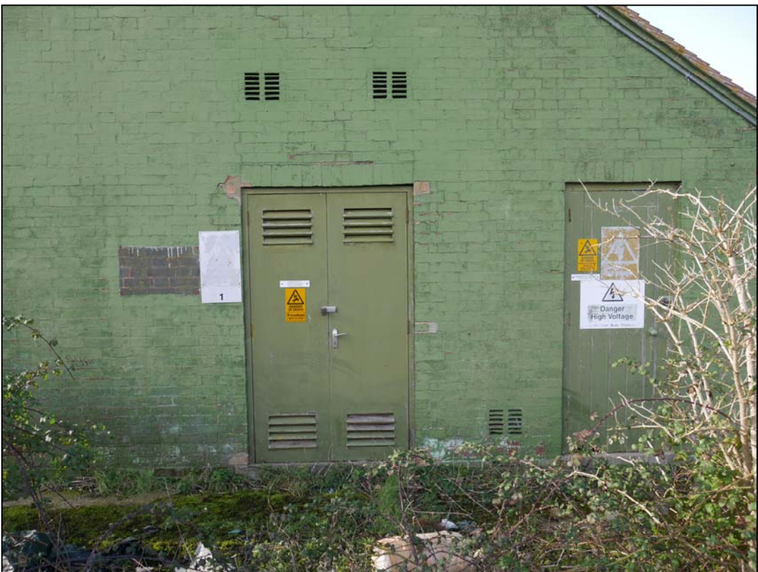
Plate 22. Sub-station access and northeast entrance to store
