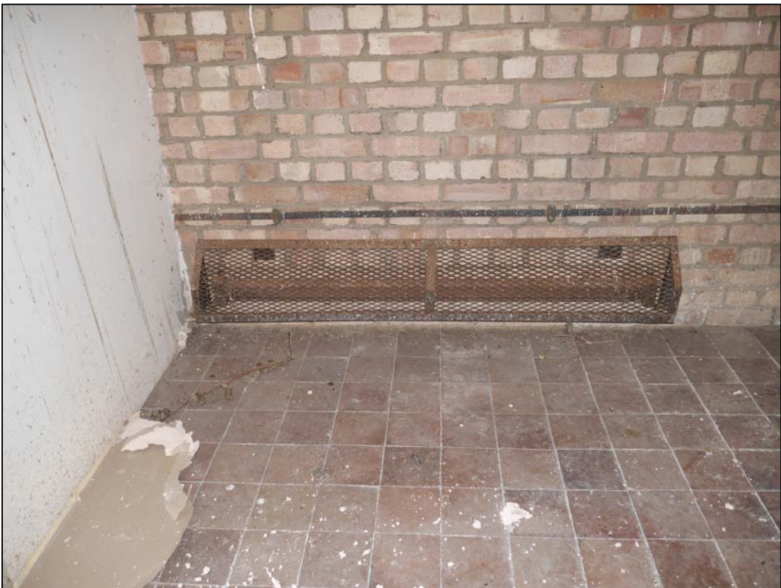
Plate 42. Electrical heater as fixed to inserted wall within store
