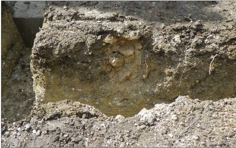
Plate 3. Footing observed in new foundation trenches (facing west)
