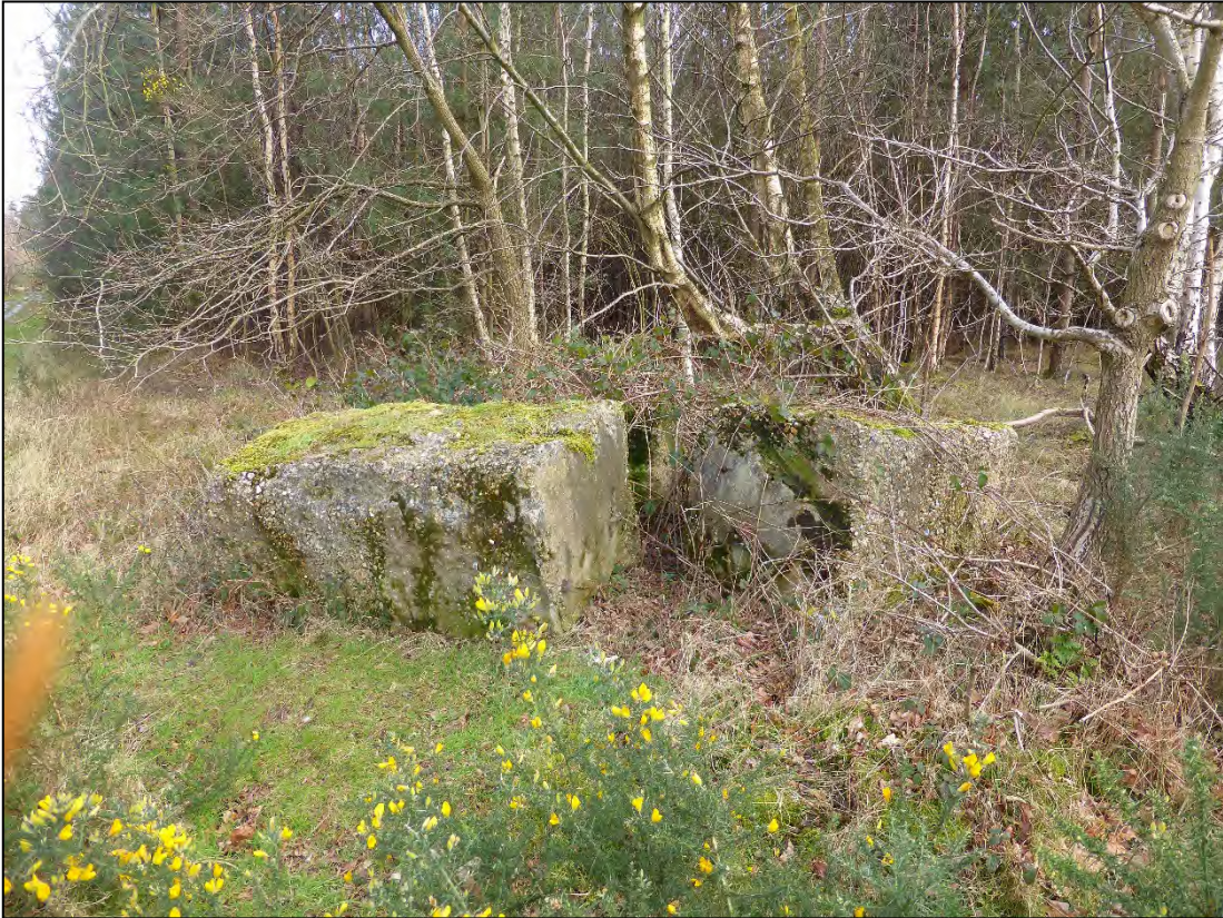
Plate 29. Concrete blocks/supports (050), camera facing southeast
