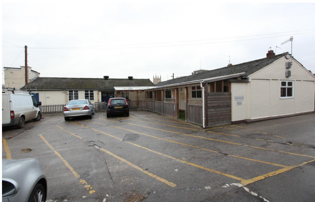
Illus. 2. The two adjoining huts from the south showing the modern veranda adjoining the eastern range (1) on the right and the water tower against the gable of the western range (2) on the left. The outline of a blocked original window is visible in the southern roof gable on the extreme right. The windows of the eastern range are modern PVC replacements but the original Crittall windows survive in the western hut.
