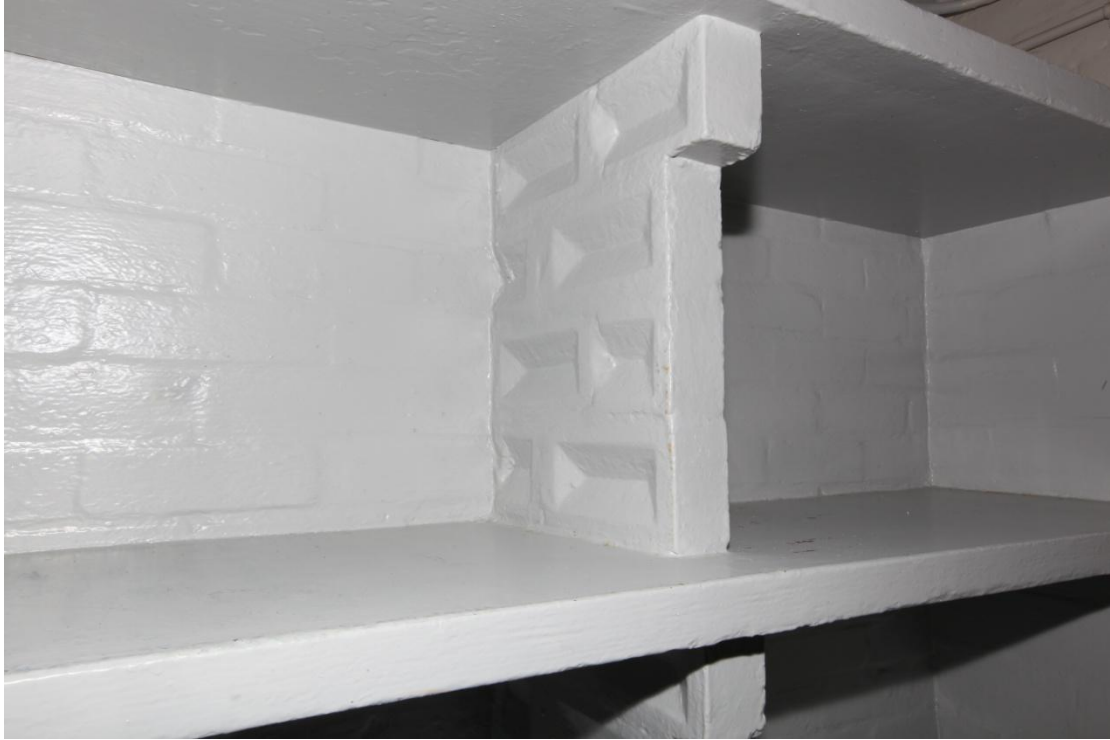
Illus. 15. A detail of the exposed frogs in the brick piers supporting the original shelves of concrete slabs against the western wall of the eastern store room (2d).
