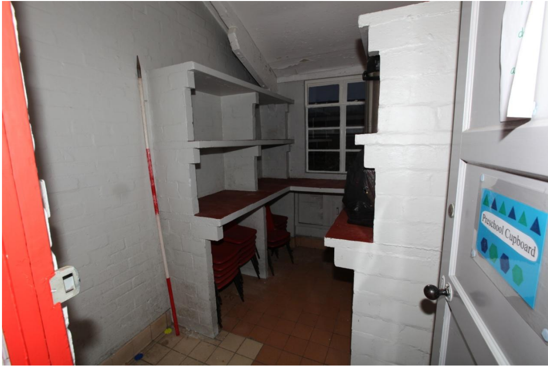
Illus. 13. The interior from the axial passage to the south of the narrow central store room (2c) showing its original door and brick shelving.
