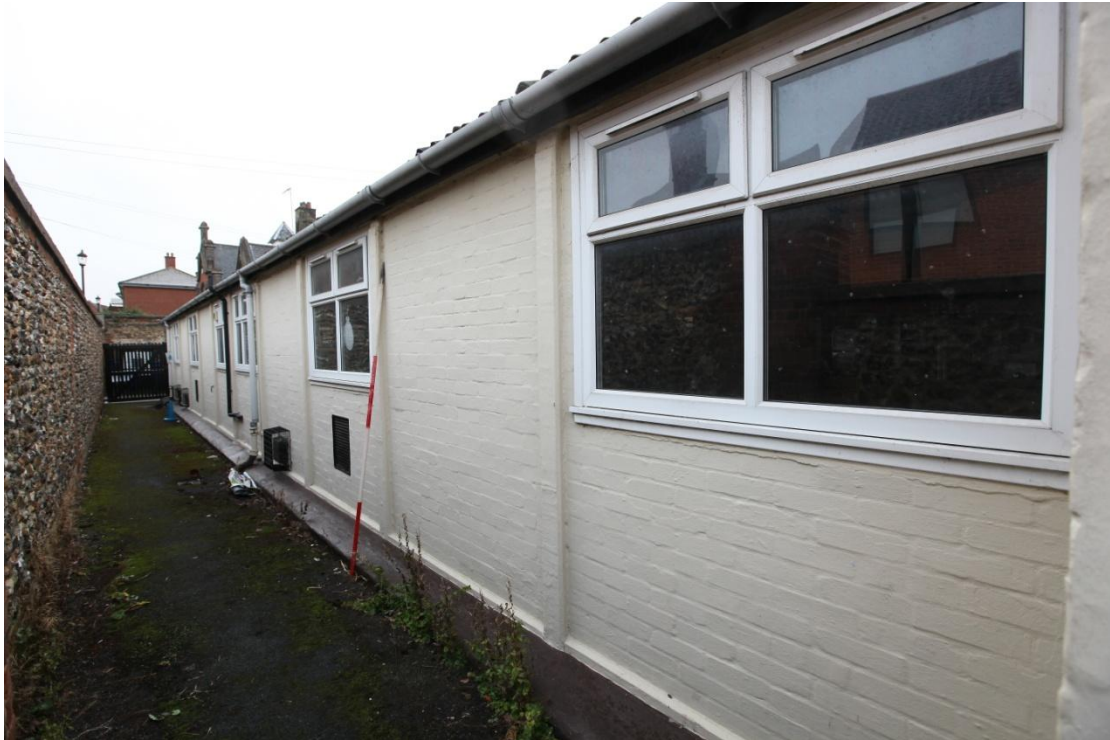
Illus. 3. The eastern exterior of the eastern hut (1) seen from the north with the perimeter wall adjoining Bridewell Lane on the left. The wall fabric of pre-cast concrete piers infilled with brick is original but the PVC windows are recent replacements.
