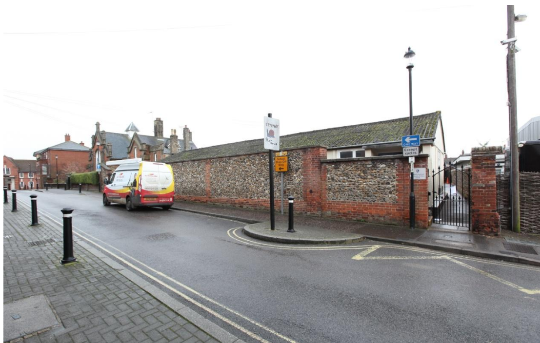
Illus. 1. A general view of the site from Bridewell Lane to the north-east showing the corrugated asbestos roof of the eastern range (1) behind the flint-rubble perimeter wall. The original Mock Gothic school buildings designed by Henry Kendall in 1842 are visible in the rear to the left.
