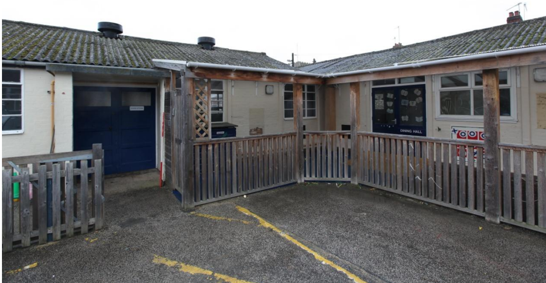
Illus. 6. The southern junction of the two ranges showing the later doors to the dining hall (1a) on the right and the original doors to the kitchen (2a) on the left.
