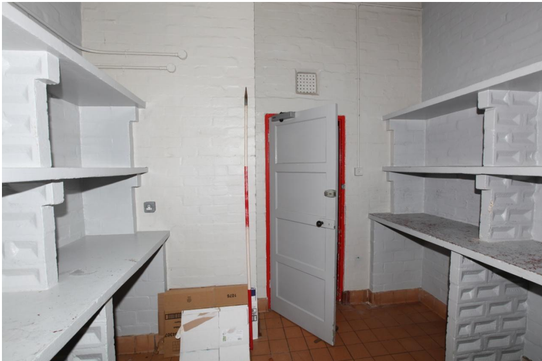
Illus. 14. The eastern store room (2d) from the north showing its original brick shelving and the door to the axial passage (2f).
