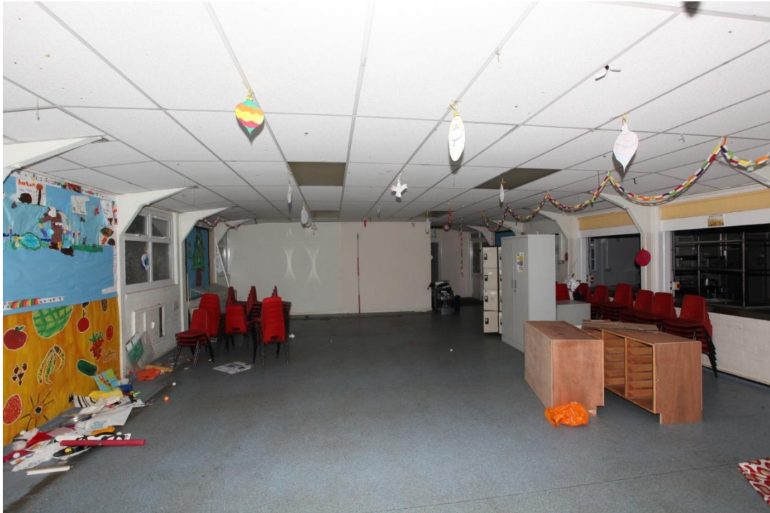
Illus. 9. The dining hall (1a) from the north showing the later ceiling and original concrete bolted knee-braces. The serving hatches adjoining the kitchen (2a) on the right are divided by the original concrete piers.
