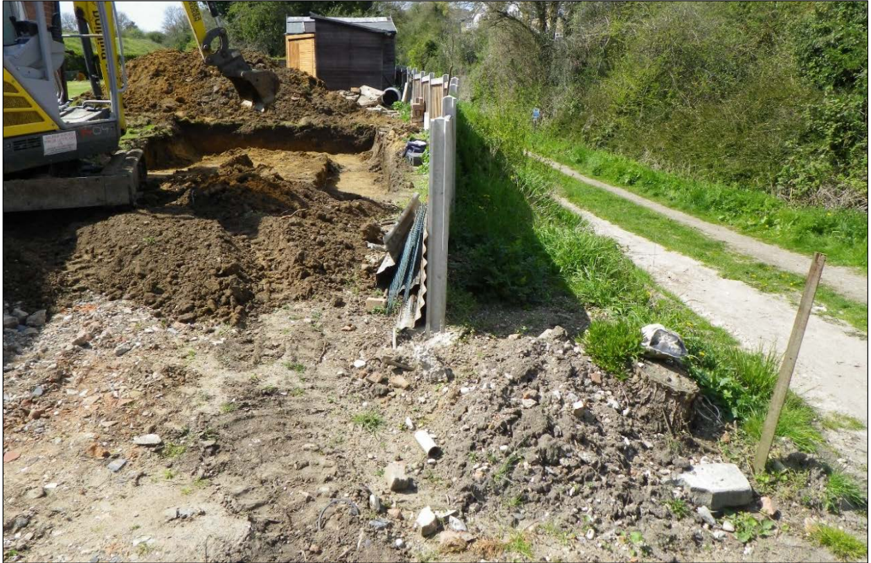
Plate 2. View showing height difference from site to Sheepgate Lane (facing west)
