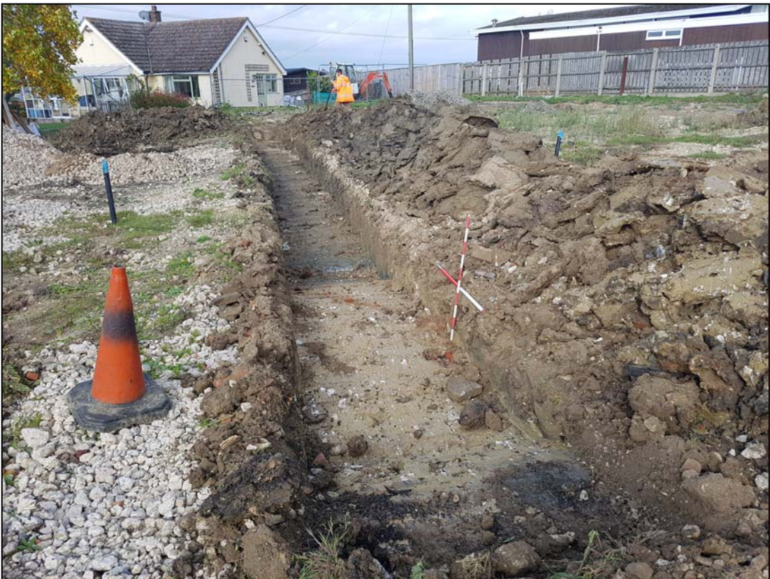
Plate 4. General view of Trench 2 (camera facing northwest)
