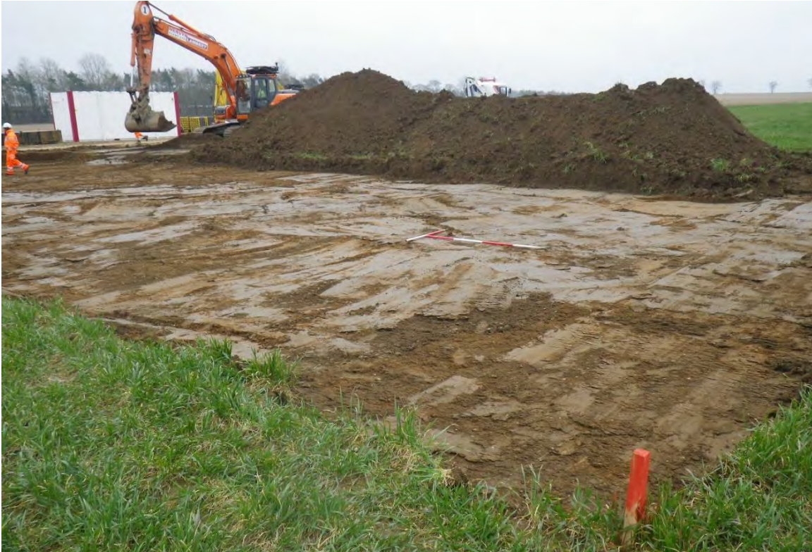
Plate 2. Temporary compound strip, looking south-east, 1x2m and 1x1m scale
