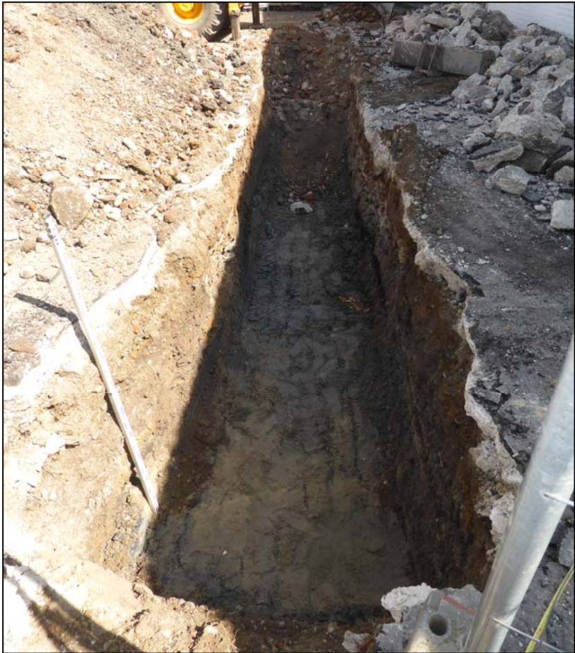
Plate 1. General view of the evaluation trench (camera facing north)
