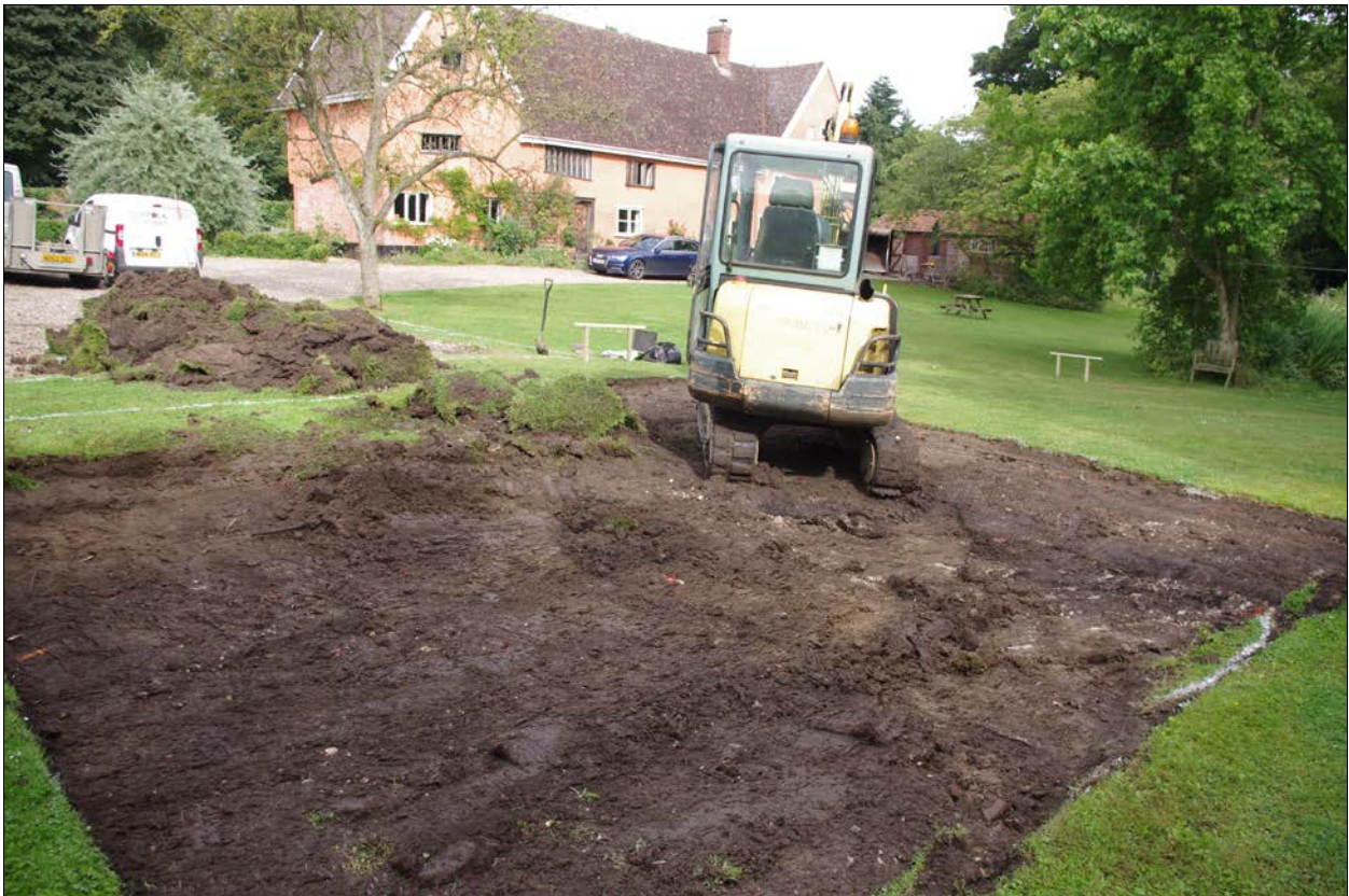
Plate 1. Groundworks in relation to the house
