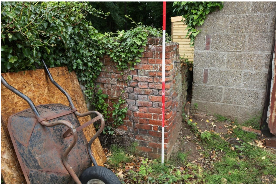
Illus. 4. The south-western external corner of the 19 th century brick shed (6) adjoining the cement-block vehicle shed (5) on the right. The ivy-covered lower courses of a narrow 'porch' flank the original entrance on the left and correspond to the northernmost structure depicted on the 1927 Ordnance Survey –proving the earlier kiln stood on the site of the vehicle shed (5).
