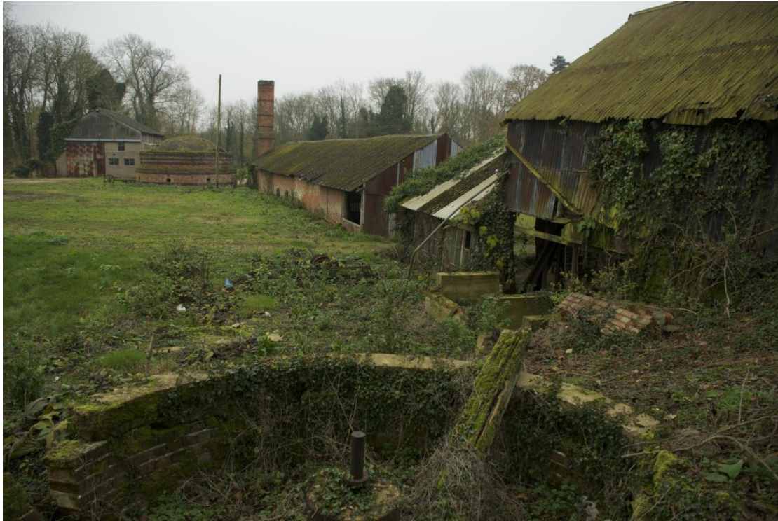
Illus. 17. A 2014 photograph of the site looking east from the pugmill (2) showing the corrugated asbestos roof covering of the drying sheds with the uncovered kiln (1) in the rear. Note the concrete blocks for missing machinery adjoining the extrusion shed (3a) on the right.
