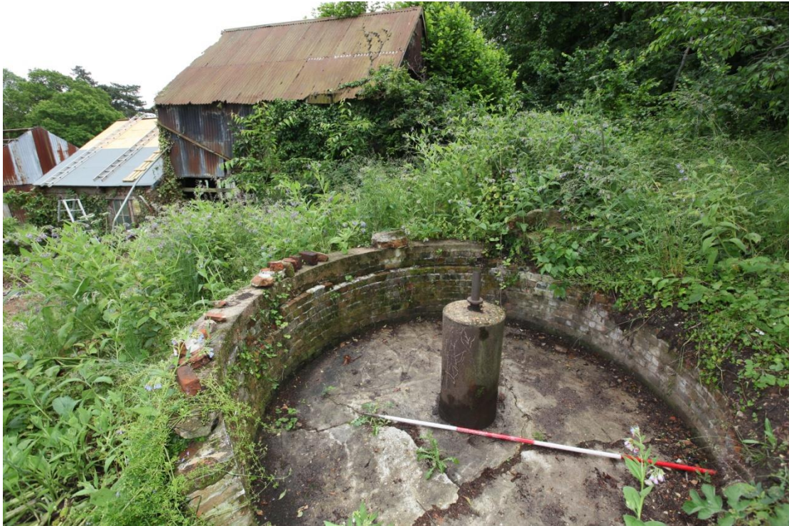
Illus. 13. The circular brick pugmill (2) from the north showing its central iron pivot with the corrugated iron roof and cladding of the two-storied extrusion shed (3a) in the rear. This upper storey of this shed is entered from the higher ground at road level on the right.
