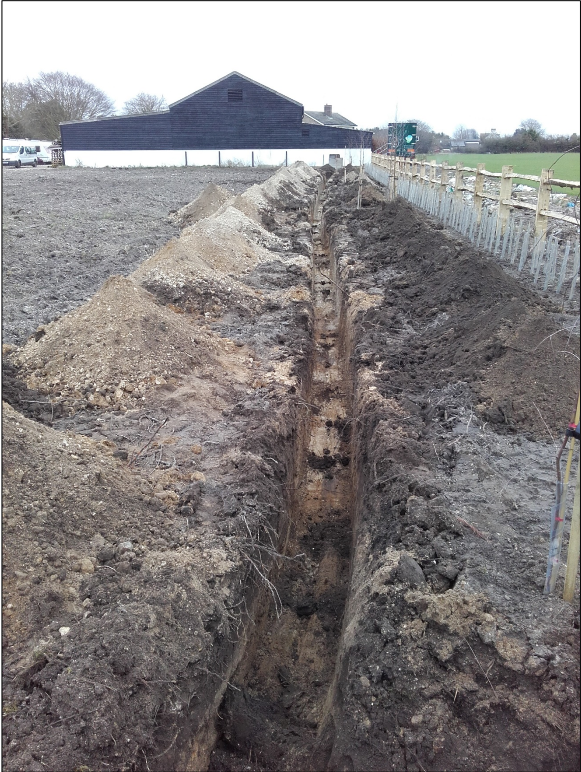
Plate 3. Service trench run, looking west
