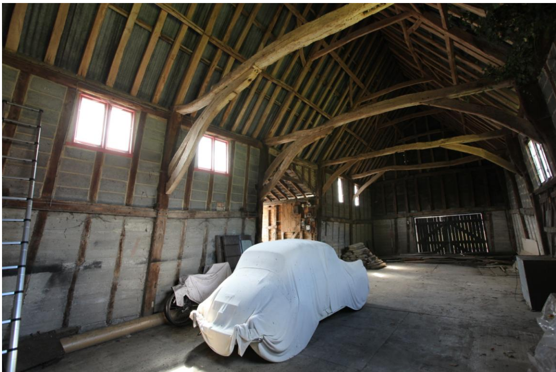
Illus. 6. The interior of the barn (1a) from the north showing the 19th century porch (1b) projecting from the central bay to the left and the 20 th century fenestration. The steeply pitched roof consists of two tiers of butt-purlins and retains almost all its original wind-braces.
