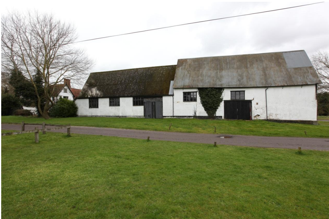
Illus. 4. The threshing barn (1) and former stable (2) from Church Green on the west. Both original roofs are steeply pitched for thatch but are now covered with corrugated asbestos and iron respectively. The stable walls consist of painted 20 th century cement block-work between the original storey posts, and the barn has been rendered in cement. The windows and both sets of double doors are insertions of the 20 th century.
