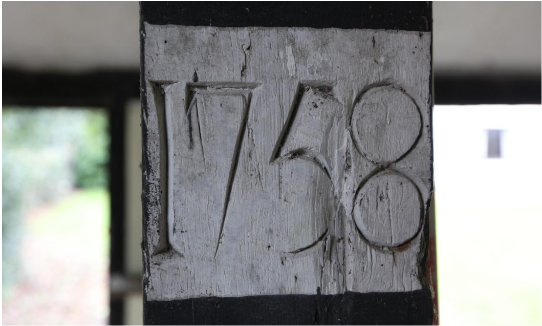
Illus. 15. A detail of the carved date 1758 to the interior of the central post of the former stable's northern section (2b). The carving appears authentic and is consistent with the likely date of construction.
