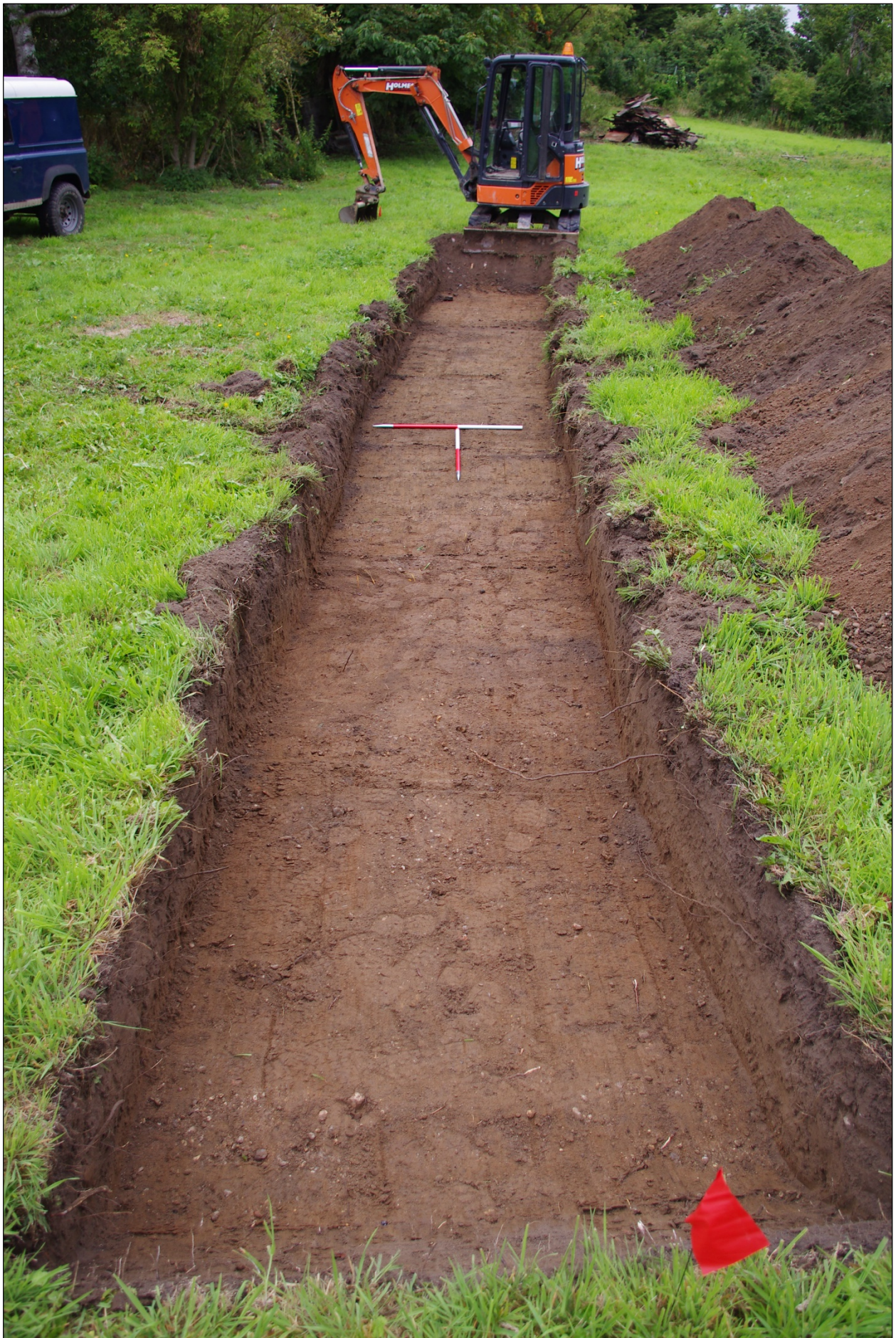
Plate 2. Trench 1, facing east (2 x 1m scales)
