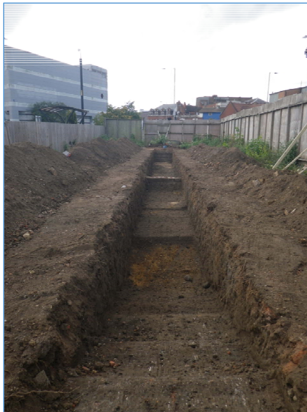
Plate 2. Trench taken from the north
