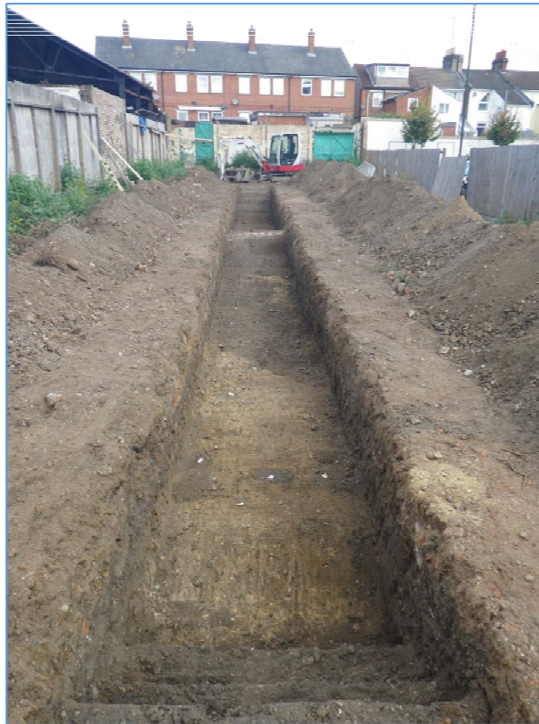
Plate 1. Trench taken from the south
