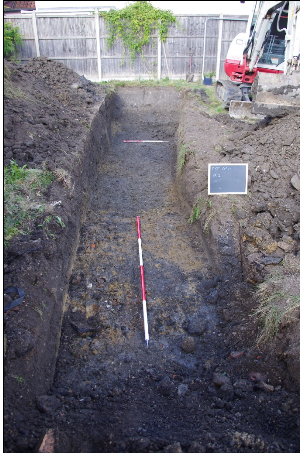
Plate 2. Trench 01, facing northwest
