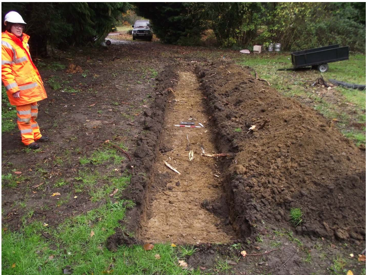
Plate 1. View of Trench 2 looking north-west
