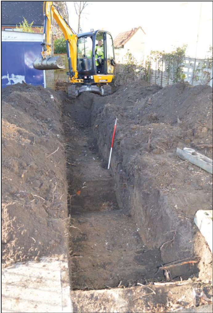
Plate 2. General view of Trench 2 (camera facing west)
