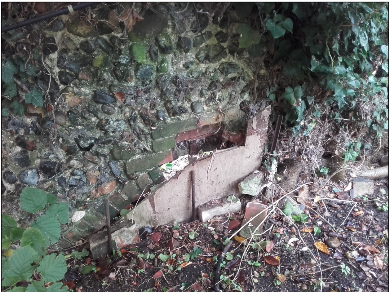
Plate 4. Buried archway in post-medieval wall, looking south
