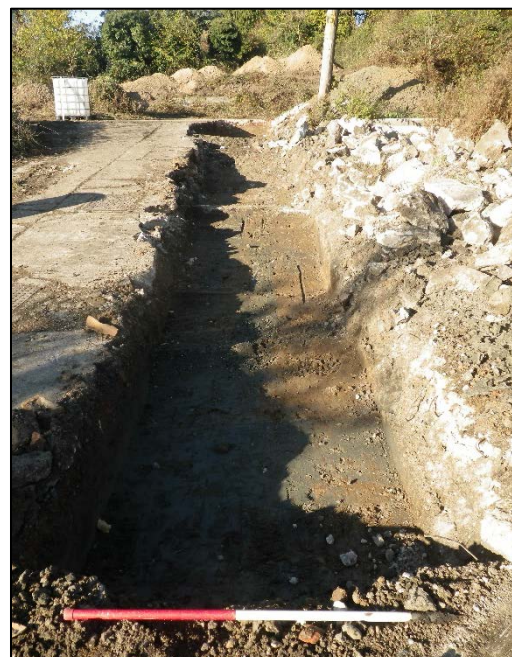
Plate 4. Trench 2, looking NNW
