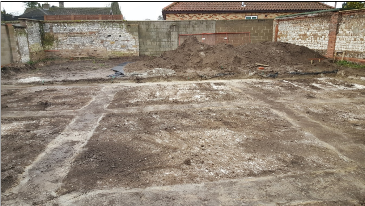
Plate 4. Block 1, facing west across centre after concreting and topsoil strip
