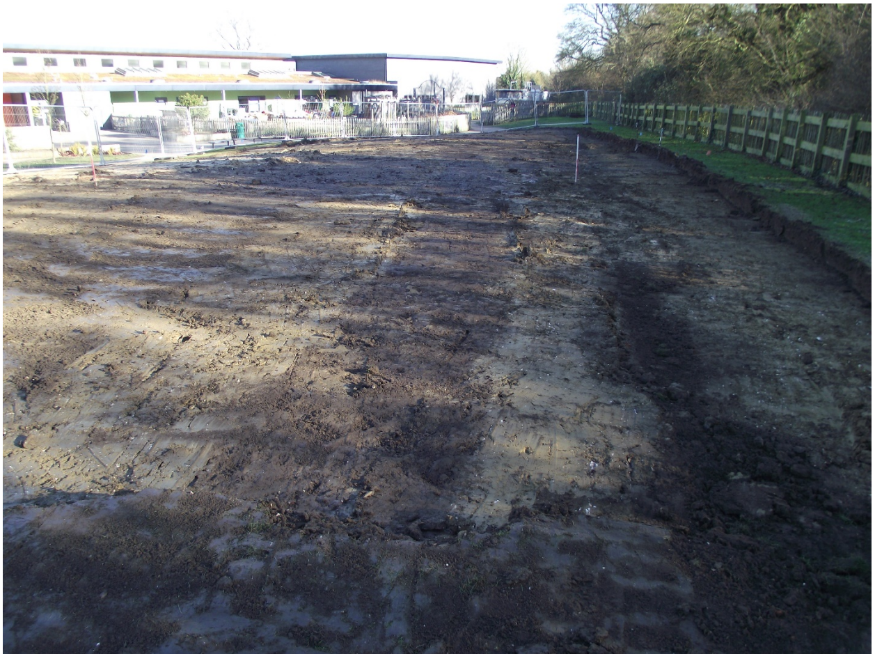
Plate 1. View of site looking east: note deep dumper ruts in the foreground while the least disturbed area is the strip along the right of the frame; the school is situated to the background, note how the ground slopes to the left due to landscaping the level down to the paved playground area to the north.
