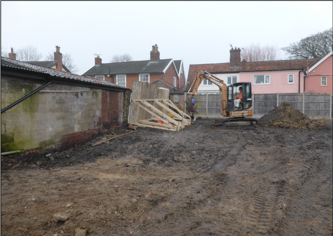
Plate 1. General view of the building footprint, camera facing northwest
