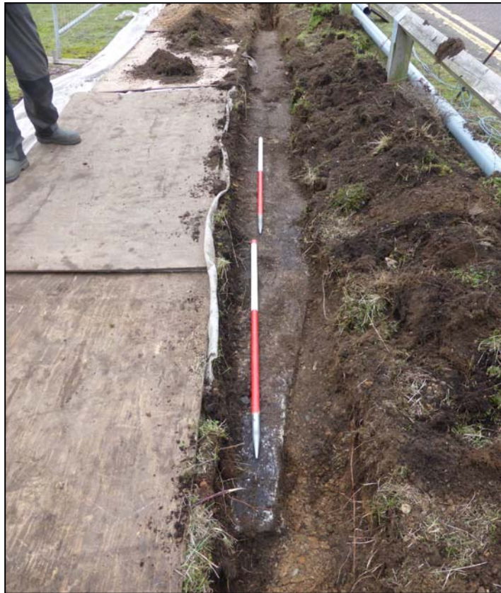
Plate 33. Item 12, exposed section of concrete roadway (camera facing SW)
