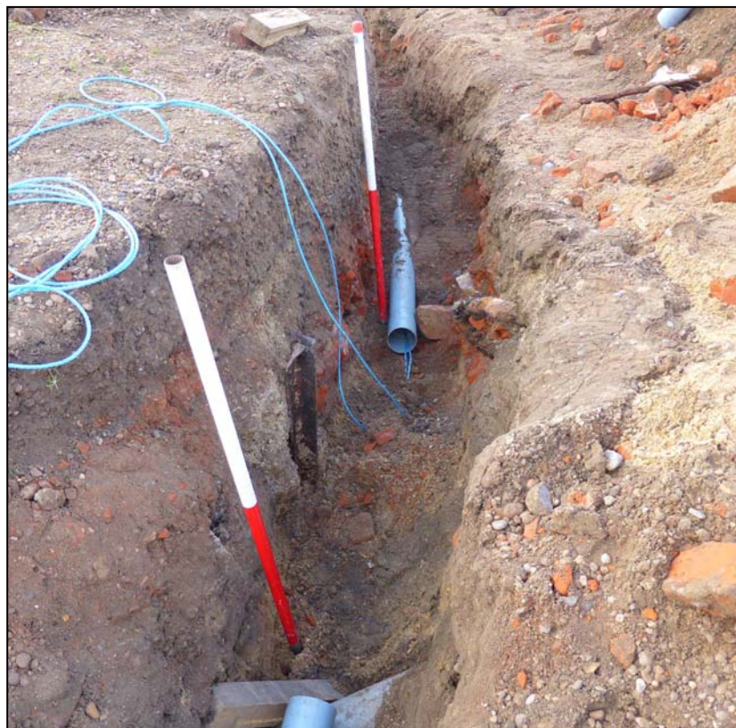
Plate 6. Item 4, with Item 3 beyond (camera facing W)
