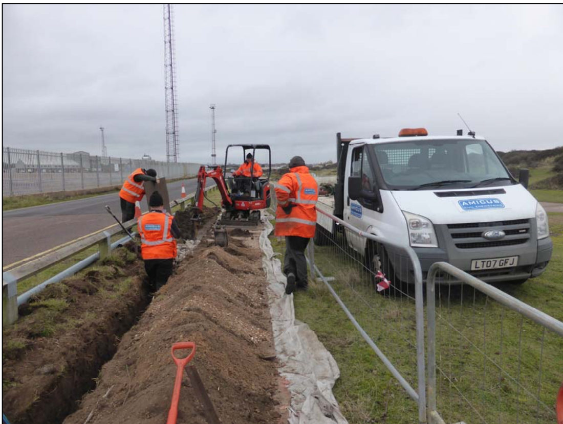
Plate 36. Work underway (camera facing NE)
