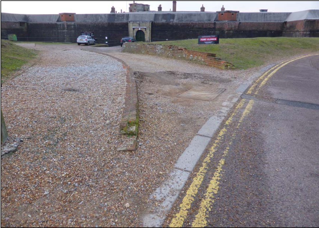
Plate 1. General view of the start point of the service duct showing the fort entrance chicane and the existing manhole, with its cover in place (camera facing SW)
