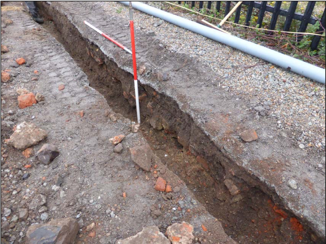
Plate 12. Item 9, after breaking out (camera facing E)
