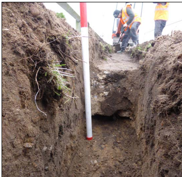
Plate 34. Item 12, cross section of concrete roadway (camera facing NE)
