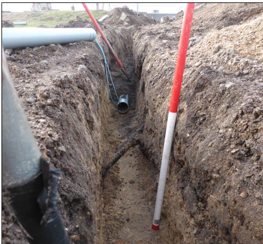
Plate 8. Item 5 (electric cable) running across the excavated trench (camera facing SW)
