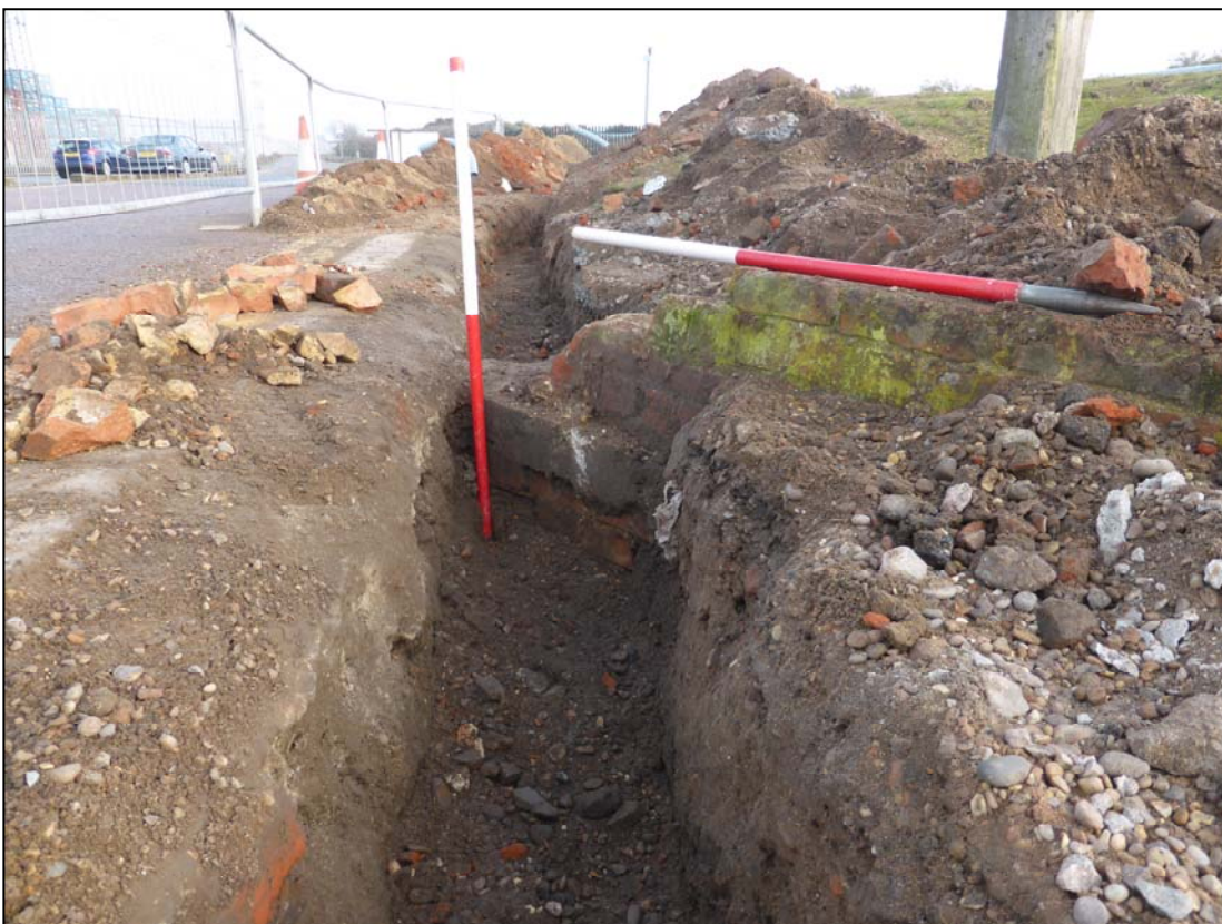
Plate 2. End of chicane wall (Item 1) exposed by excavated trench (camera facing NE)
