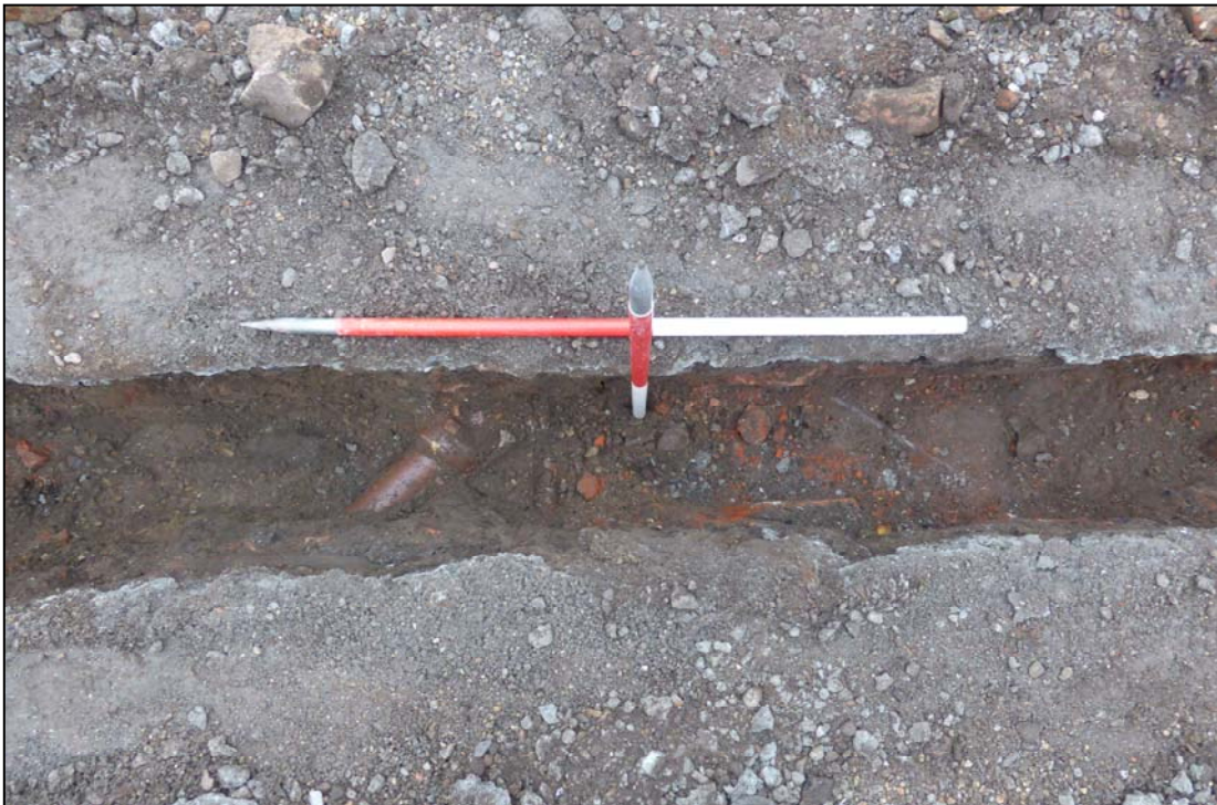
Plate 10. Items 7 (salt-glazed pipe) and 8 (steel pipe) visible on base of trench
