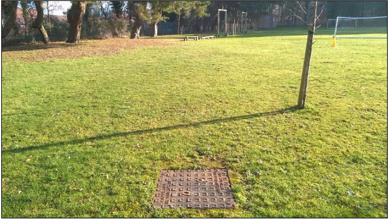
Inspection chamber and proposed development site, facing east.
