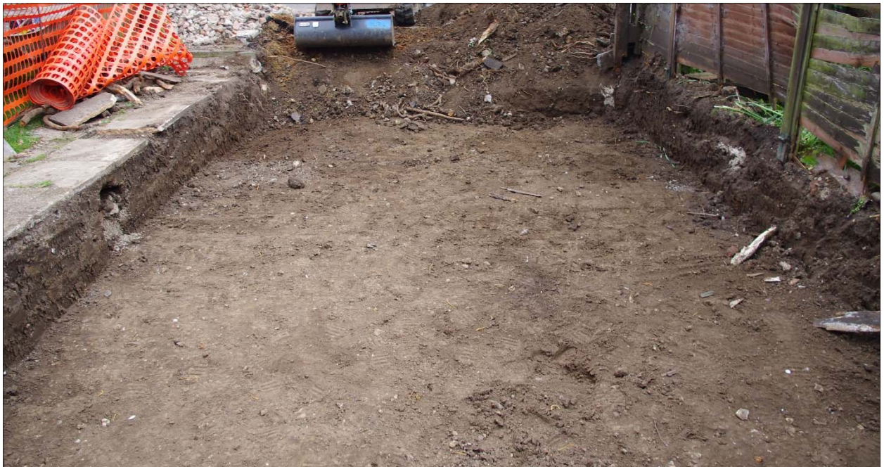
Plate 1. Garage strip (facing east-south-east)
