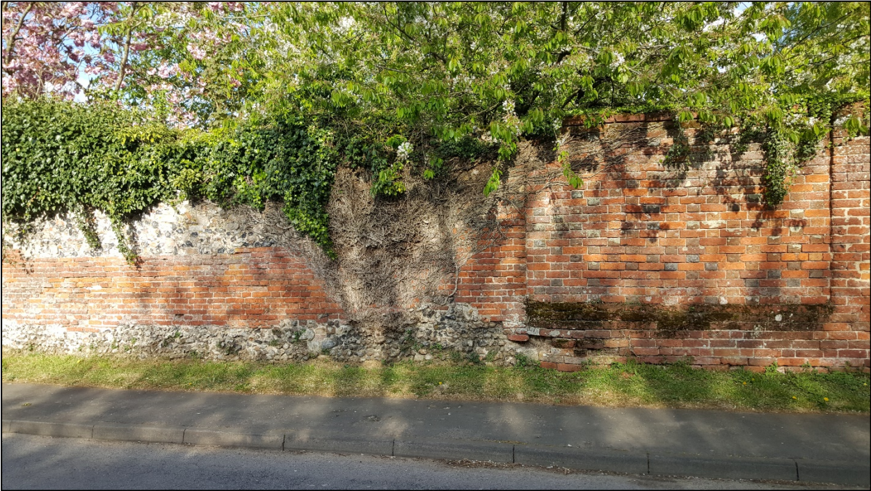
Plate 7. Exterior of the curtilage wall, facing east, at point where medieval flintwork terminates
