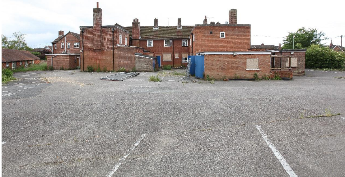
Illus. 3. The site from the car park to the north showing the two projecting rear wings with the Police House and single-storied 19 th century sheds on the left. In their present forms both square-ended gables are later additions and contrast with the elegant hips of their predecessors.
