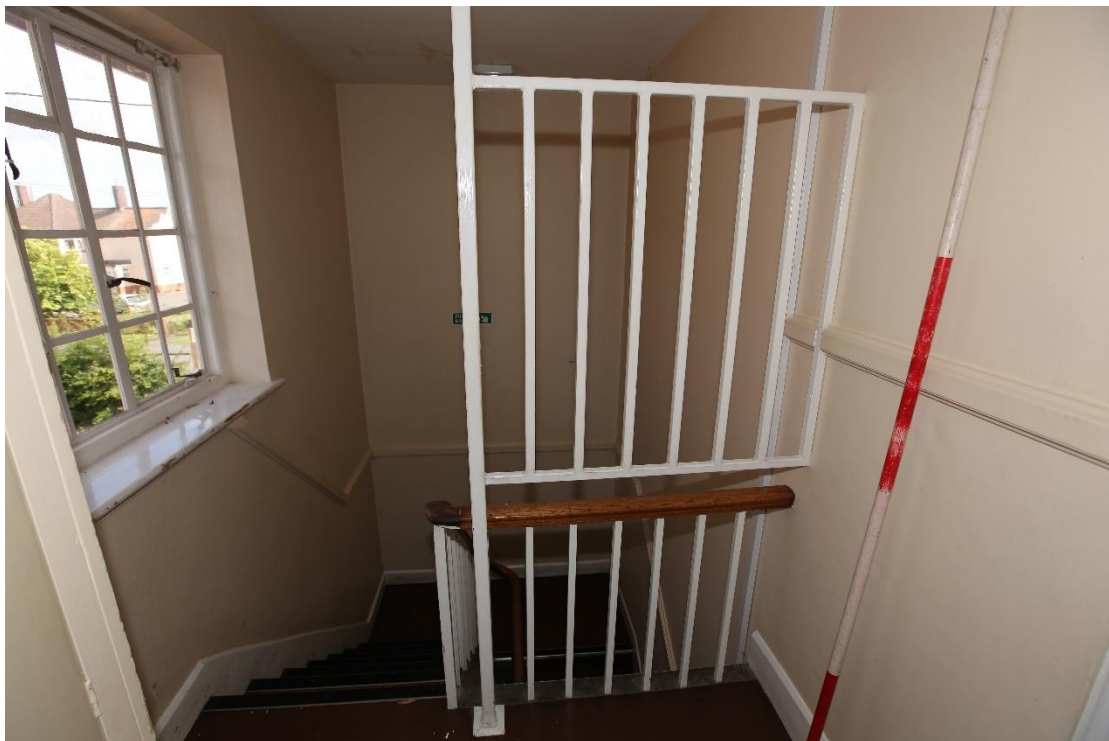
Illus. 14. The first-floor landing of the relatively plain staircase (18f) at the eastern end of the main building, viewed from the rear (north). The steel bars are later insertions presumably designed to deter jumping. This stair initially linked the communal ground-floor mess and kitchen to the first-floor cadets' cubicles and constables' bedrooms.
