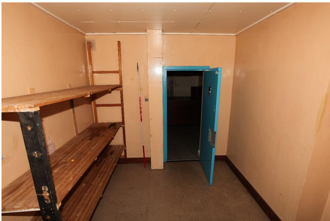
Illus. 10. The juvenile detention cell (19g) from the west showing the steel door opening onto the charge room (20g). This cell is an addition of 1966 but was evidently converted into a storage shed in recent years as the shelving on the left is a modern insertion.
