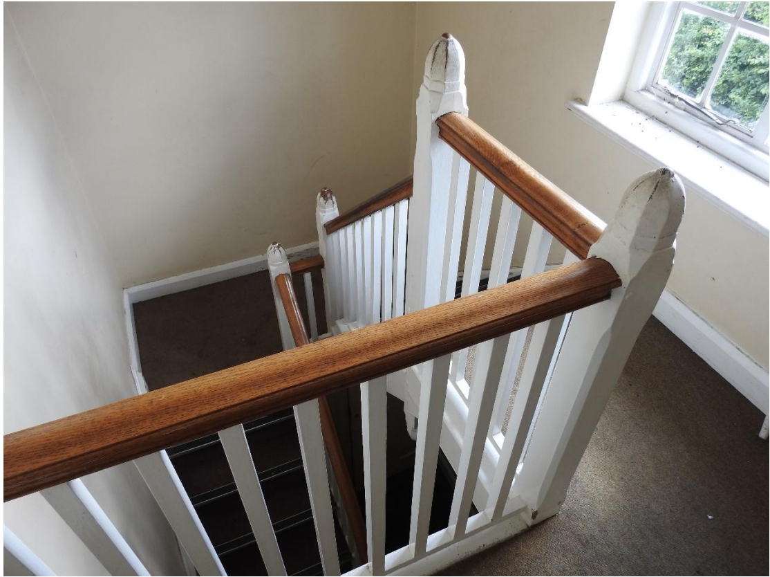
Illus. 7. The original main staircase at the western end of the building as seen from the first-floor landing (12f) to the north. The finials of the newel posts bear a striking and surely deliberate resemblance to contemporary police helmets.
