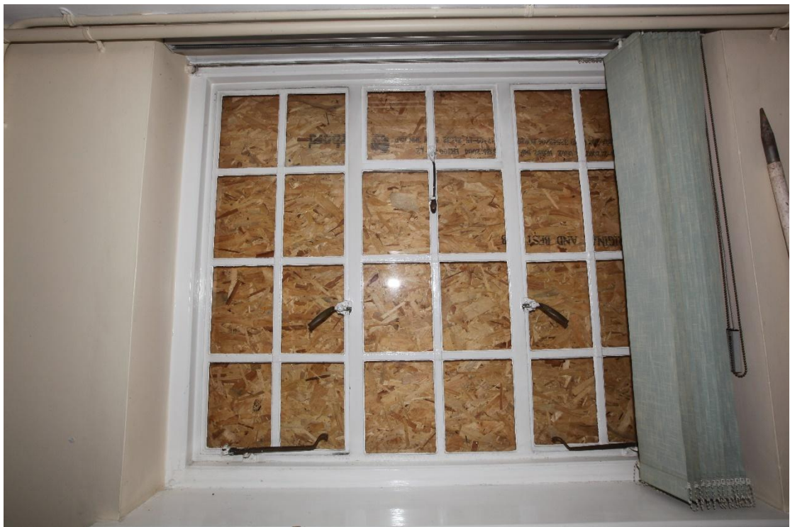
Illus. 8. An original metal-framed Crittall window, typical of those found throughout the building, with bronze handles, latches and catches. This example is in the eastern internal wall of the former constables' room, which was originally a kitchen (8g).
