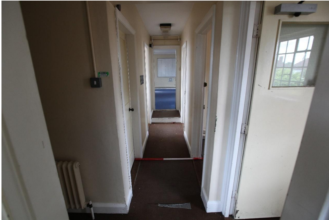
Illus. 15. The axial central first-floor corridor of the eastern wing (20f), seen from south, with the incident room (23g) in the rear and the door to the eastern staircase (18f) on the right. The appearance of this corridor is typical of those elsewhere in the building.
