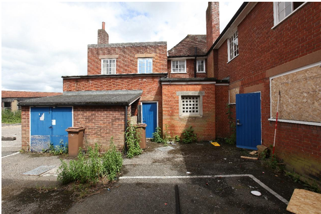
Illus. 4. The eastern rear wing from the yard to the west showing the window of the juvenile detention cell (19g) in the centre and the enclosed exercise yard (E) to the left. The upper storey originally ended at the hipped gable above the juvenile cell and was extended in 1952.
