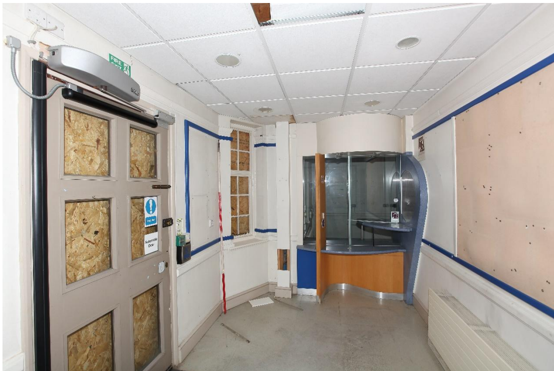
Illus. 6. The interior from the east of the public lobby (15g) showing the reception desk with the central main entrance on the left and a notice board on the right.
