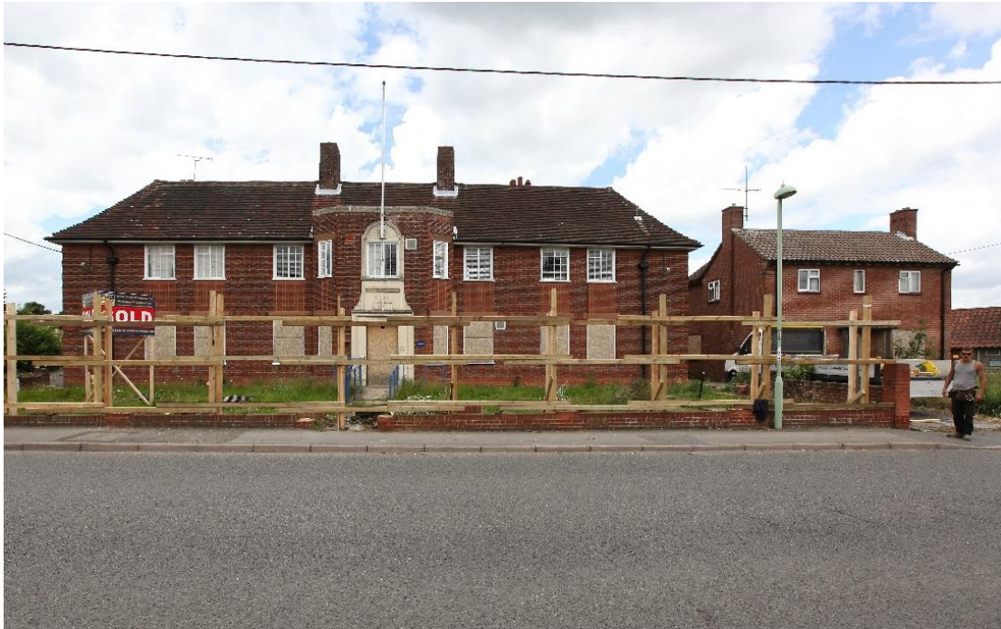
Illus. 1. The distinctive facade of the 1930s Police Station seen from Grundisburgh Road to the south with the 1960s Police House to the right. (The perimeter fence is a modern addition in course of construction at the time of inspection.)
