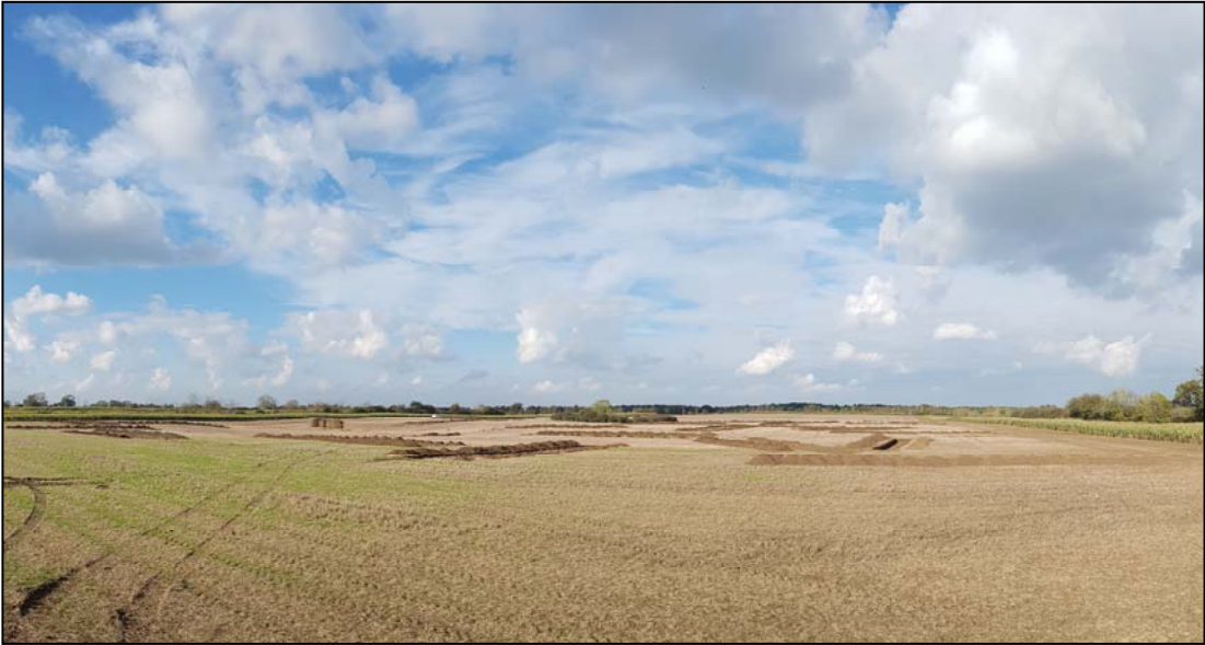
Plate 1. General view of the reservoir site (camera facing northwest)
