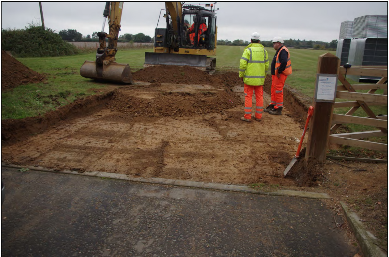
Plate 1: General shot during excavation of the access road, looking west
