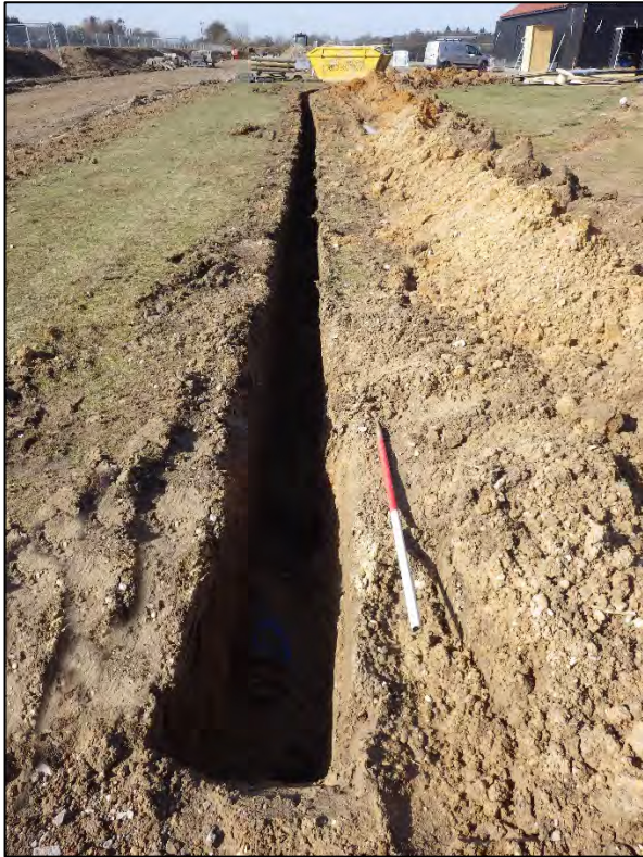
Plate 3: General shot of the drainage trench, looking west, 1m scale
